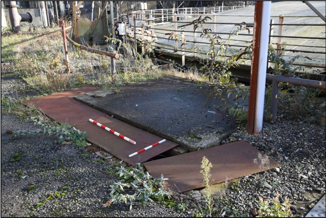
Tank or dry well at the north-west side of Gasholder 1 Fig 27
