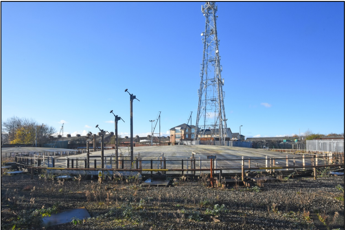
General view of Gasholder 4, looking south-west Fig 38
