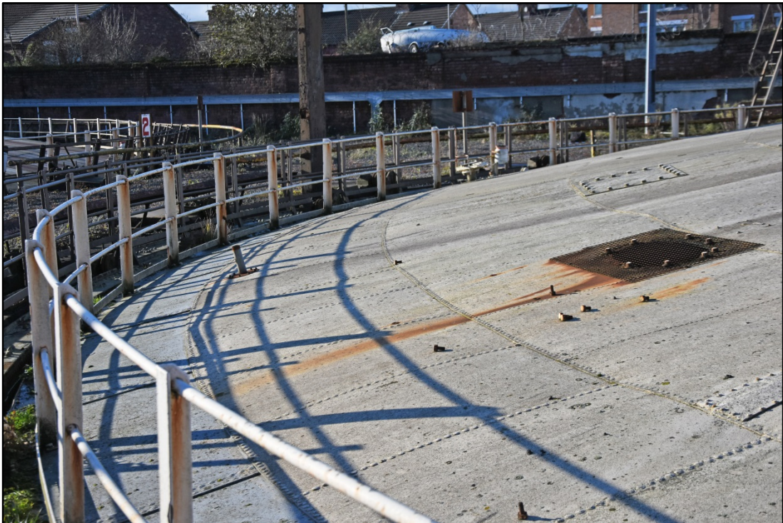
The gasholder crown with manholes Fig 44
