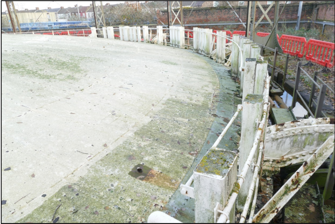
The concrete filled 'balancing boxes' of Gasholder 1 Fig 23
