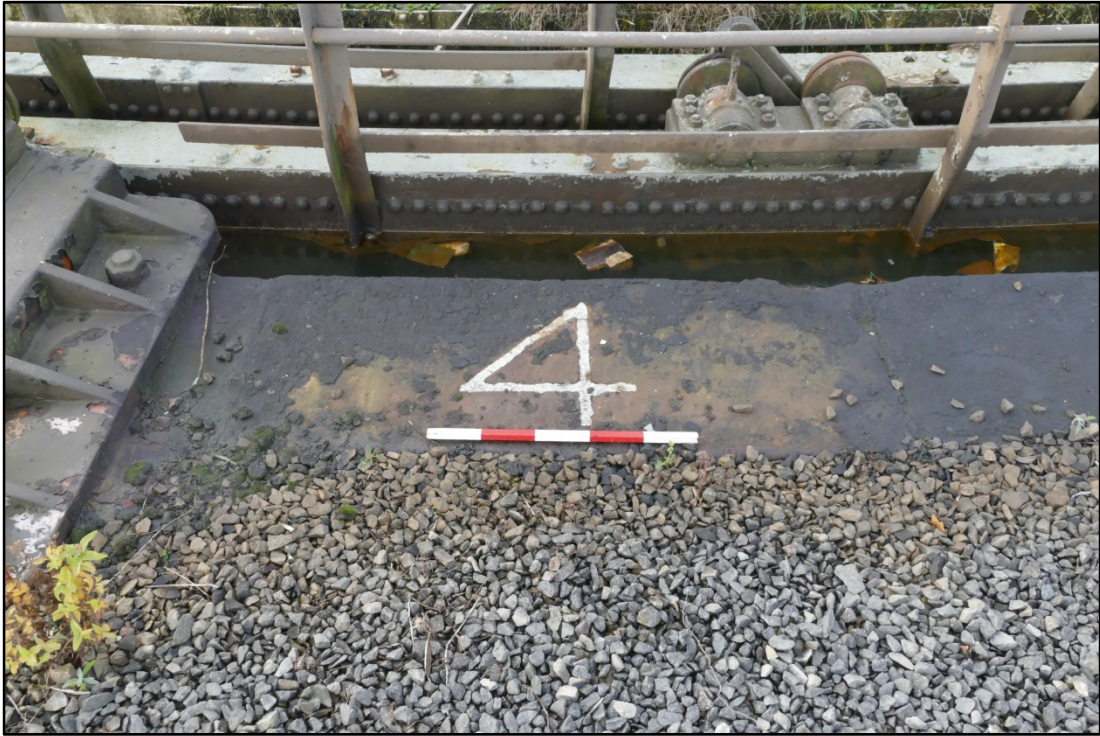
Gasholder designation '4' in the masonry top curb Fig 43
