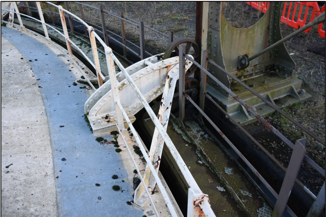
Example of the outer roller carriages Fig 16
