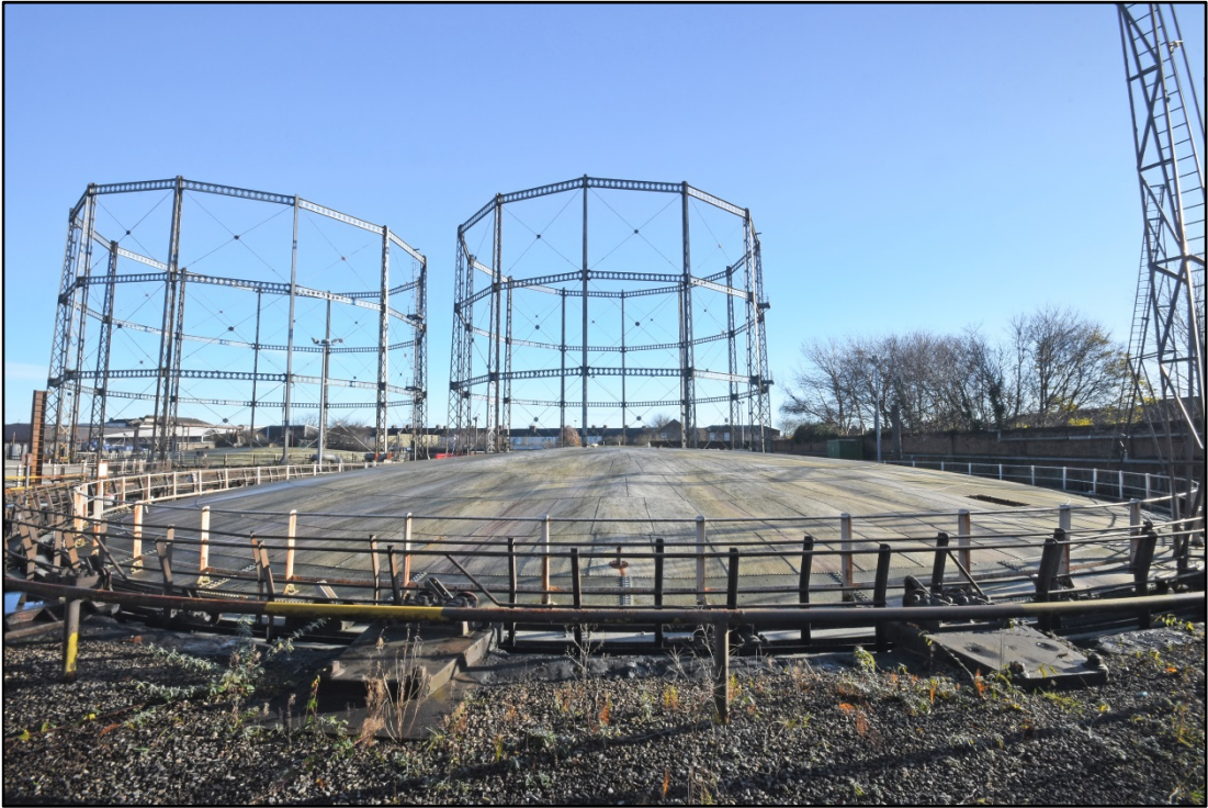
General view of Gasholder 2, looking east Fig 29
