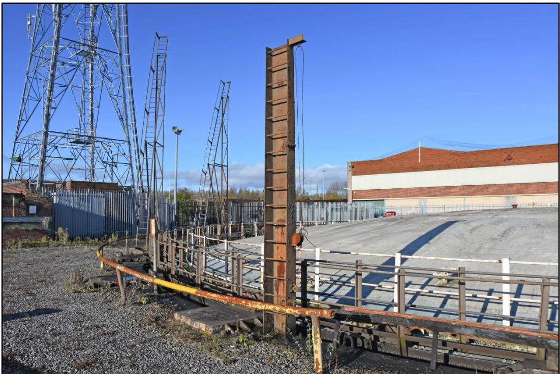
Anti-freeze support and attached cables Fig 42
