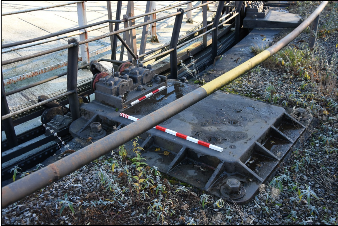
Example of the larger roller carriage footings Fig 33
