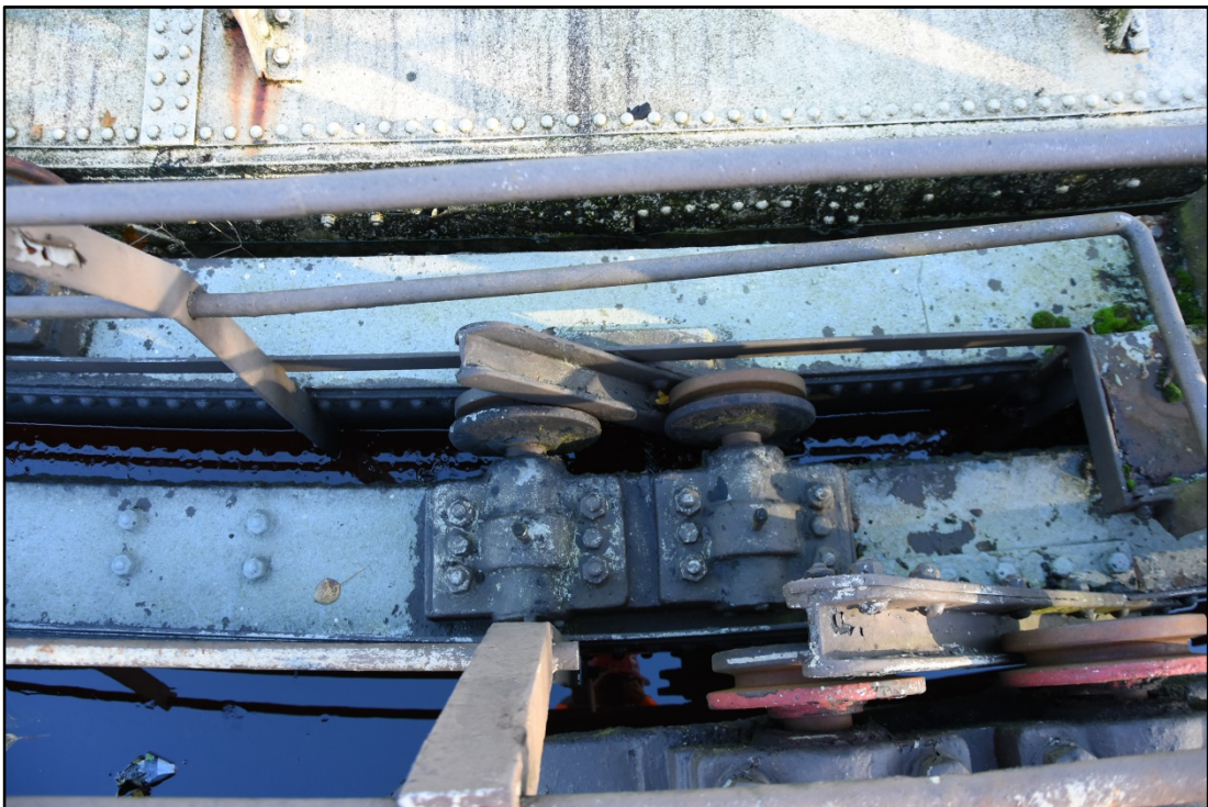
Detail of the tank grips and inner roller carriage Fig 34
