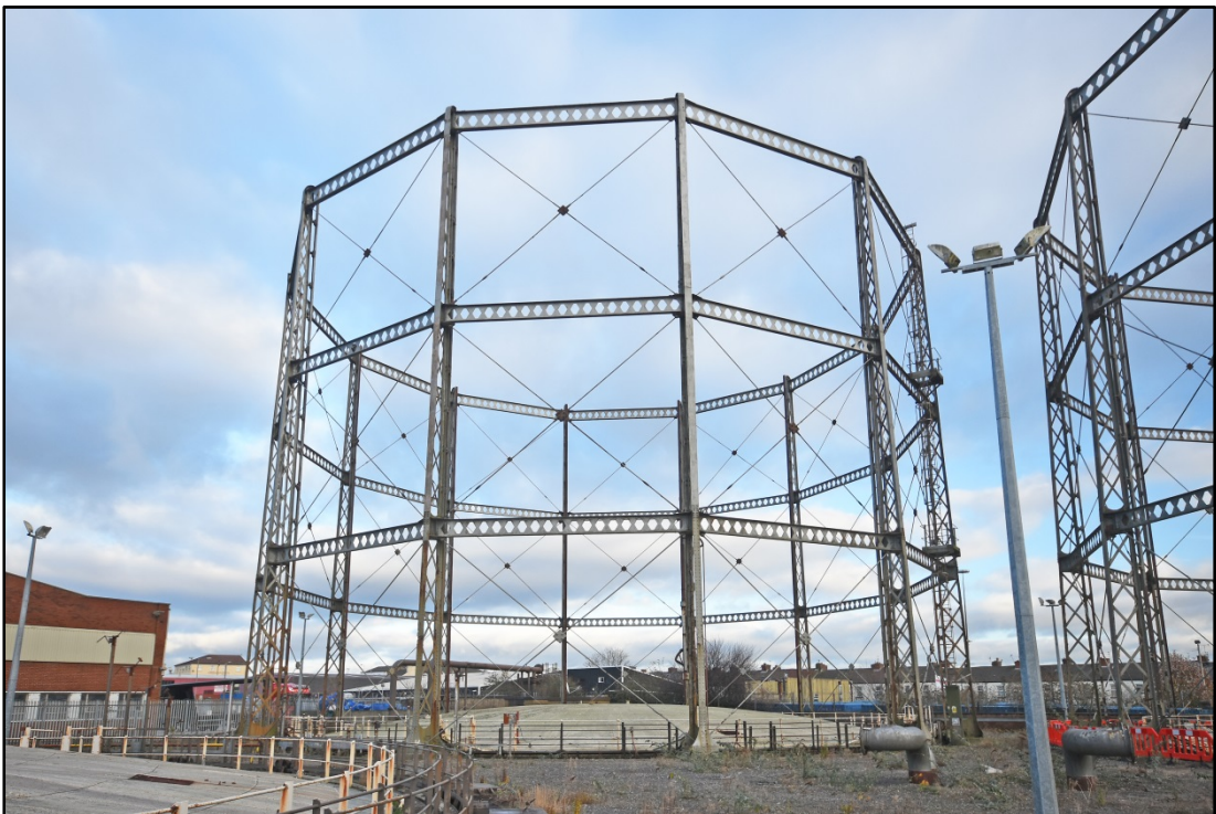
Gas holder 3, looking north-east Fig 12
