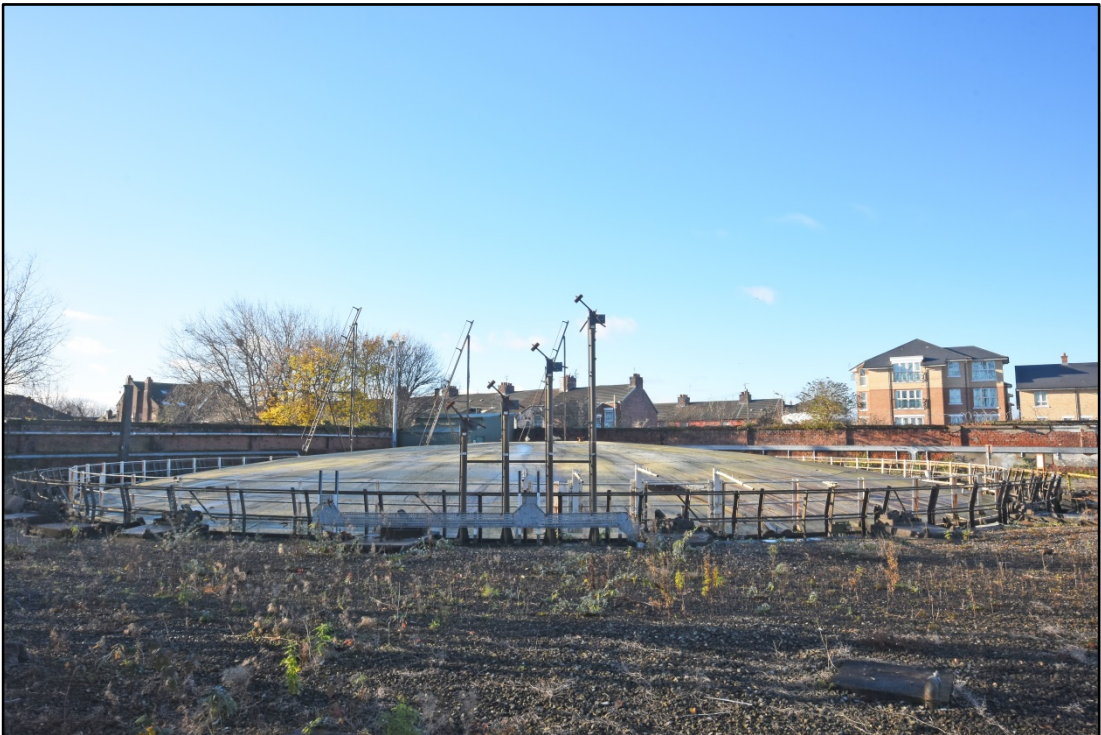
General view of Gasholder 2, looking south-west Fig 30
