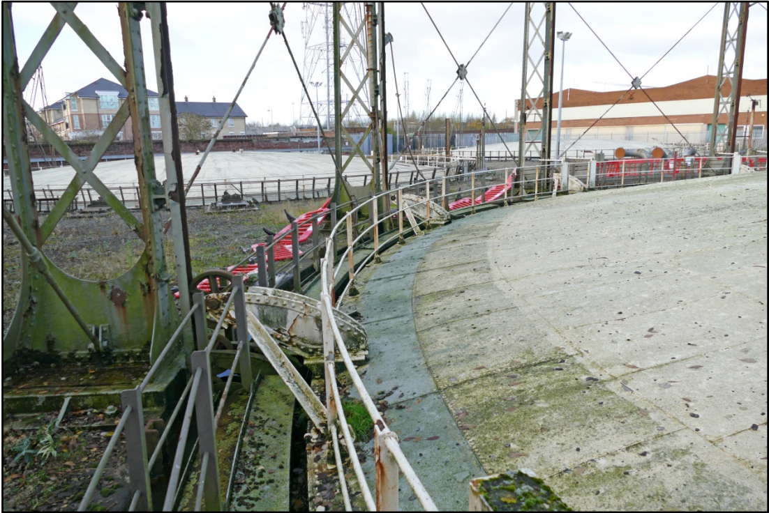
General view of the tanks, grips and roller carriage arrangements, Gasholder 1 Fig 13
