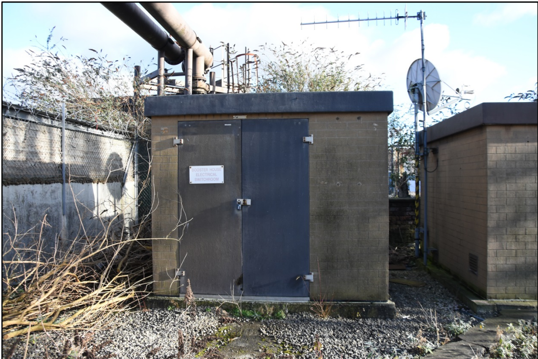
The Booster House and Electrical Switch Room Fig 46
