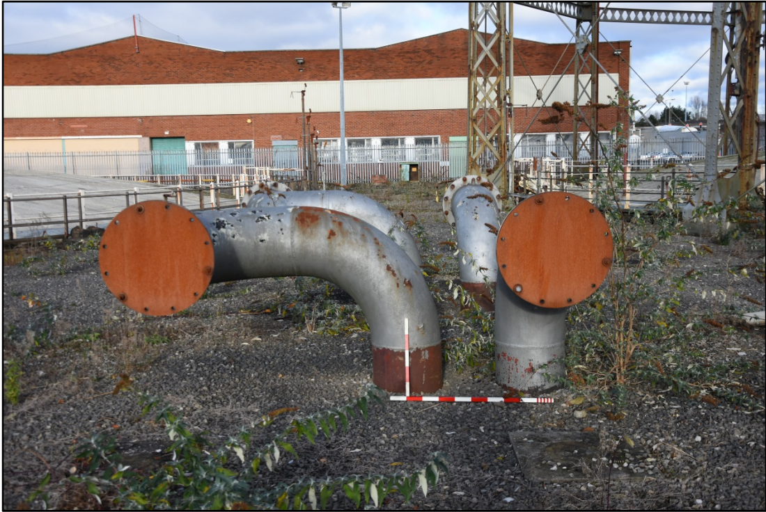
Defunct pipework marking the position of the former Valve House, looking north Fig 45
