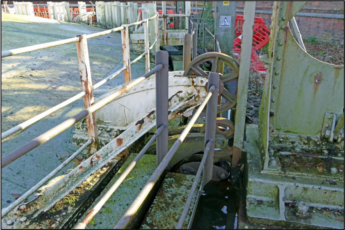
The arrangement of roller carriages Fig 17
