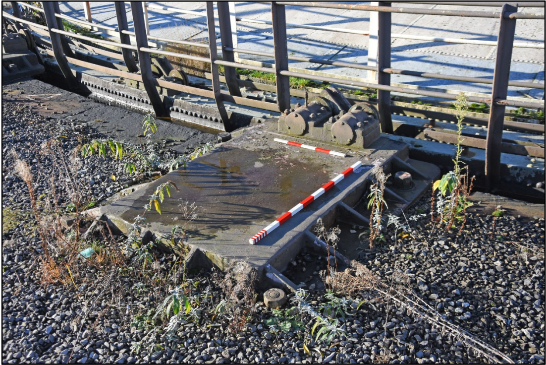
Example of the larger roller carriage footings Fig 41
