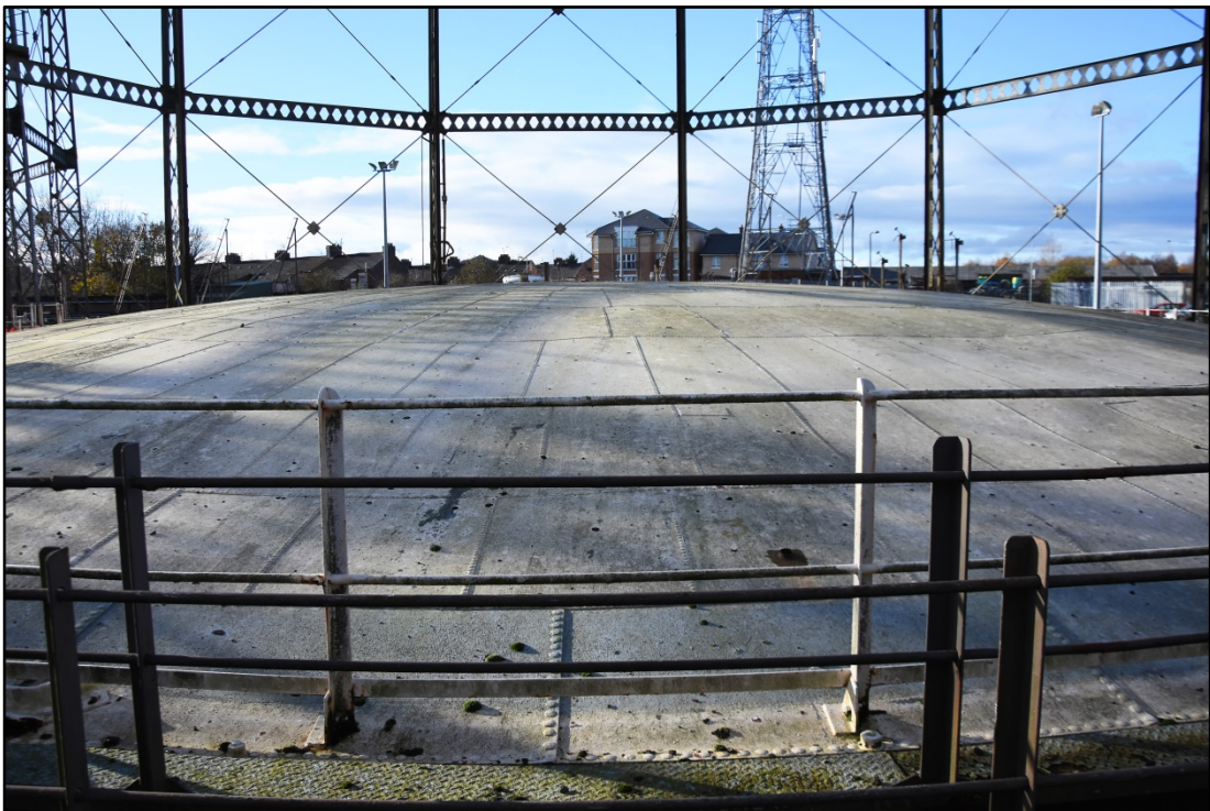
General view of the crown of gasholder 3, looking west Fig 24
