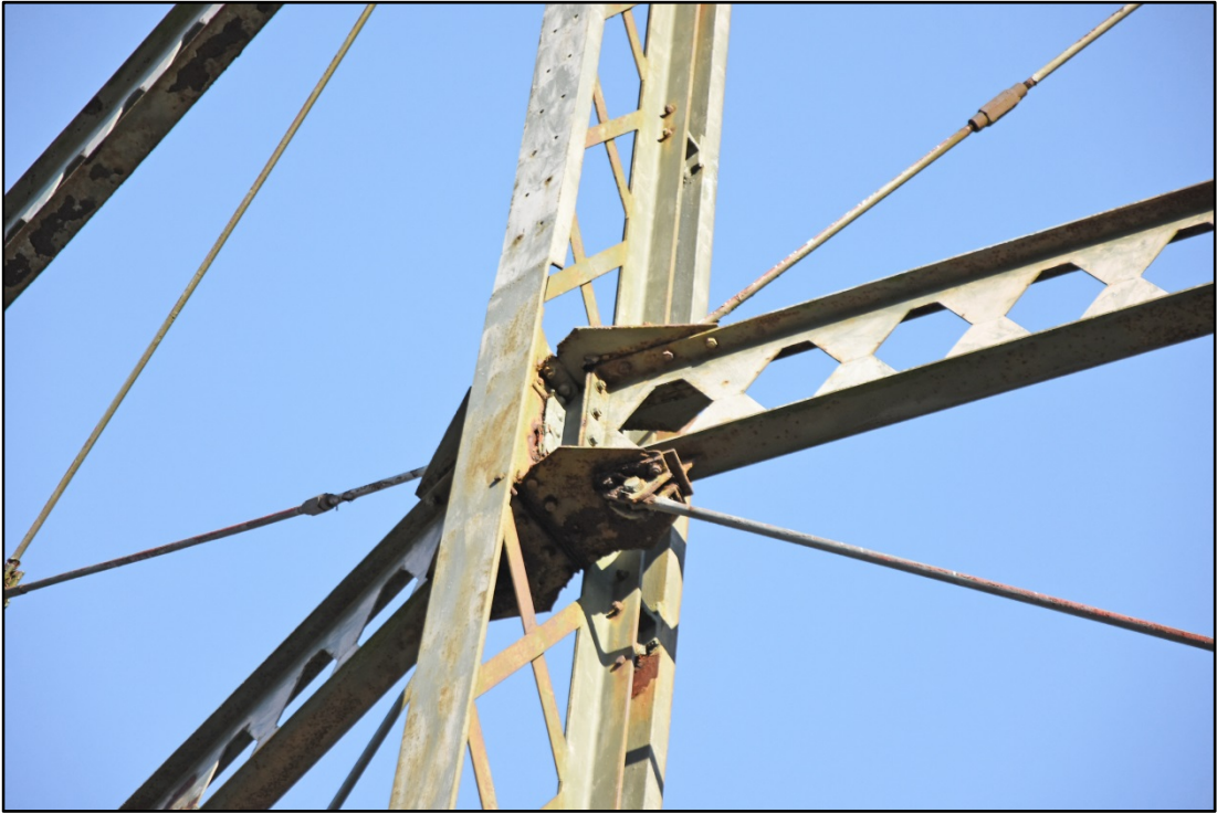
Example of the second tier connections Fig 19
