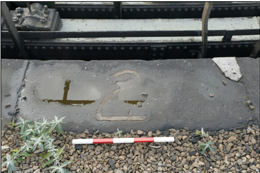
Gasholder designation '2' in the masonry top curb Fig 36
