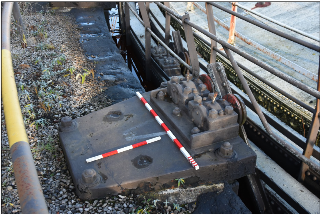
Example of the outer roller carriages. Note stencilled W (west) Fig 32
