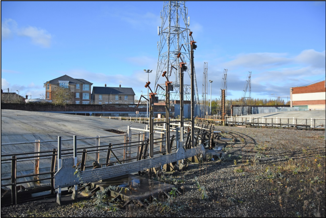
The hammer switches, trips and alarms Fig 35
