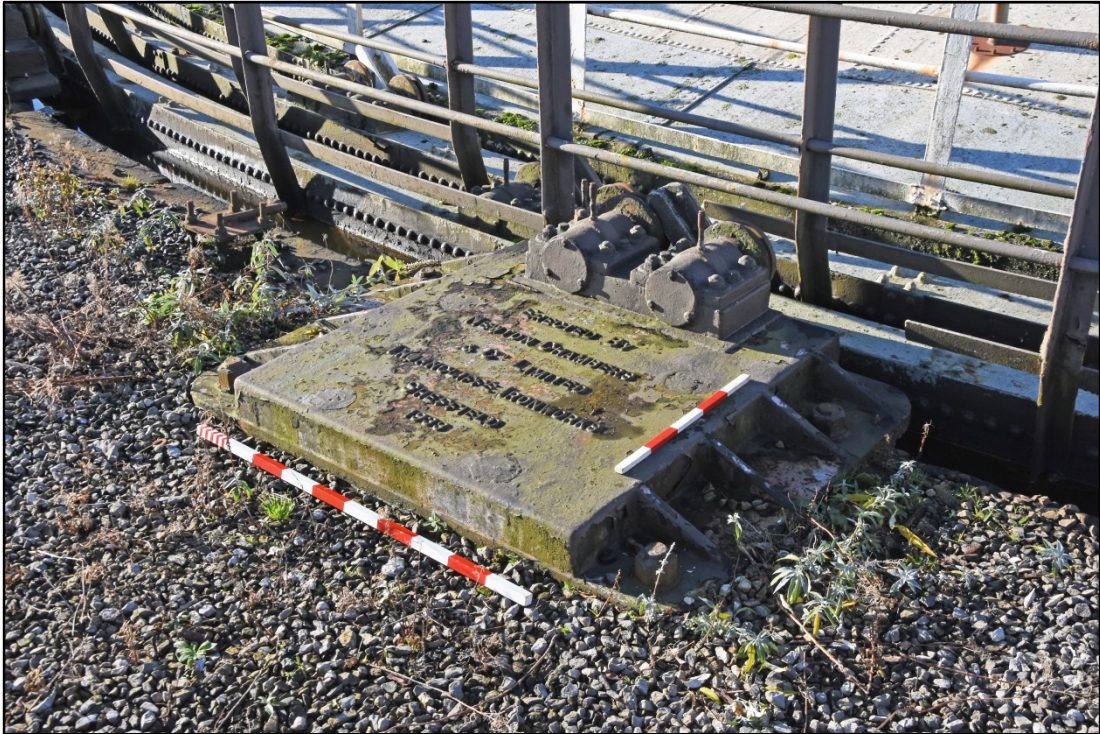
Example of the outer roller carriages with commemorative plaque Fig 39
