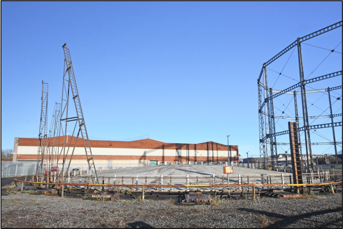
General view of Gasholder 4, looking north-east Fig 37
