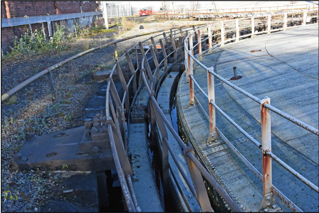
View of the arrangement of tank grips, railings and top curb Fig 31
