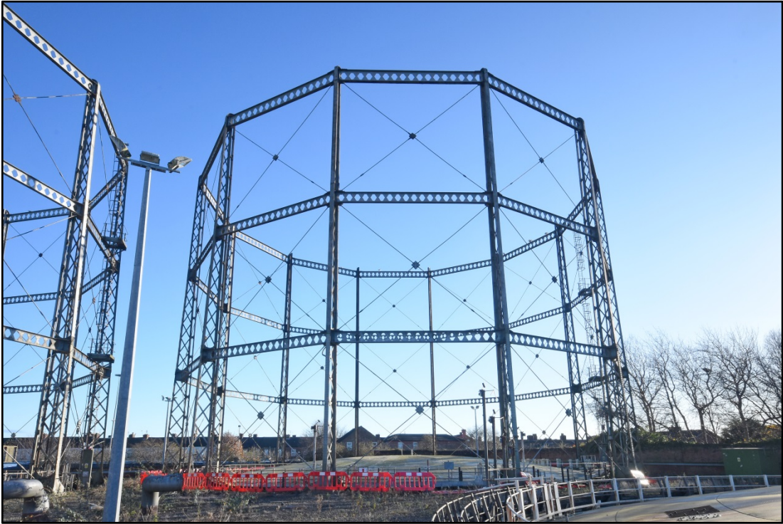
Gas holder 1, looking south-east Fig 11
