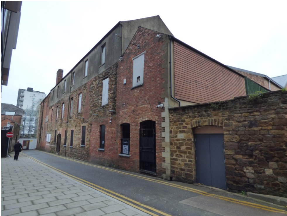
View of the south wall of the Angel Hotel, looking north-west along Angel Street Fig 3
