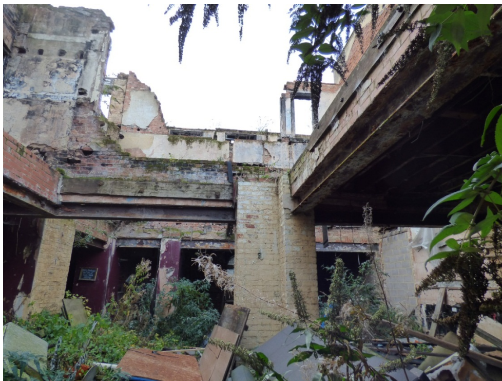
View of ground floor, looking west towards Bridge Street Fig 5
