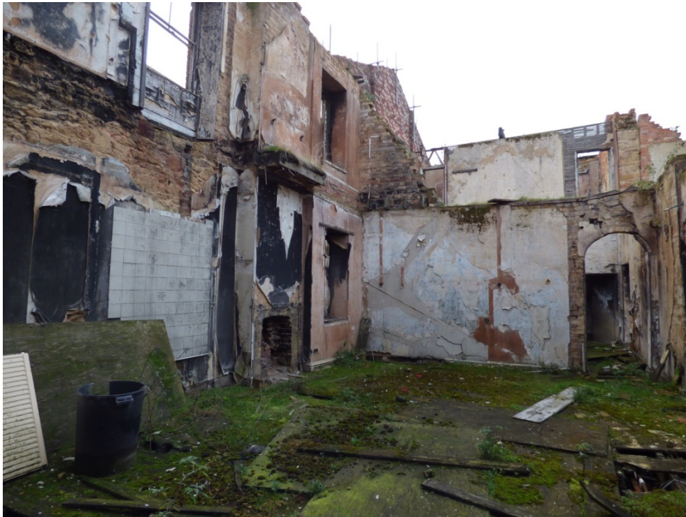
View of first floor, looking north Fig 6
