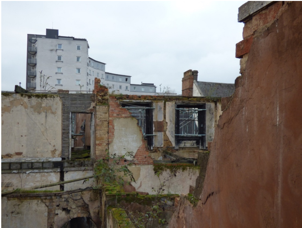
View of second floor, looking north Fig 8
