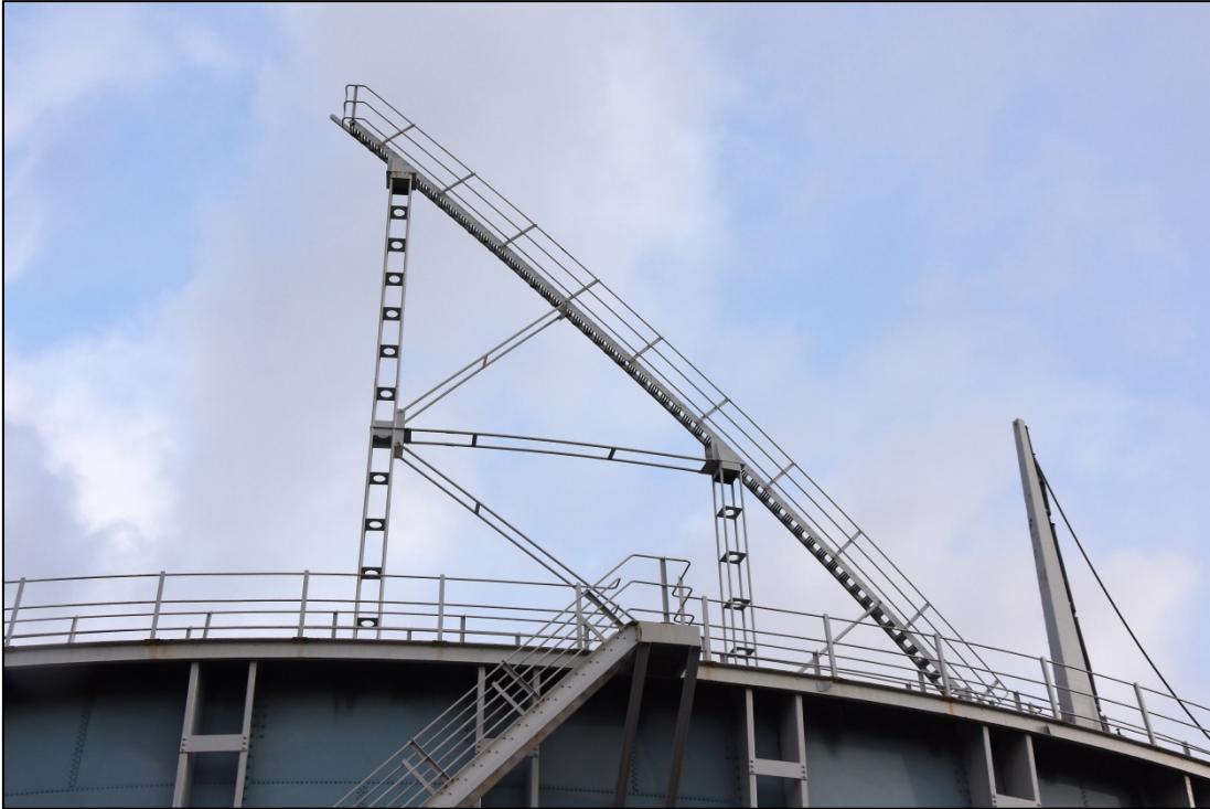
Example of the spiral stairs Fig 25
