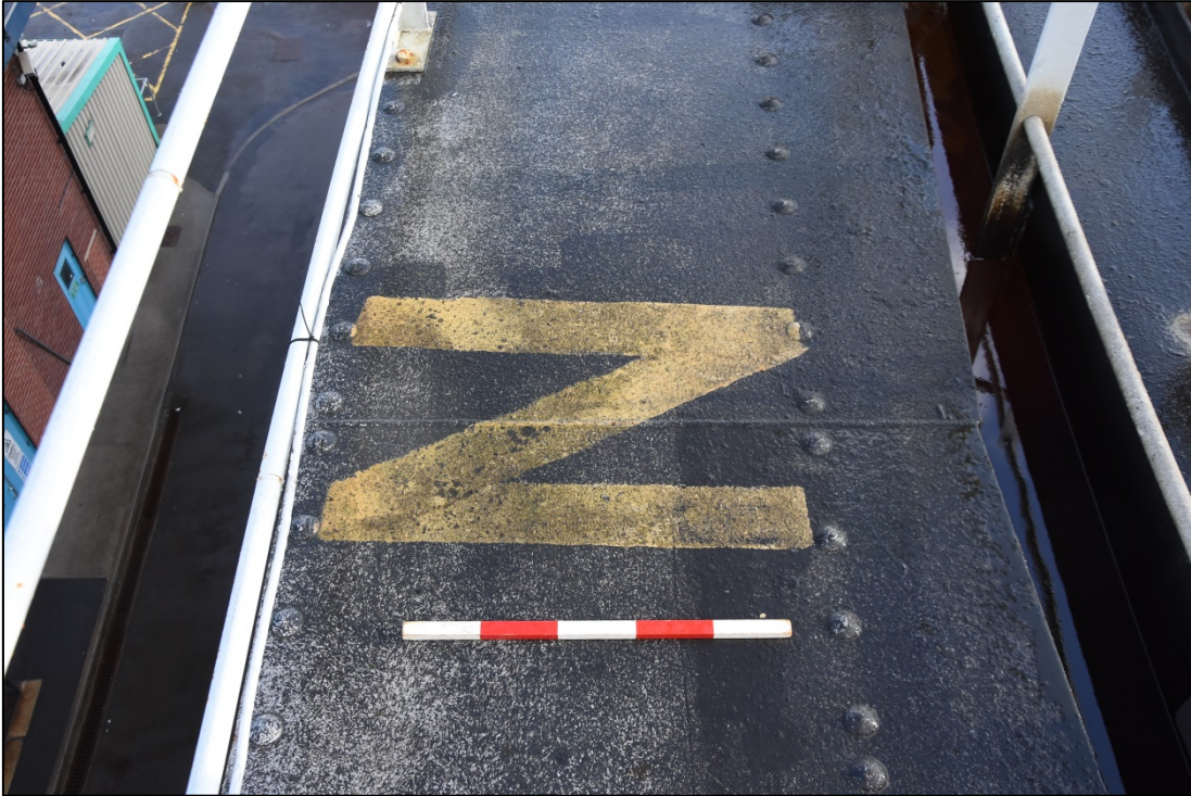
Stencilled N (North) located on the walkway at the north side of the gasholder Fig 23
