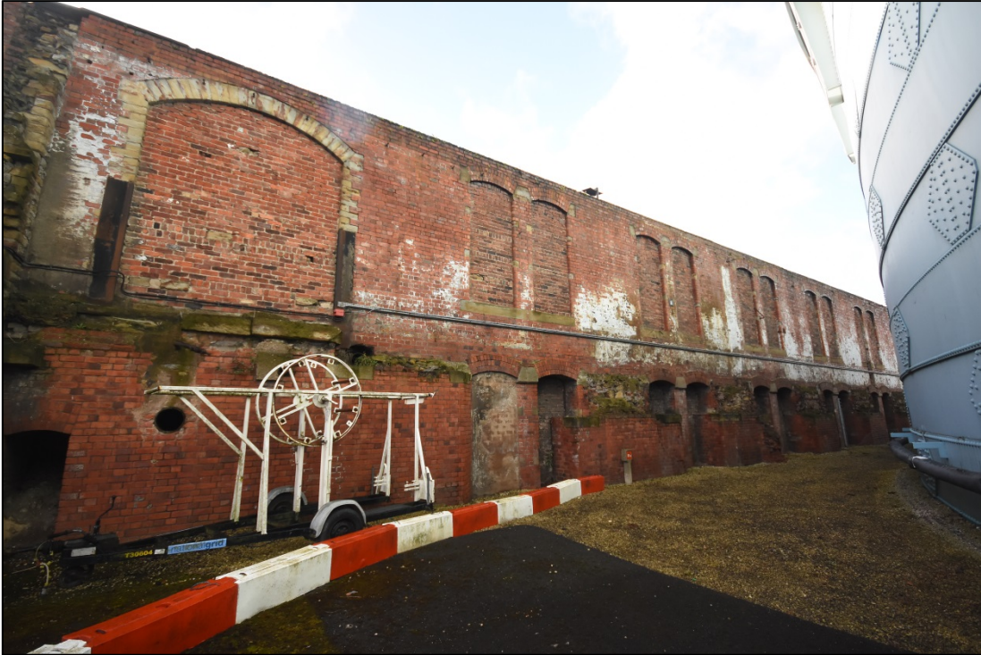
General view of the wall to Sussex Street, showing blocked doors and windows at two levels Fig 35
