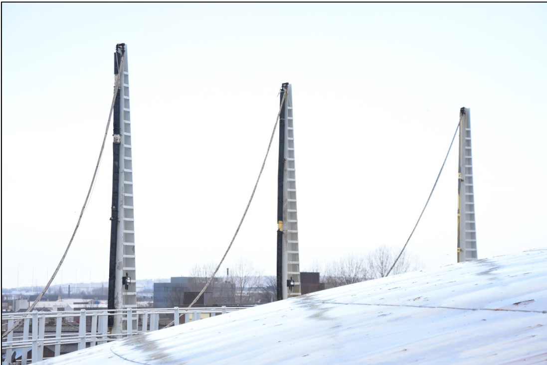
Antifreeze pylons at the south-west site of the gasholder Fig 24
