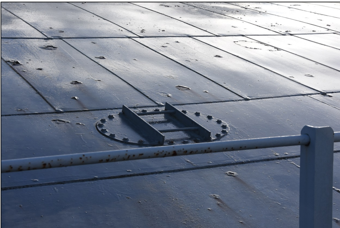
Detail of manhole in the crown Fig 22
