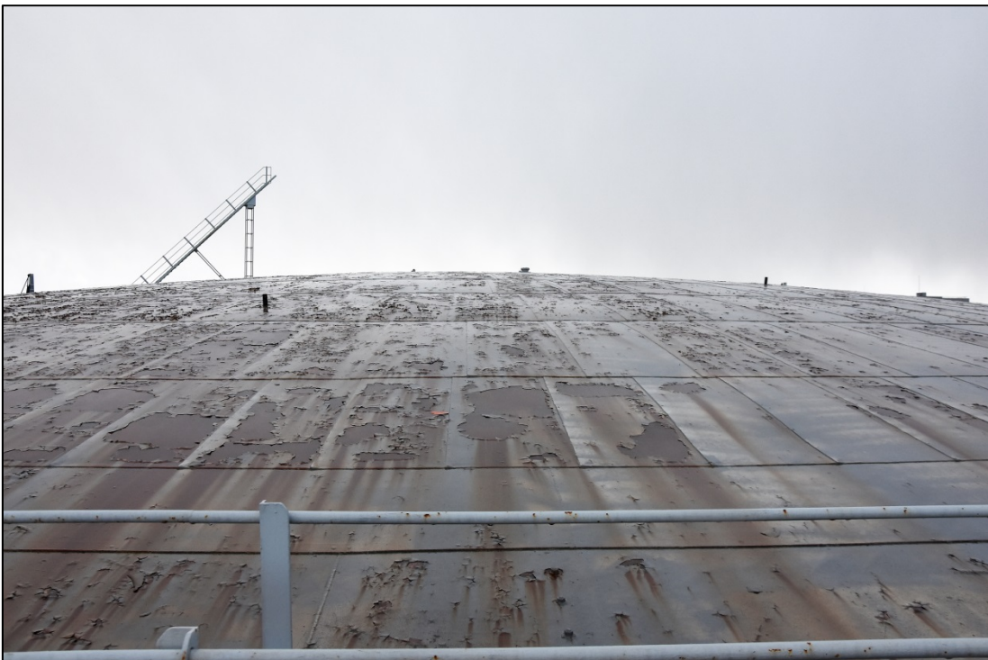
General view of the crown, looking east Fig 20
