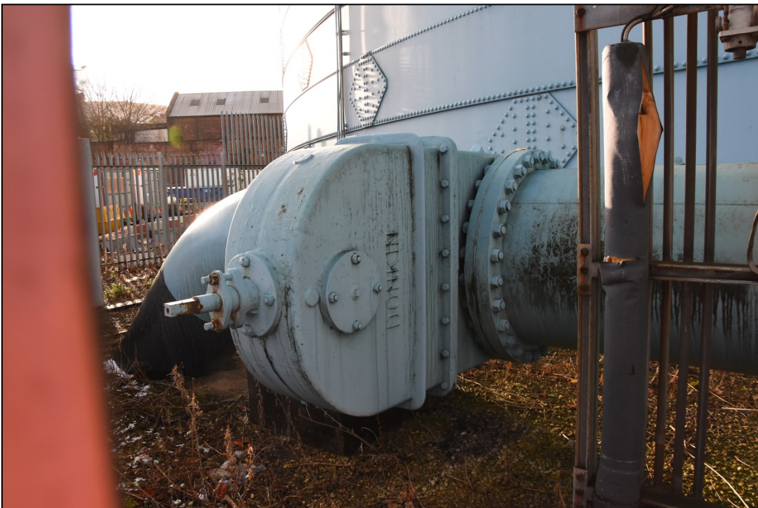
Detail of Donkin flow valve Fig 32
