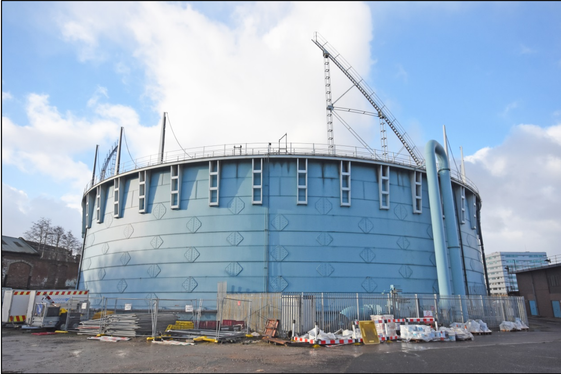
General view of the gasholder, looking south-west Fig 11
