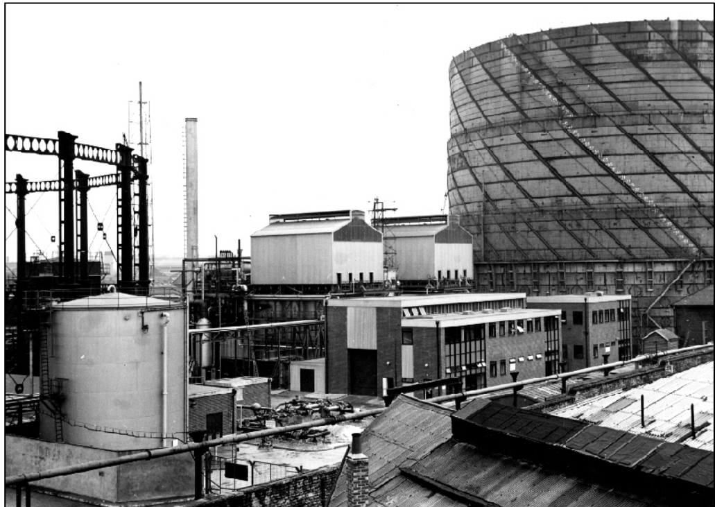
View of the gasworks, 1963-1975, looking north-east (NGA ref XG00914) Fig 9
