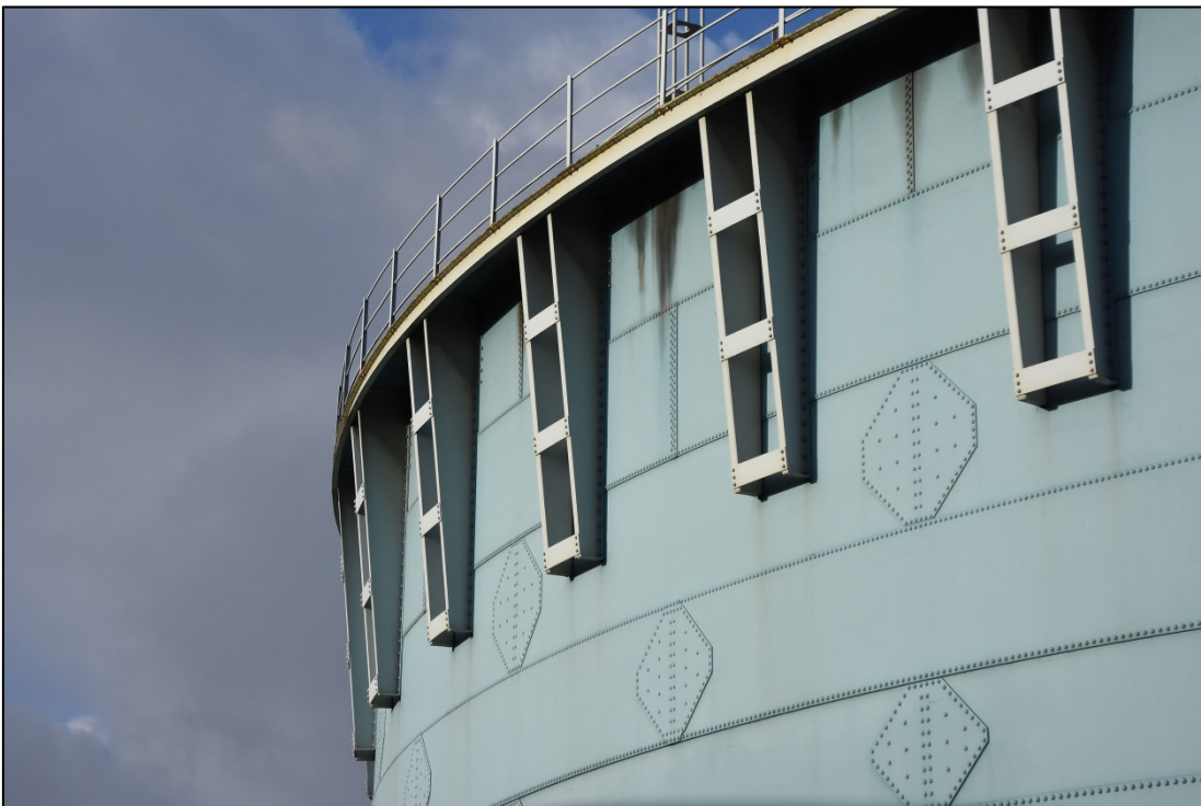
The external brackets supporting the tank walkway Fig 16
