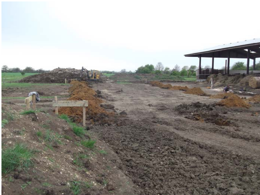
Fig 2 General shot of the 2013 works area of investigation
