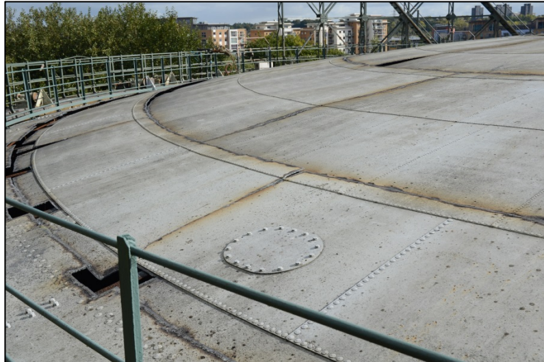
Detail of manhole on the crown Fig 22
