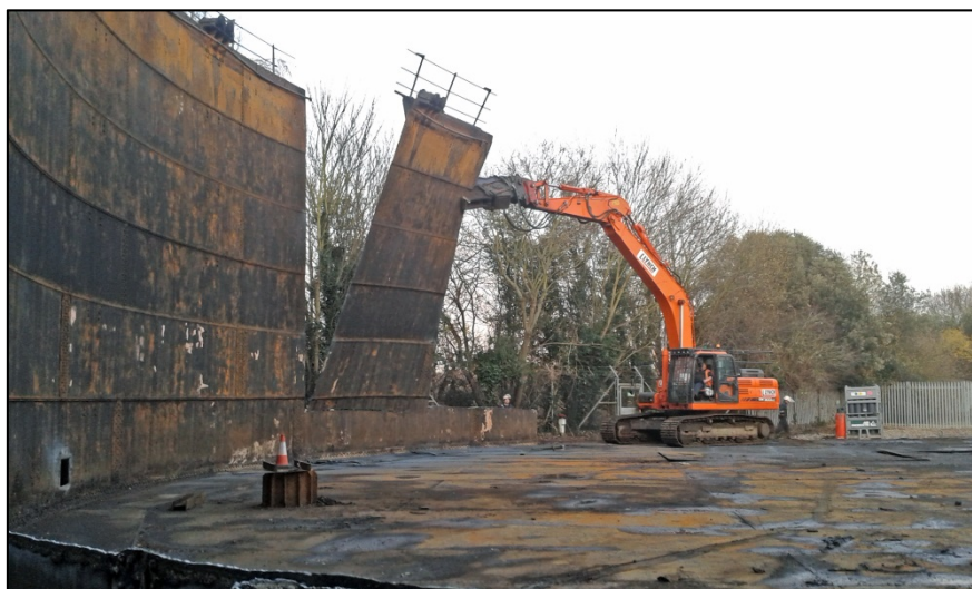
The gas holder tank during dismantling Fig 24
