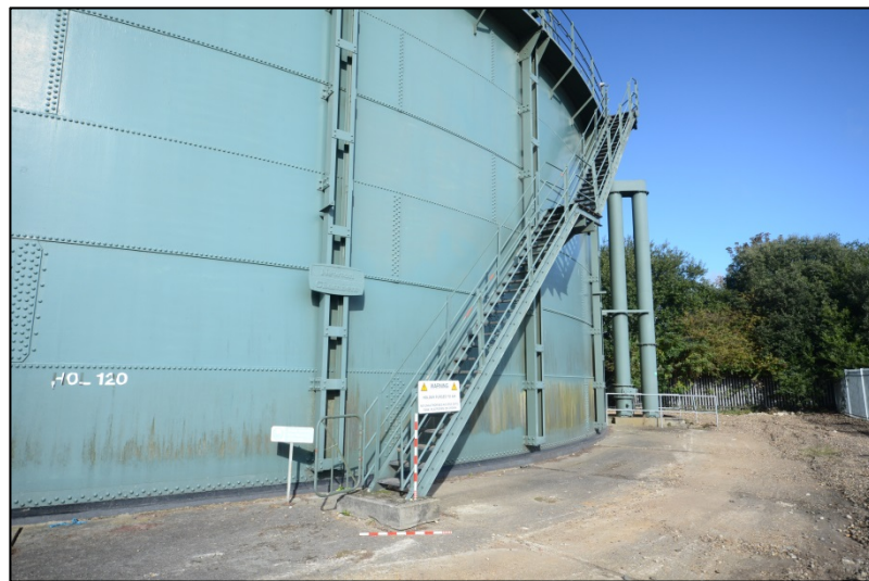
The tank stair, looking north, with inlet / outlet pipes beyond Fig 11
