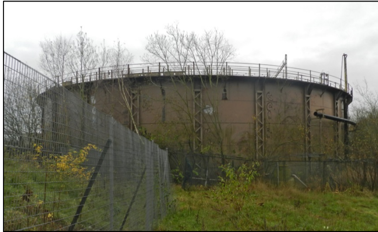
General view of Gasholder 119, looking east Fig 5
