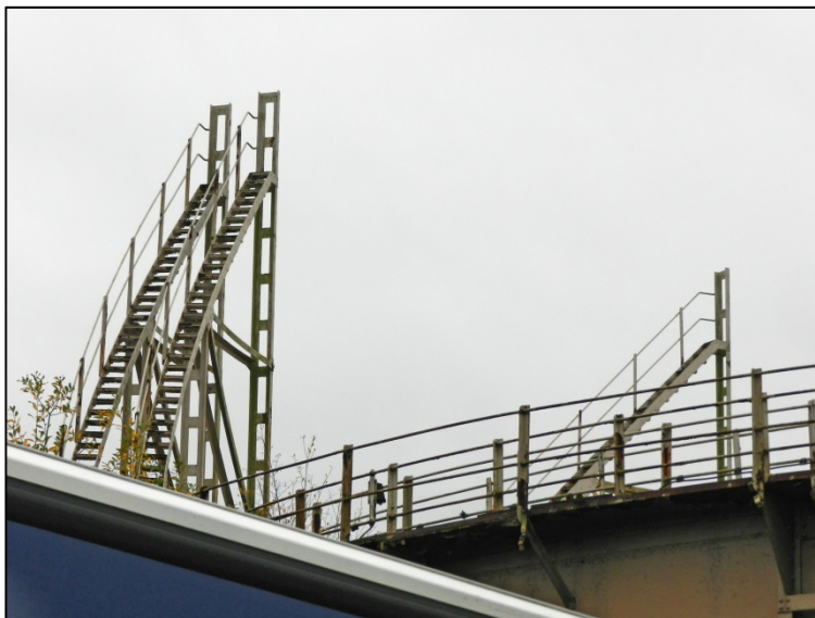
The spiral stairs and railings Fig 7
