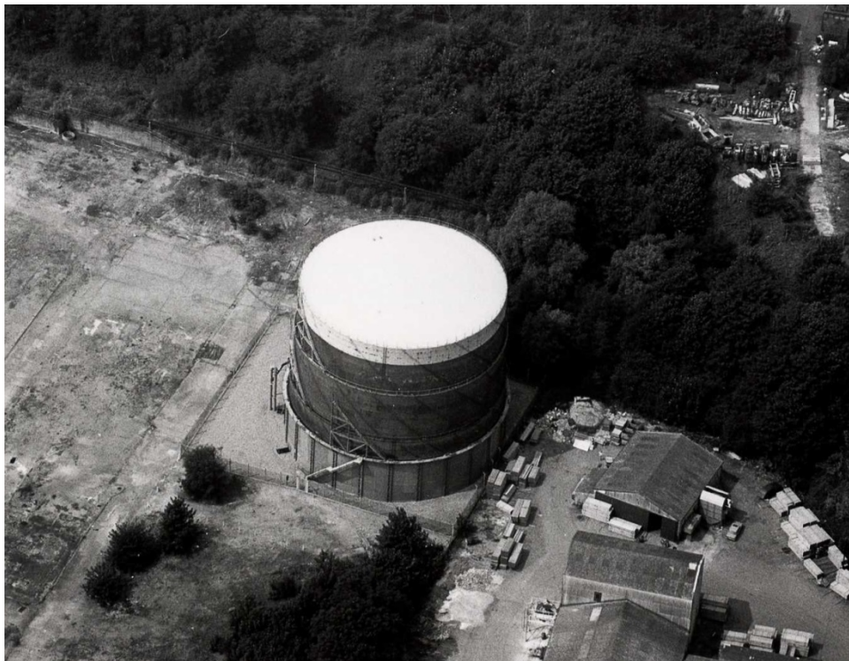
Aerial view of Gasholder 119, c1980s (EA/DX/E/F/2) Fig 4
