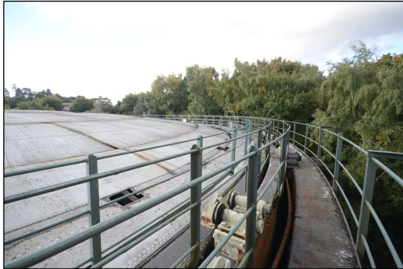
View of the tank walkway, lifts and railings Fig 16
