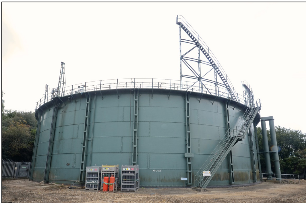
General view of Gasholder 120, looking north-west Fig 9
