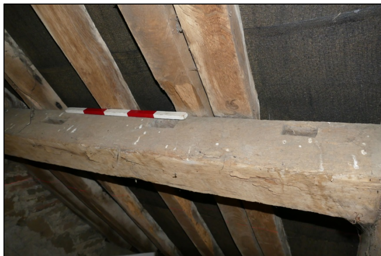
Empty mortice slots on purlin adjacent to Truss N4 Fig 258
