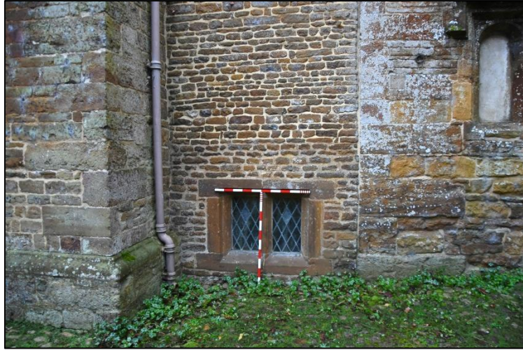
The join between the tower and south-east extension Fig 68
