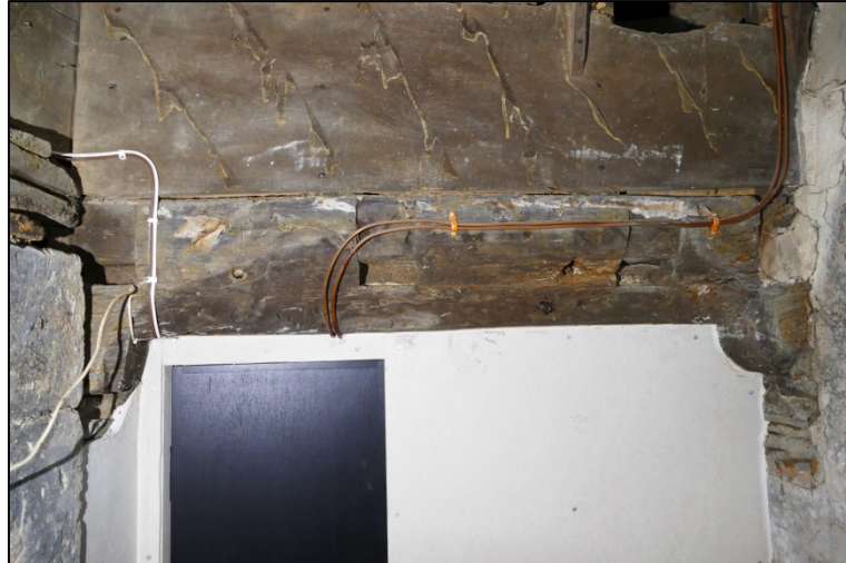
Tie beam with carved door head over the stair entrance Fig 210
