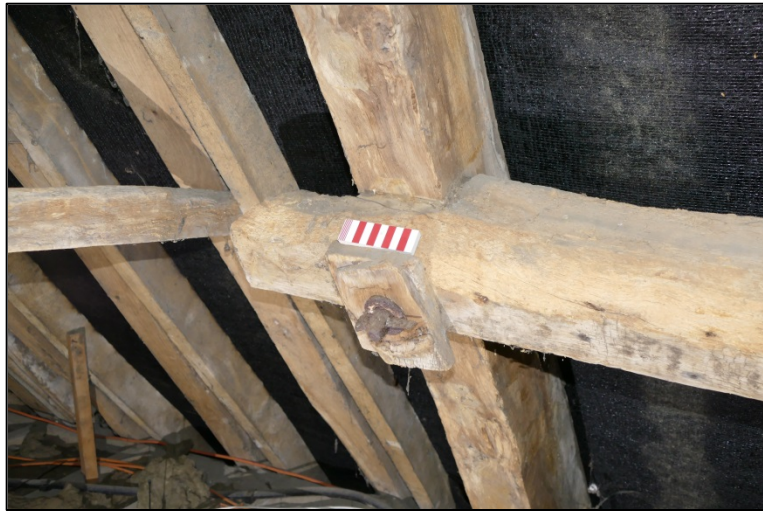
Detail of forelock bolt Fig 239
