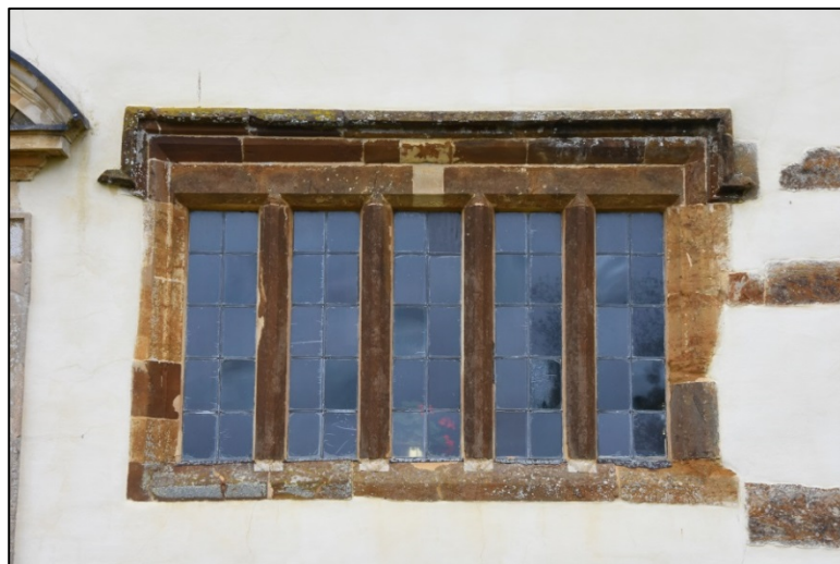
The ground floor tower window Fig 34
