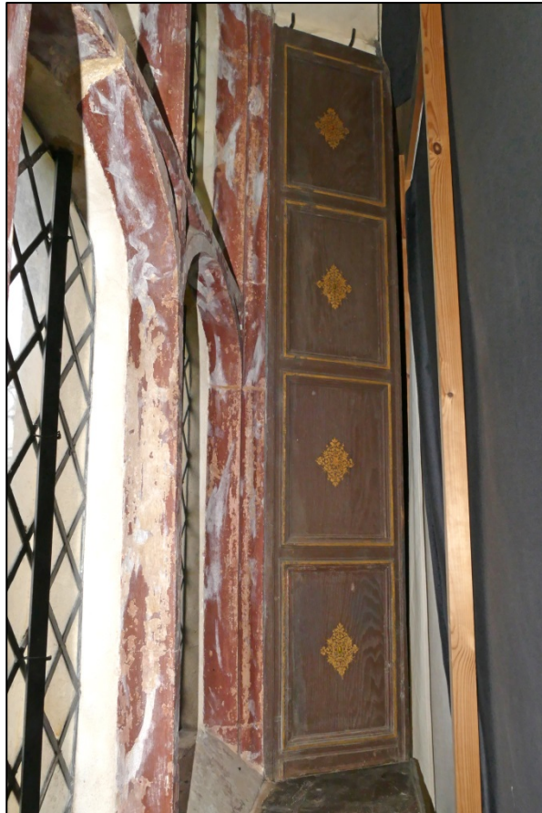
Detail of the panelled reveals Fig 21
