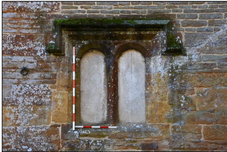
Blocked window to the Tower Fig 69
