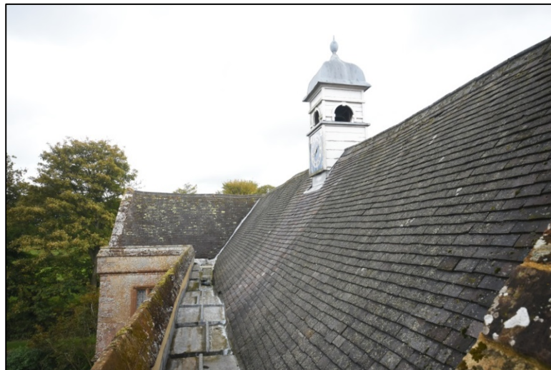
View along the parapet, looking north Fig 28
