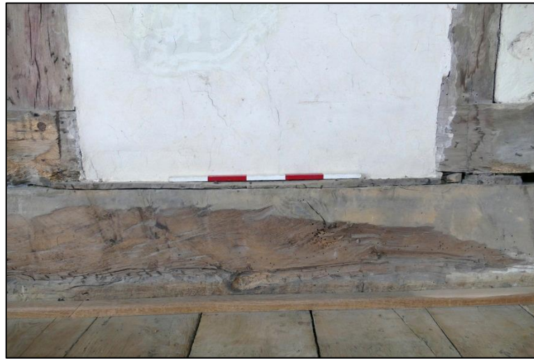
Truncated floor boards at the base of the former door Fig 159
