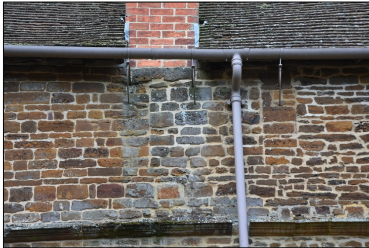
Blocked window to the Long Gallery Fig 75
