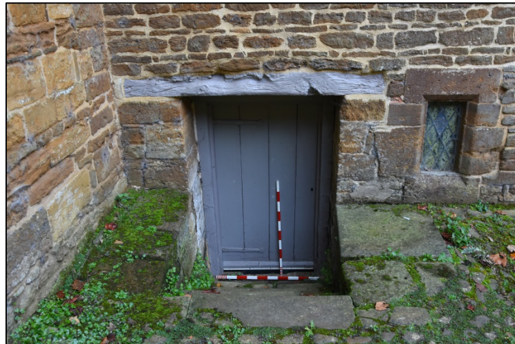
Door to the cellar with former tower window adjacent Fig 73
