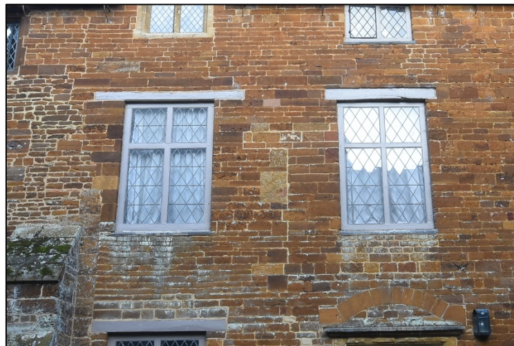
Blocked window and change in fabric Fig 54
