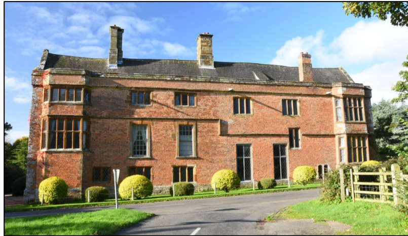
General view of the north elevation Fig 7
