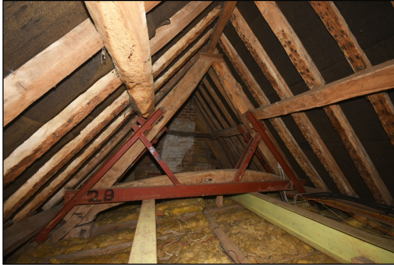
The west face of Truss N3, looking east Fig 250
