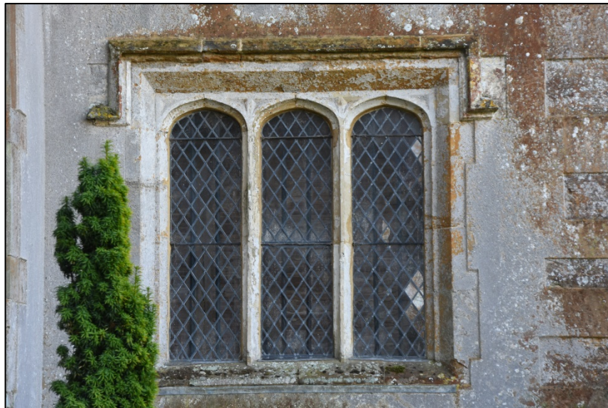
Window to the Dining Room, blocked internally by panelling Fig 22
