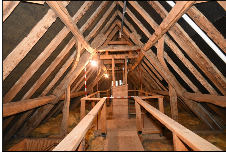
The west range roof, looking south Fig 268
