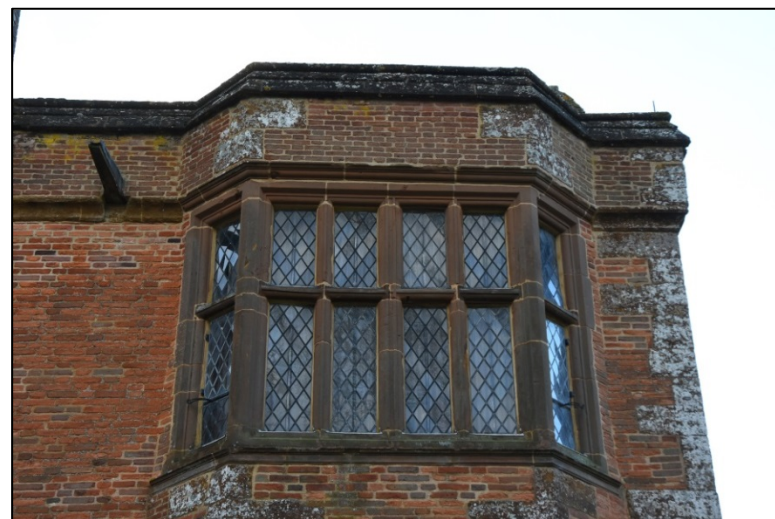
The upper western bay window Fig 12
