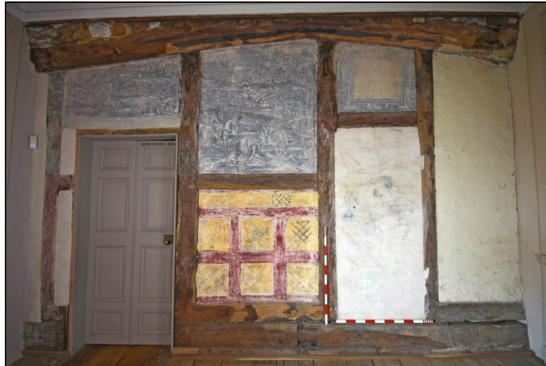
The west wall of Spenser's Room Fig 153
