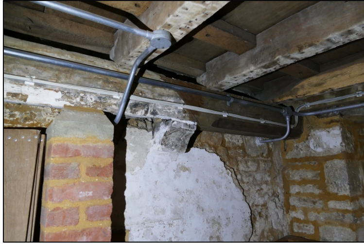
Bracket supporting the western bridging beam Fig 89
