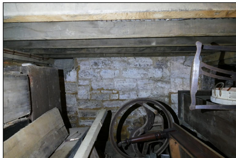
Blocking in the south wall of Room C6 Fig 97
