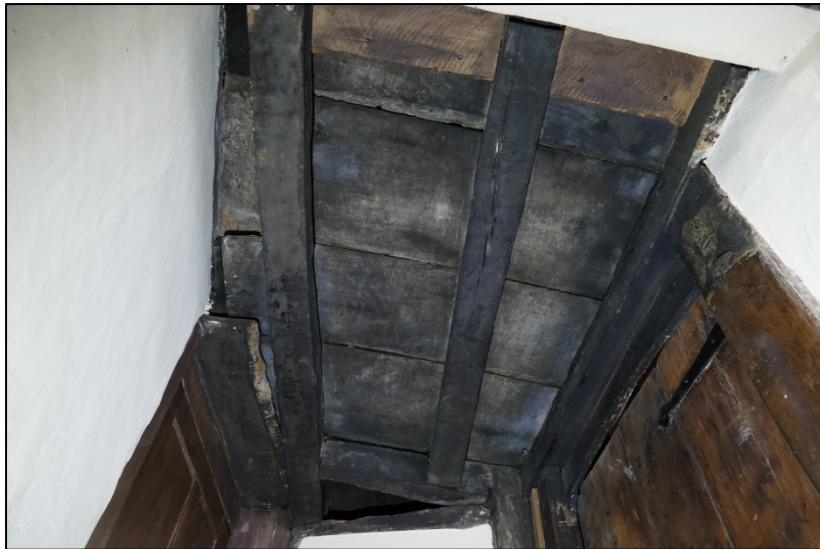
The underside of the Lobby ceiling Fig 150
