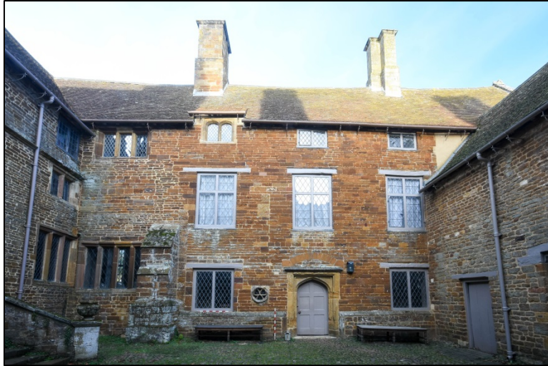
The north courtyard elevation Fig 50
