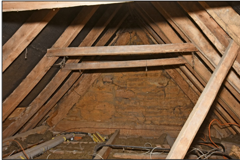
The join between the east and south ranges, Truss E1 Fig 236
