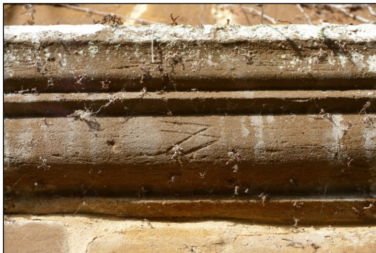
Detail of Marian or Masons mark on window lintel Fig 47
