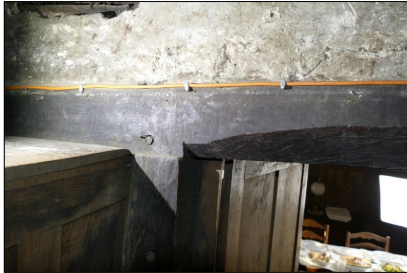
Shaped door head over alcove entrance Fig 144
