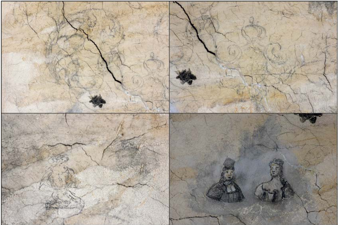
Detail of small graffiti on the west wall Fig 156
