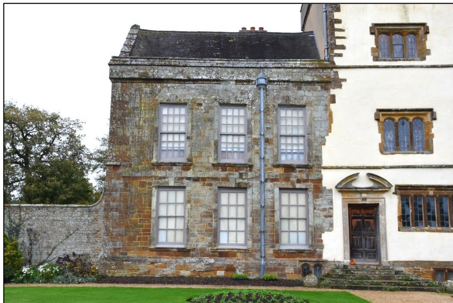
The western extent of the south elevation Fig 31
