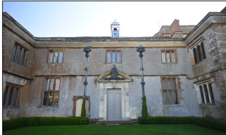
The central part of the west elevation showing the blocked cross-passage door and early 18th-century doorway, and the symmetrical arrangement of windows Fig 23
