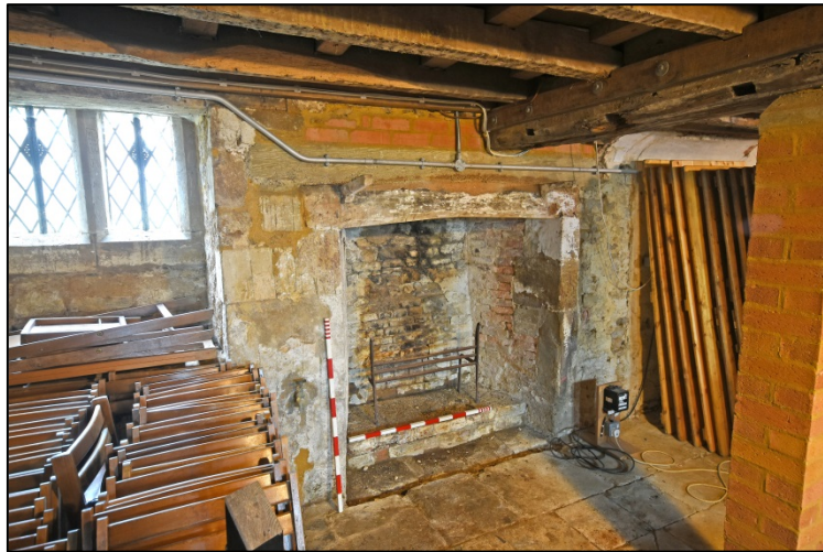
The fireplace in Room C3 Fig 87
