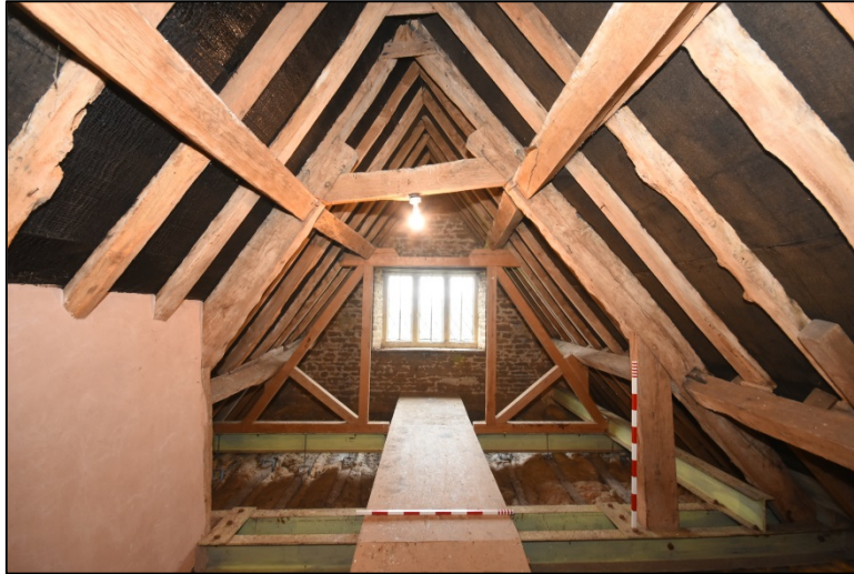
The north-west roof, looking west, showing Truss N7 Fig 260
