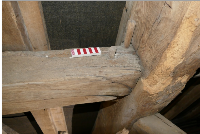
Truss N4, detail of double pegged scarfed bridge joint Fig 256
