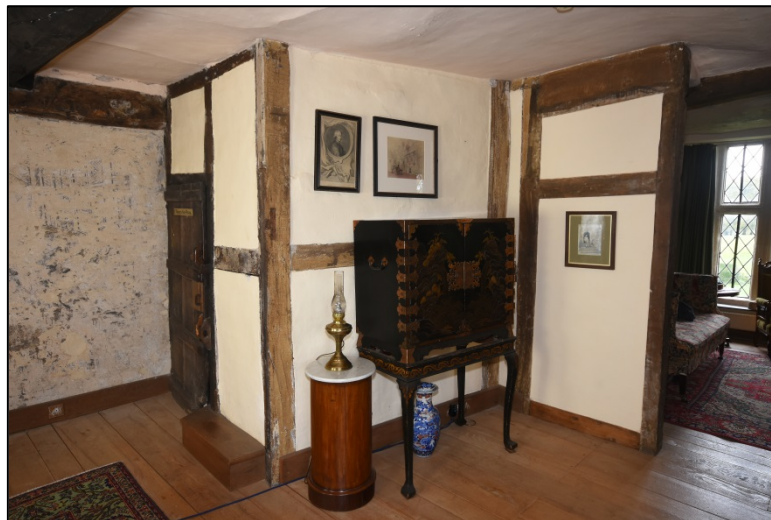
The stairwell viewed from the Sitting Room Fig 176
