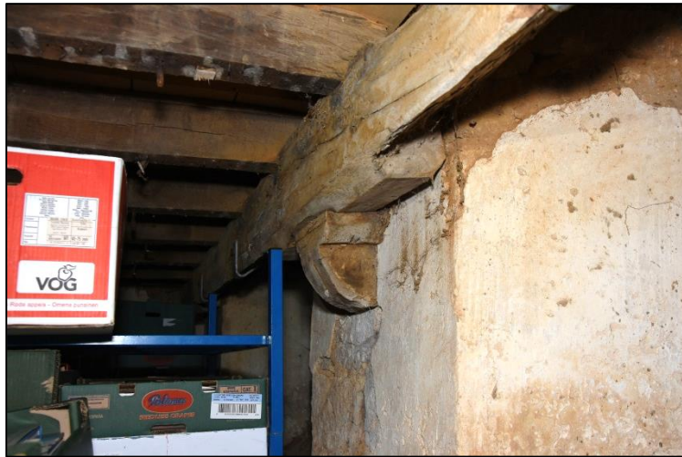
Timber bracket holding the lowered rail Fig 84
