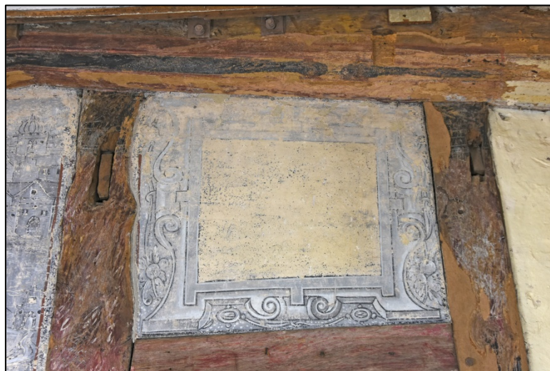
Defunct mortices with truncated tenons in situ Fig 155
