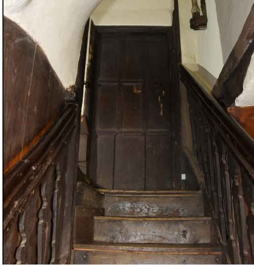
The stairwell approach to the Sitting Room Fig 192
