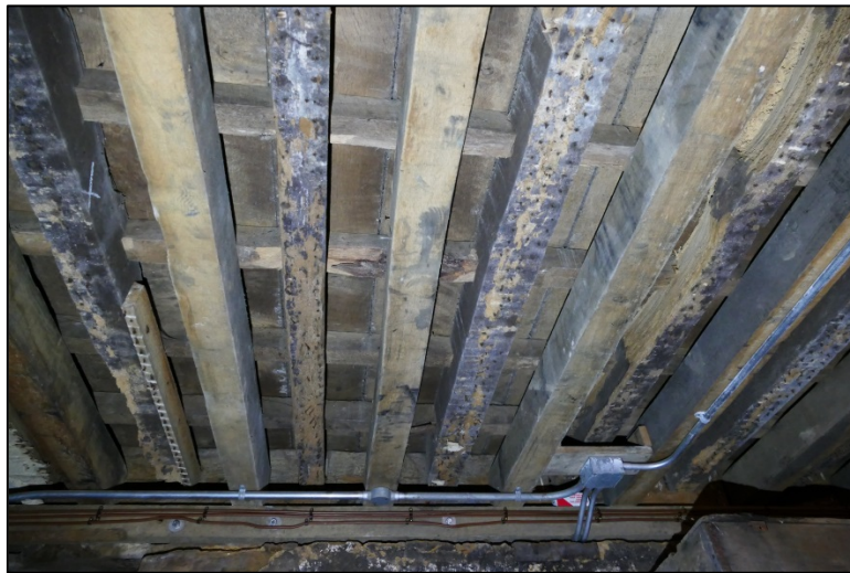
The joist and batten arrangement of the Dining Room floor Fig 96
