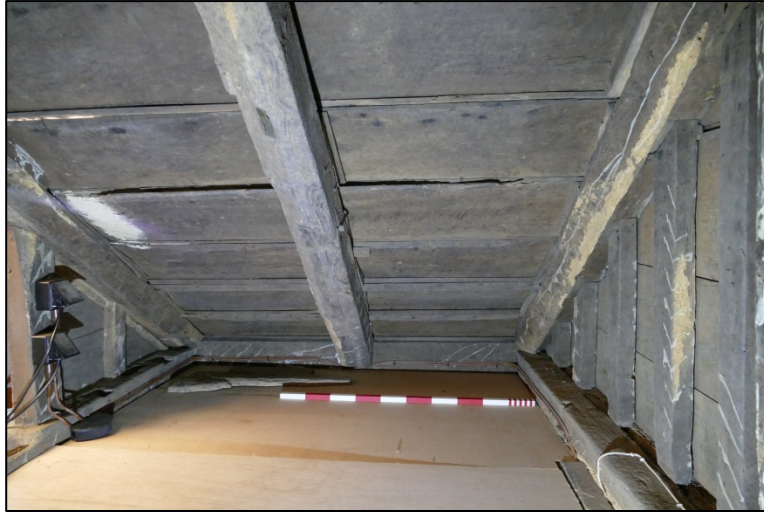
The underside of the stair at the ground floor landing Fig 213
