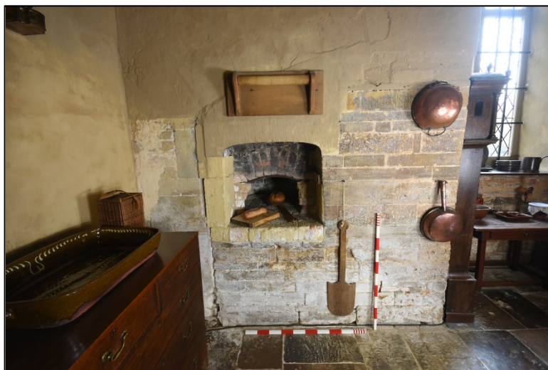
The bread oven; note vertical joint at the left side Fig 130
