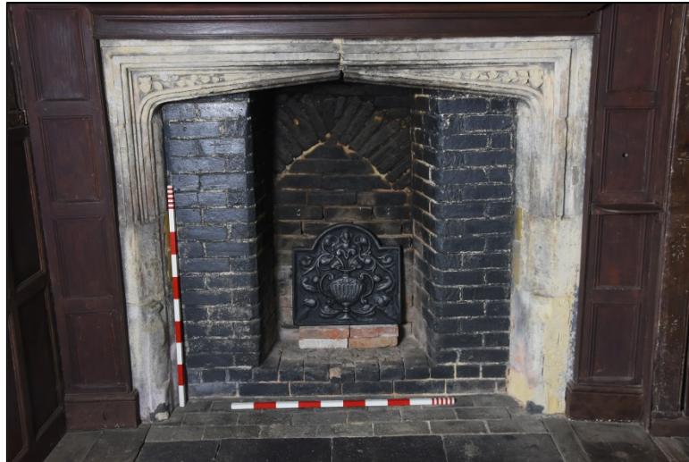
The fireplace; note reduced jambs and brick arch at the back of the flue Fig 138
