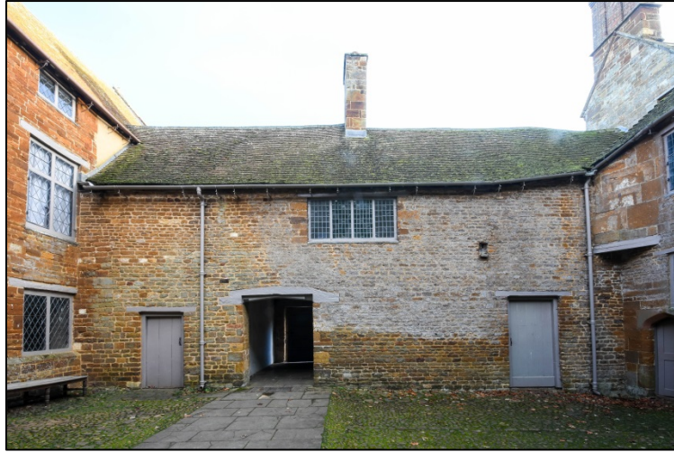
The eastern elevation Fig 57
