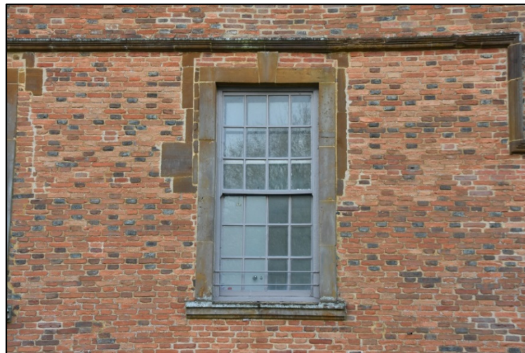
Detail of sash window with remains of blocked mullion window Fig 14
