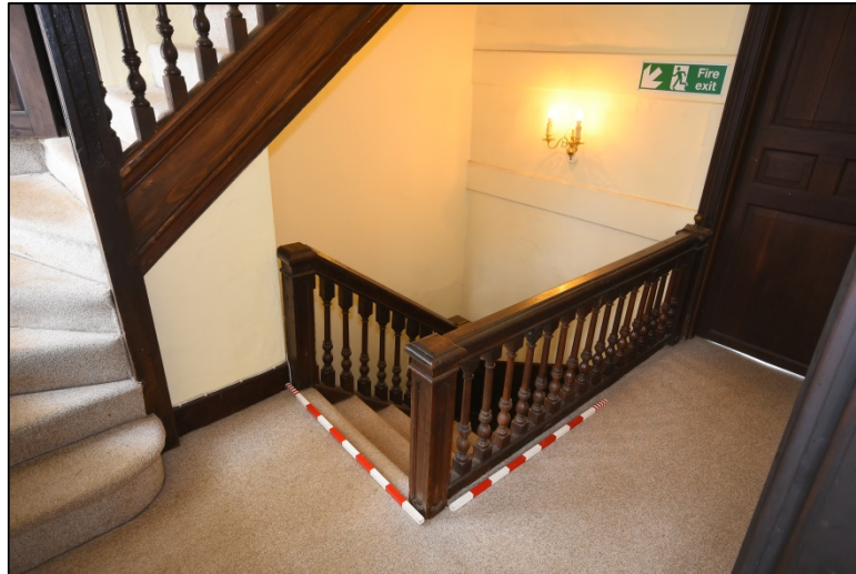
The first floor stair landing Fig 204
