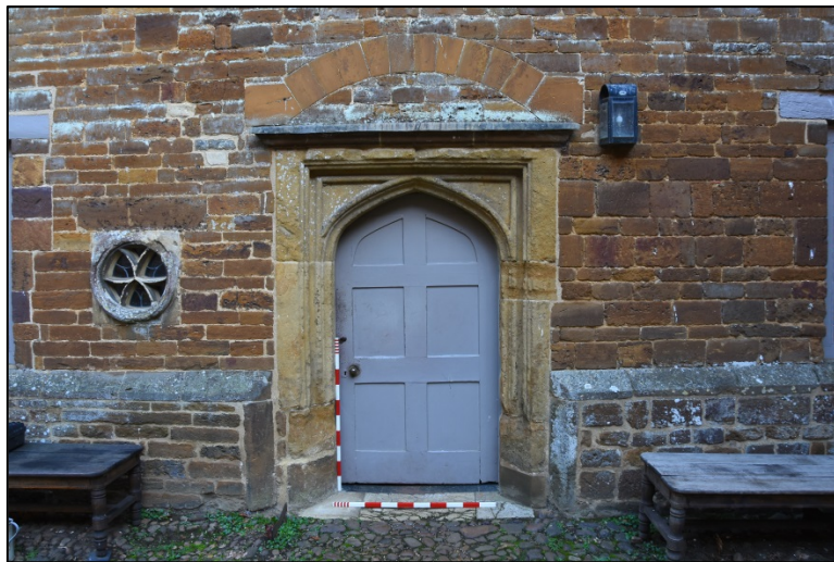
The inserted doorway and window Fig 51
