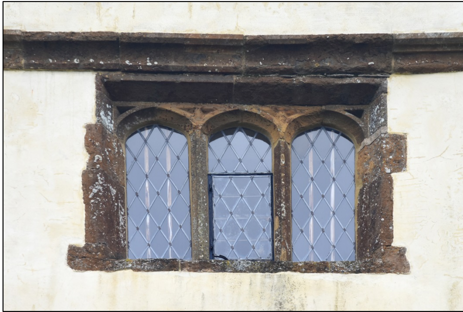
Upper storey tower window Fig 35
