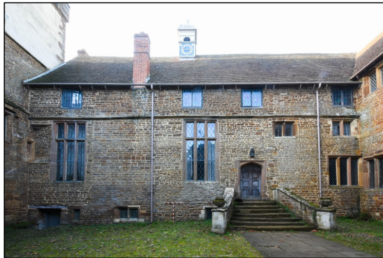
The west courtyard elevation Fig 72
