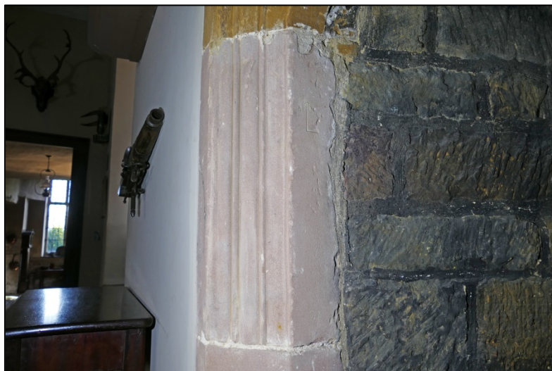
Detail of the fireplace moulding with possible Masons mark Fig 124
