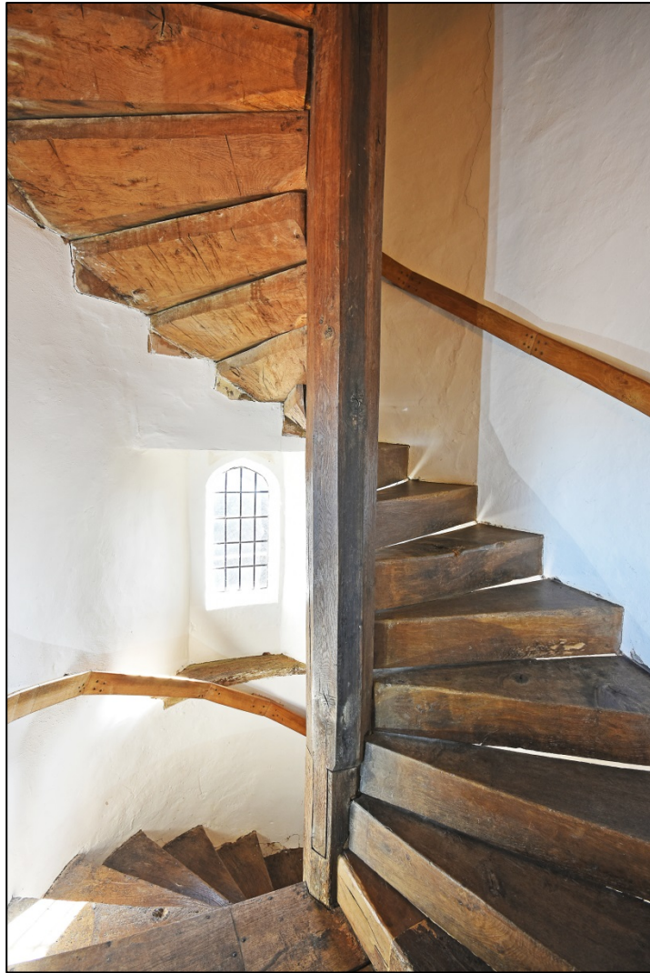
The spiral stair Fig 218
