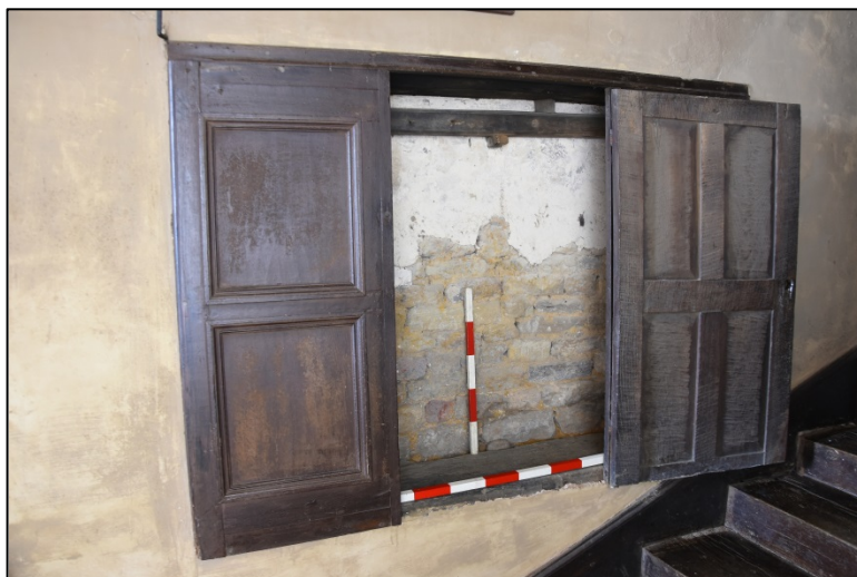
Recessed cupboard adjacent to kitchen stairs Fig 127
