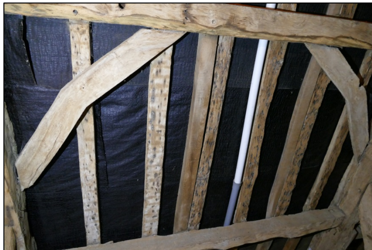
The cranked wind braces; note turned over rafters Fig 272
