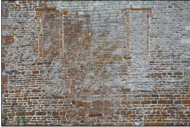
Detail of the blocked oriel window Fig 42
