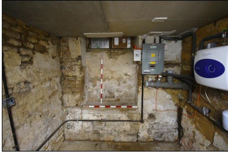
Blocked window in Room C1 Fig 80
