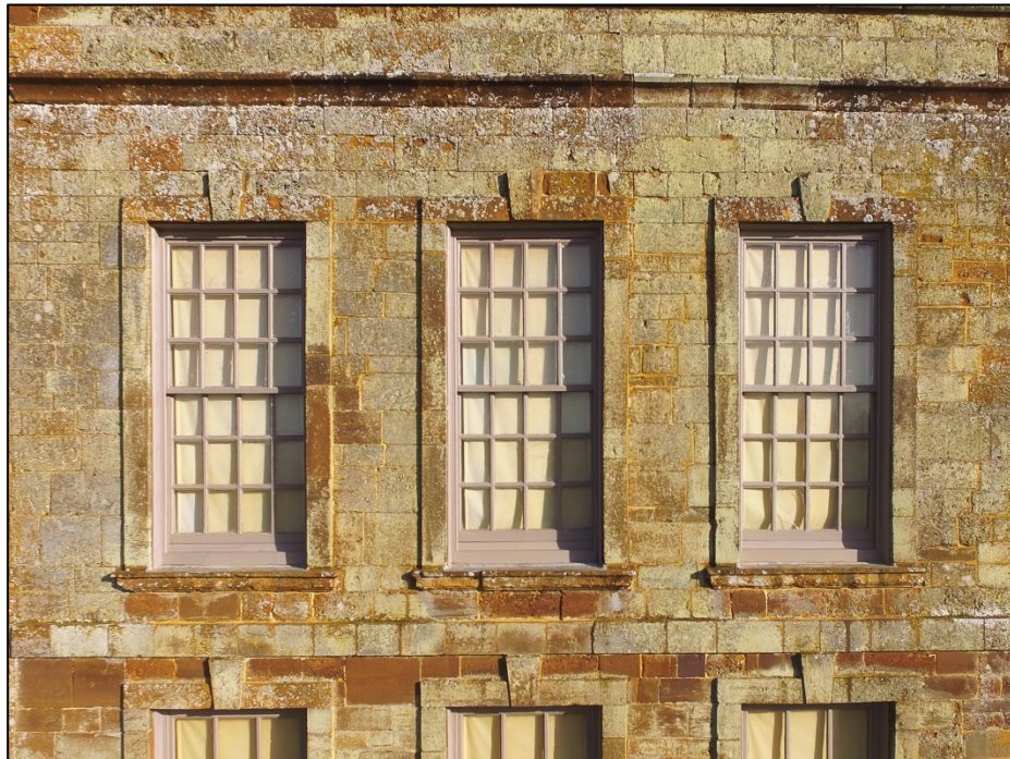
Example of the sash windows Fig 36
