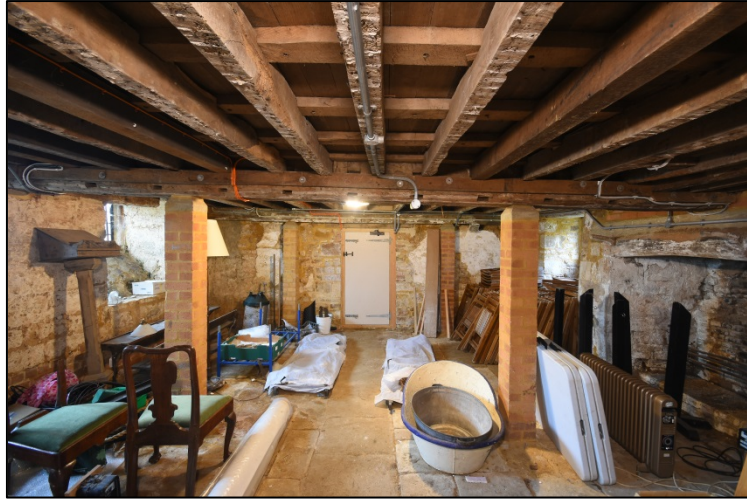
Room C3, the former Dairy, looking west Fig 86
