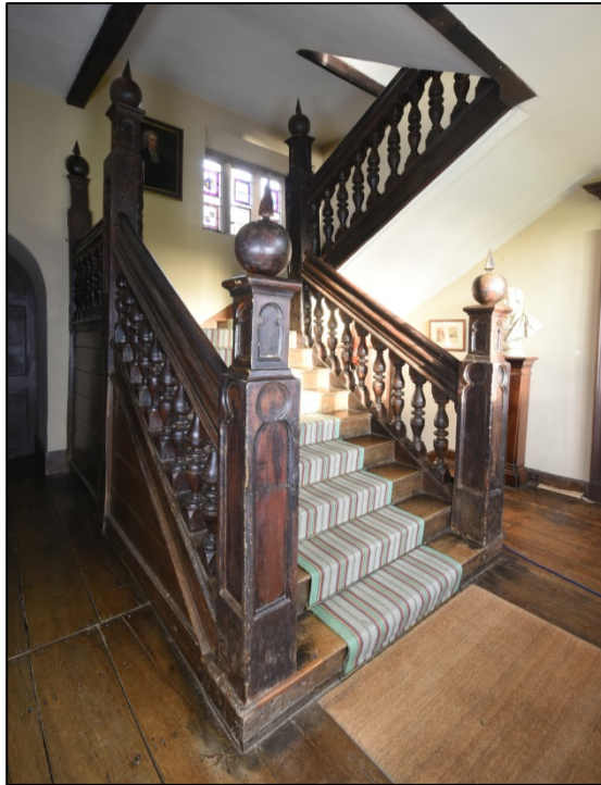
The ground floor stair landing Fig 216
