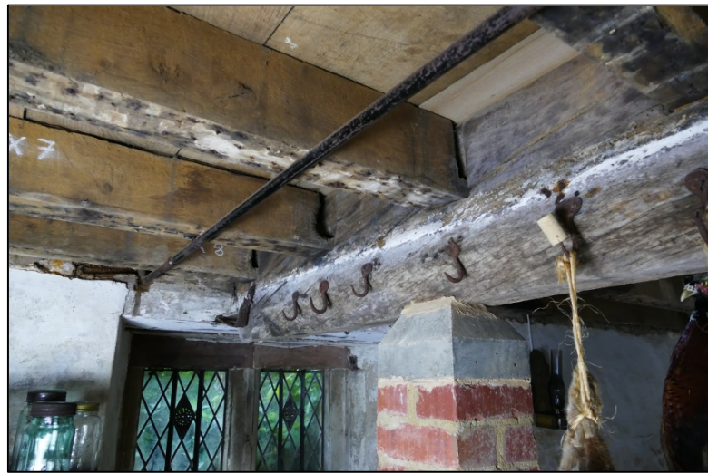
The Larder joist and bridging beam arrangement Fig 102
