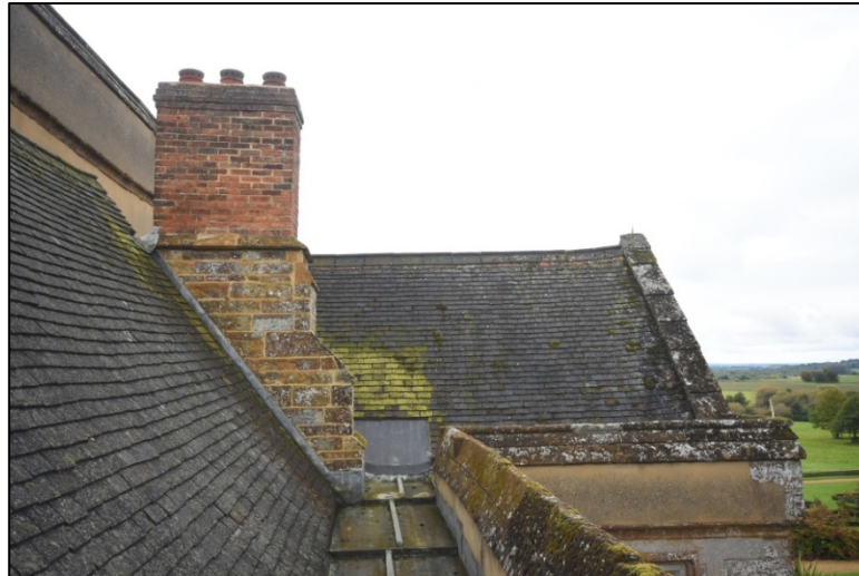
View of the chimney and parapet, looking south Fig 26
