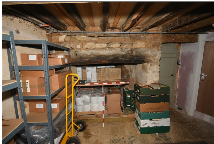
The fireplace in Room C2 Fig 85
