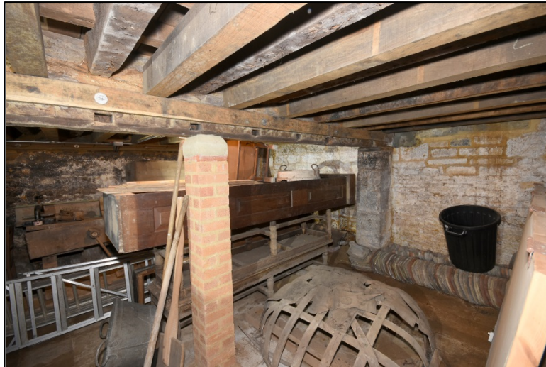
Room C6, looking south-west. Note mortices on underside edge Fig 95
