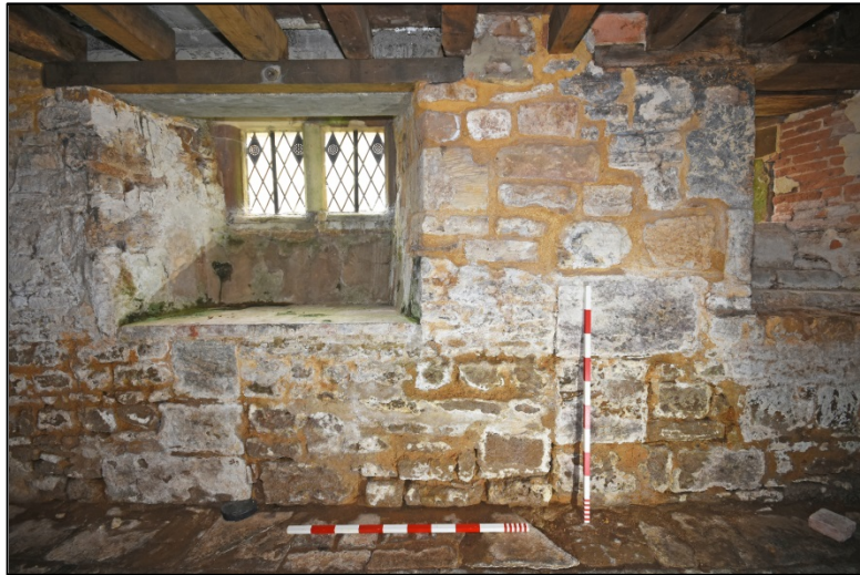
Blocking in the east wall of the corridor Fig 99
