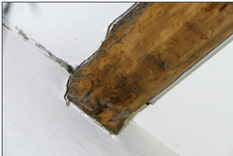
Detail of tie beam stops Fig 111
