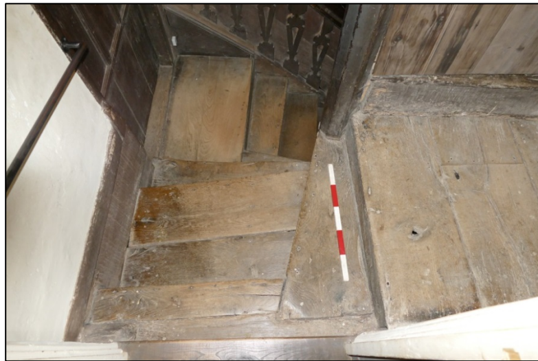
The arrangement of stairs within the stairwell Fig 193
