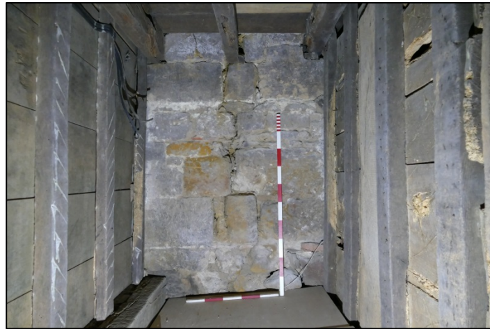
The ground floor landing, looking north Fig 214
