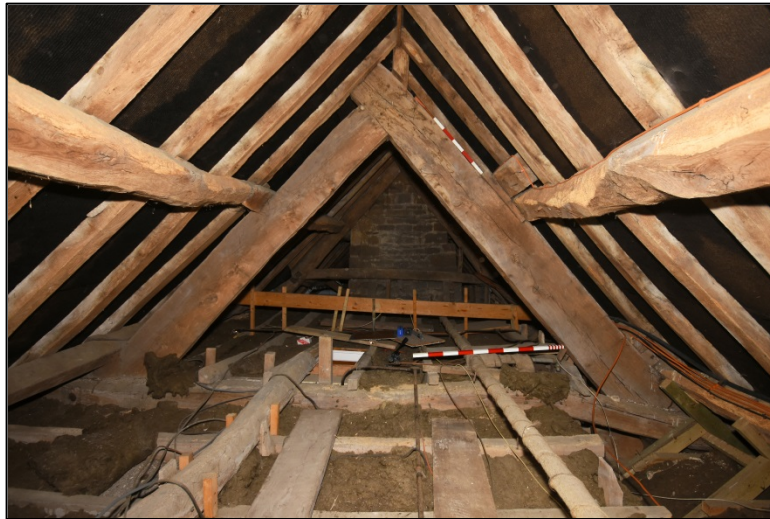
Truss E5, looking south Fig 242
