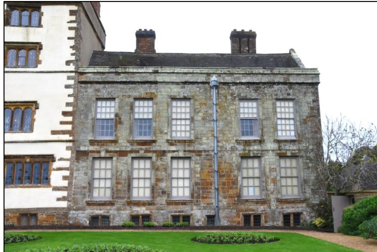
The eastern extent of the south elevation Fig 32
