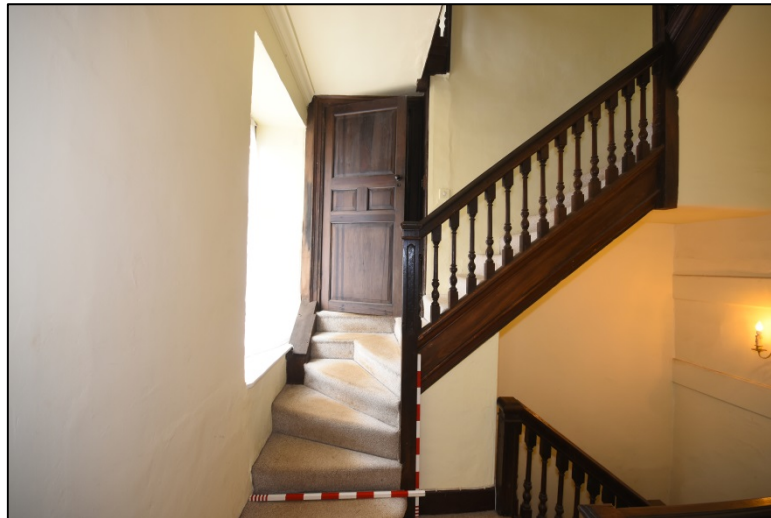
The stair to the second floor and Staff Room Fig 205
