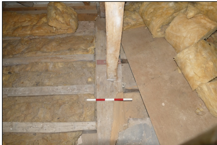
The truss, tie beam, and joist arrangement Fig 264
