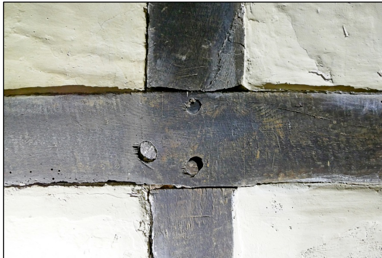
Detail of framing with faint assembly marks and scribe lines Fig 190
