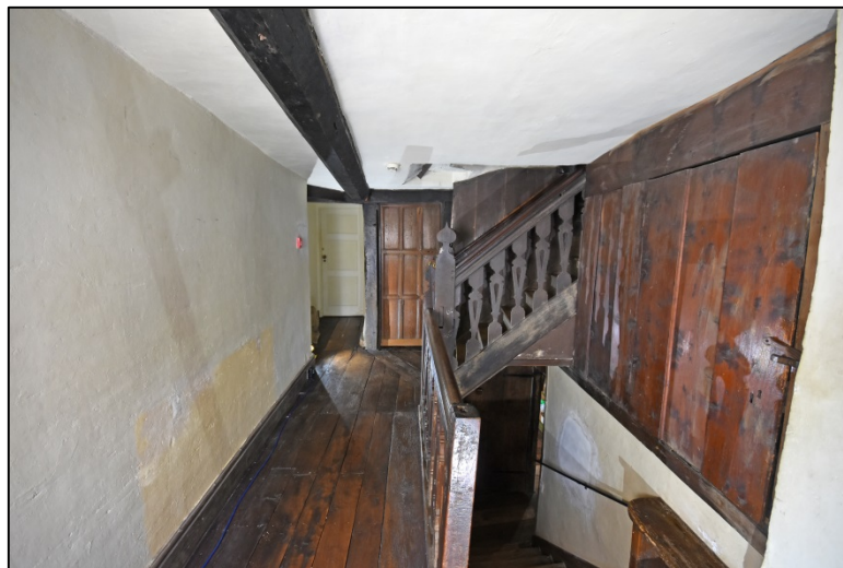
The mezzanine corridor, looking south Fig 191
