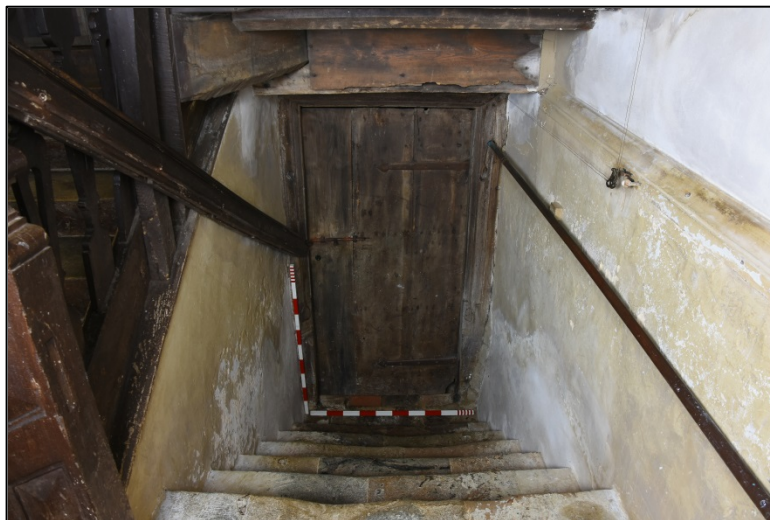
Steps down to the Cellar Fig 126
