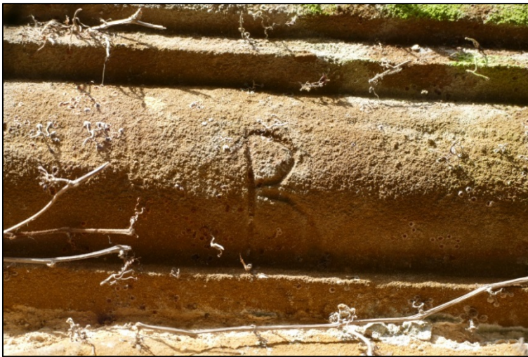
Detail of Masons mark on window lintel Fig 46
