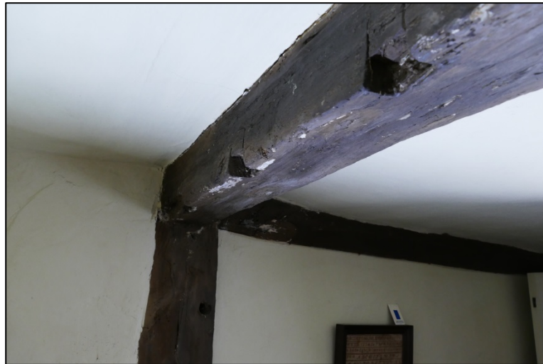
Defunct joist slots on the overhead beam Fig 199
