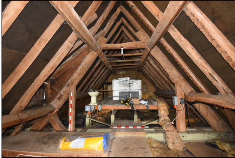
The north-west roof, looking east, showing Truss N5 Fig 259
