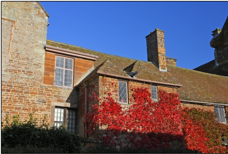
The privy and adjacent dormer Fig 43
