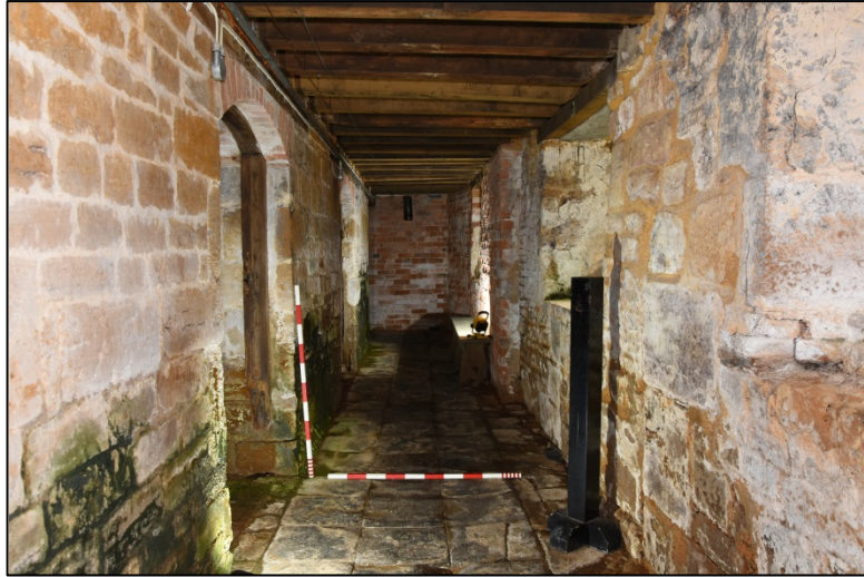
Corridor C8, looking north Fig 98
