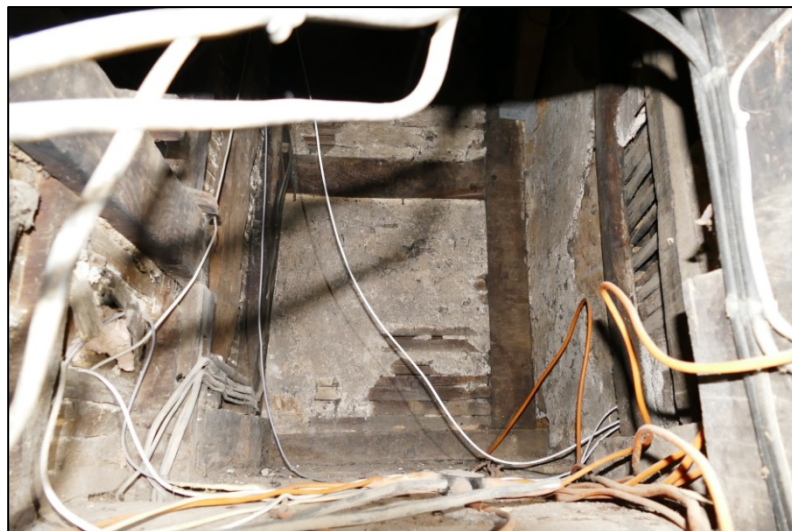
View into the void over the lobby Fig 146
