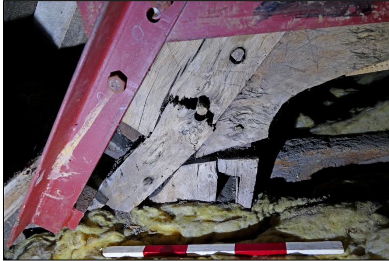
Detail of the lower north side of Truss N3 Fig 251
