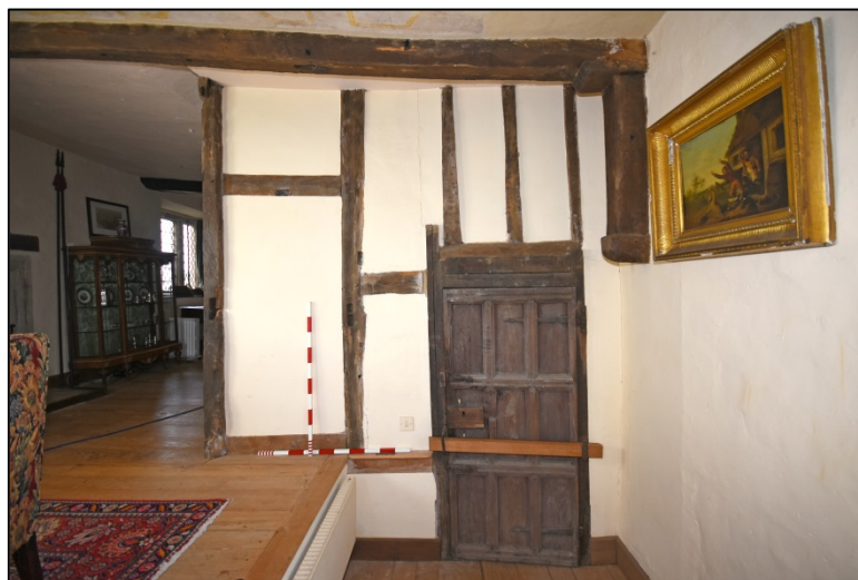
The stair partition and tie beam with bracket Fig 180
