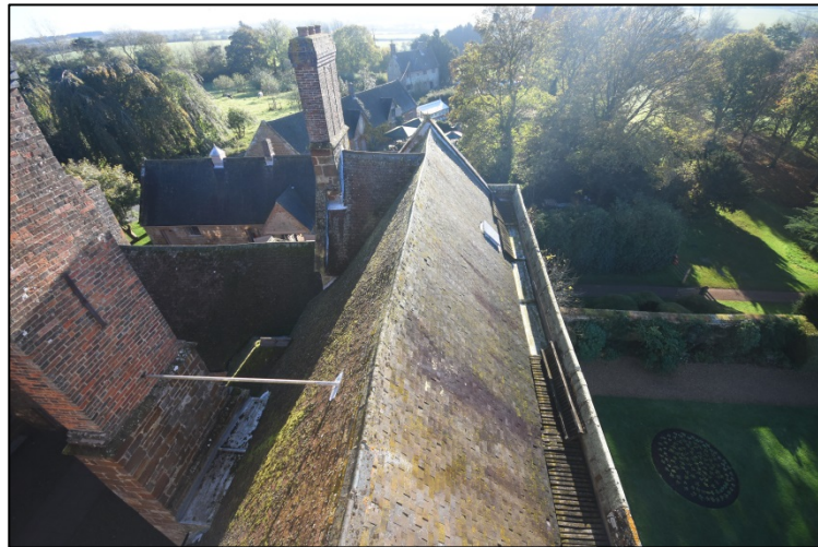
View of the south-east range from the Tower Fig 64
