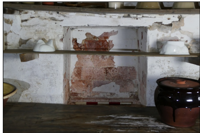
Blocked alcove in the east wall of the Larder Fig 103
