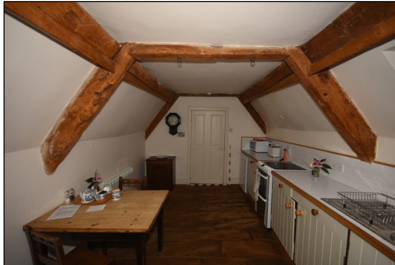
The Landmark Trust Kitchen, looking west, showing the two trusses Fig 273
