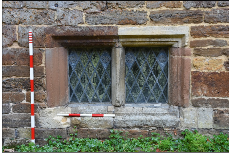
Inserted cellar window comprising of recycled framing members Fig 74
