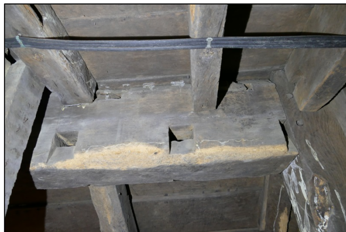
Re-used bridging beam with empty mortices Fig 215
