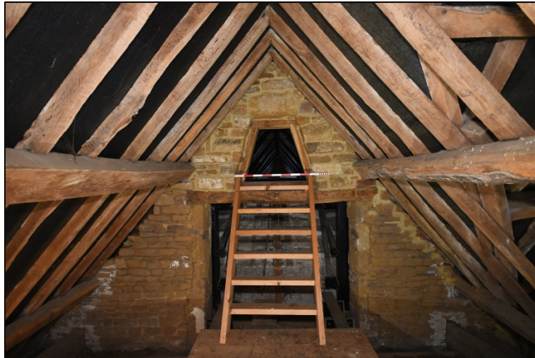
The stone gable over the Spenser's Room partition wall Fig 280
