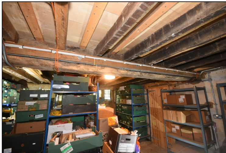
Room C2, looking south Fig 82
