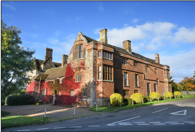
The north and east elevations, looking south-west Fig 38
