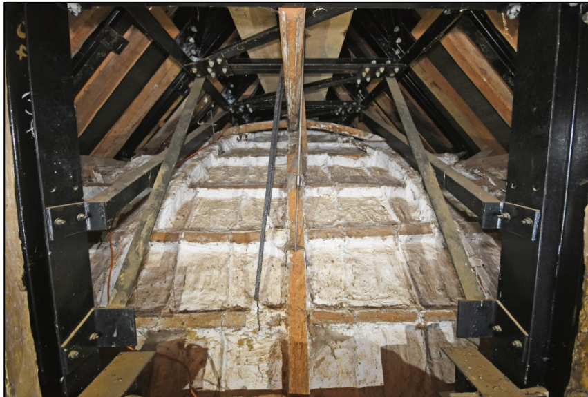
The Drawing Room ceiling frame, looking west Fig 277
