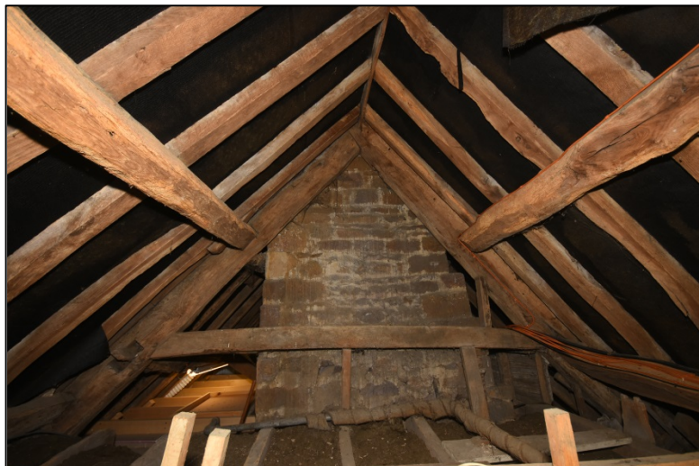
The upper part of Truss E4 Fig 240
