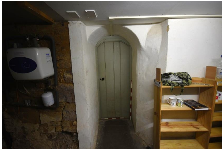
Inserted doorway between Rooms C1 and C2 Fig 81
