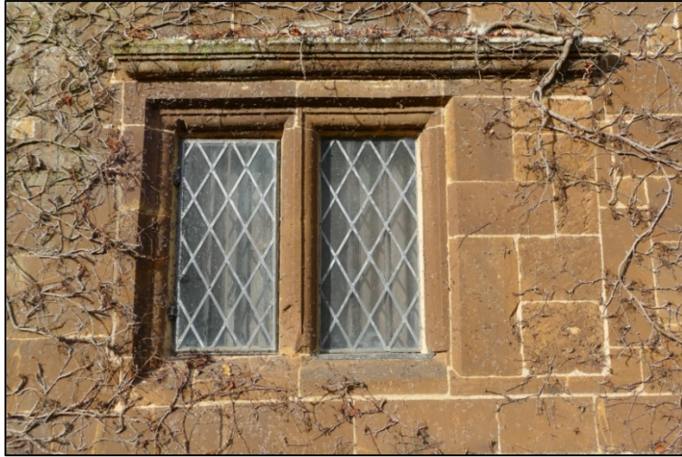
Mullion window with blocked light Fig 45
