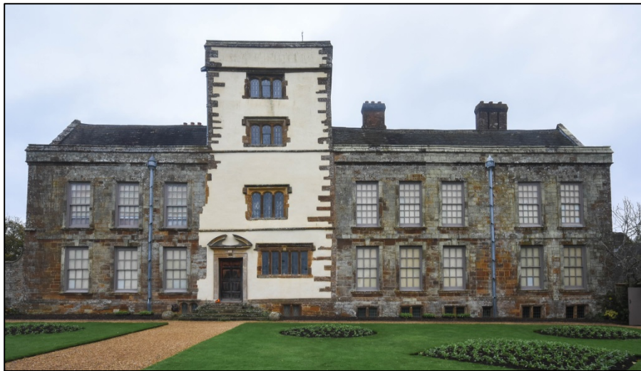
The south elevation, looking north Fig 30
