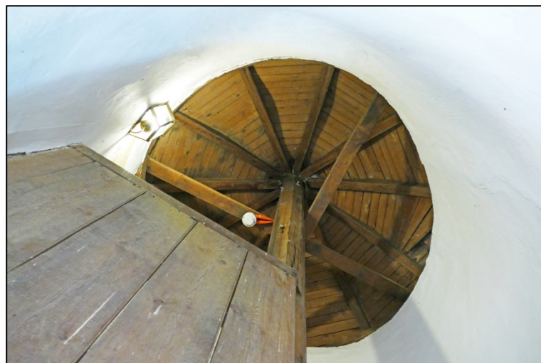
The underside of the tower roof Fig 219
