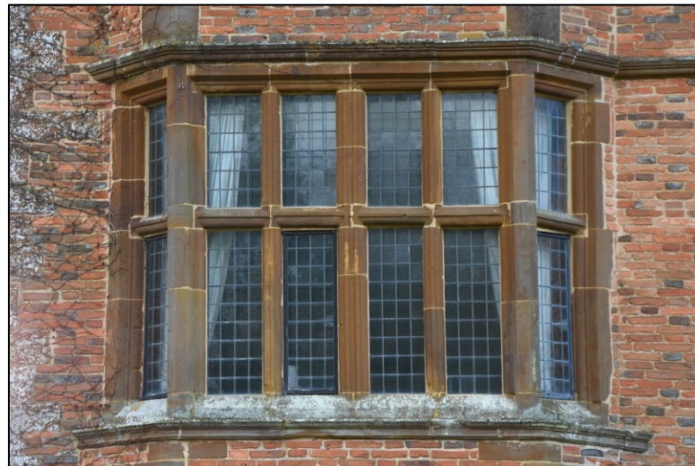
The lower eastern bay window Fig 11
