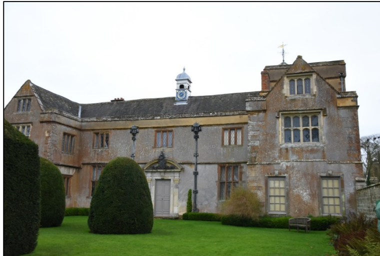
General view of the west elevation Fig 18
