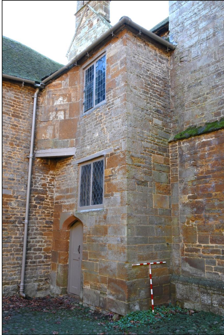
The stair turret; note blocked window and join to chimney Fig 66
