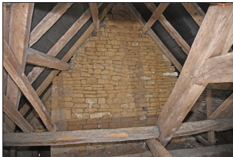
View of the south face of the gable and chimney Fig 282
