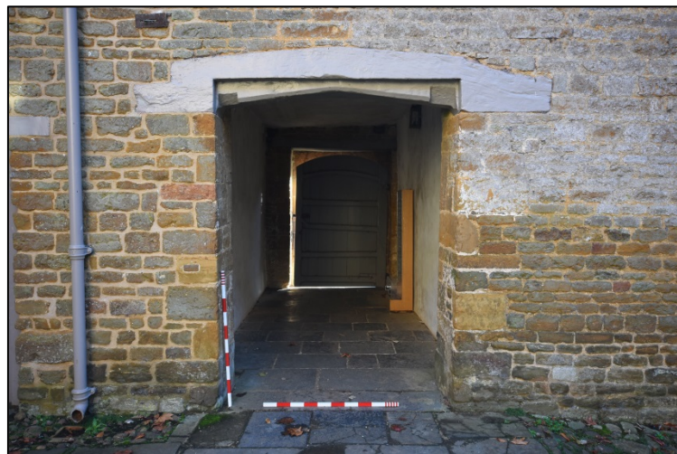
The passageway and lintel Fig 59
