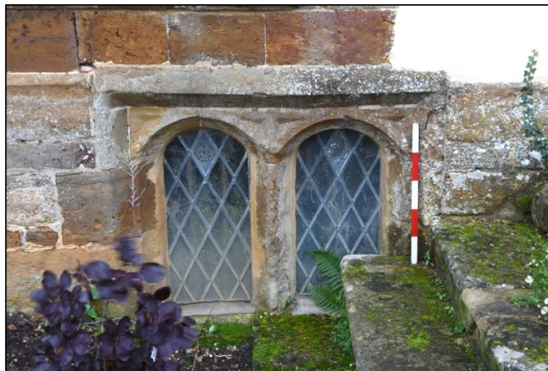
Cavetto mullion cellar window Fig 33
