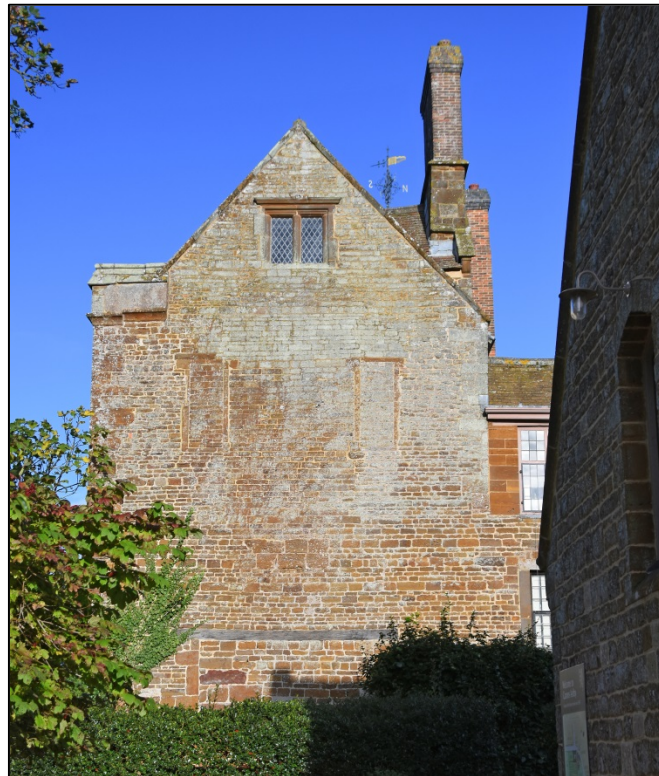
The south gable showing blocked bay window and oriel Fig 41
