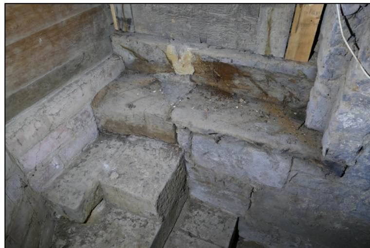
The stone stair in the cellar Fig 211
