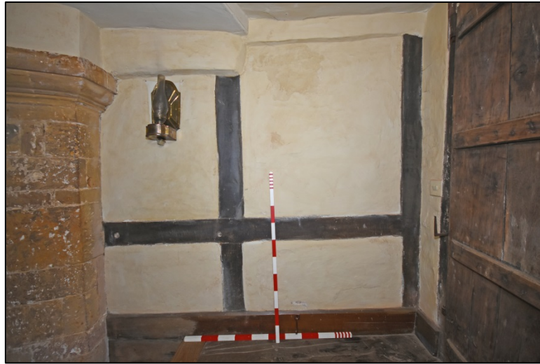
Part of the timber-frame bay adjacent to the Kitchen Fig 189
