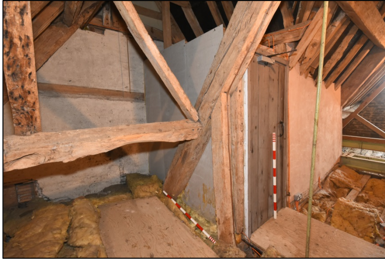
The attic stairwell Fig 262
