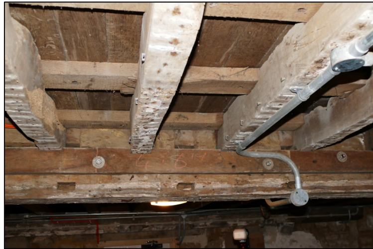
Detail of bridging beam, showing defunct mortice arrangement Fig 90
