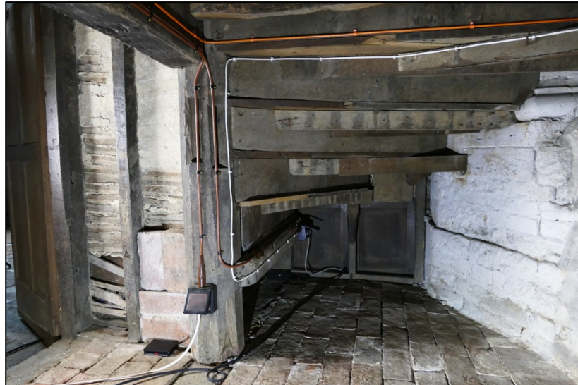
The under-stair space, looking east Fig 186
