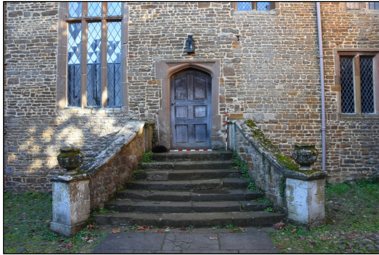
Doorway and steps. Note changes in fabric around the doorway Fig 77
