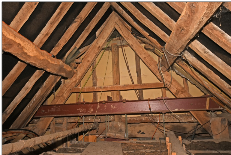
Truss E6, the join between the east and north ranges Fig 243
