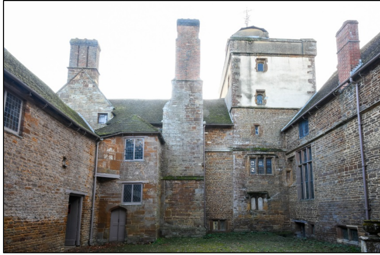
The southern courtyard elevation Fig 63
