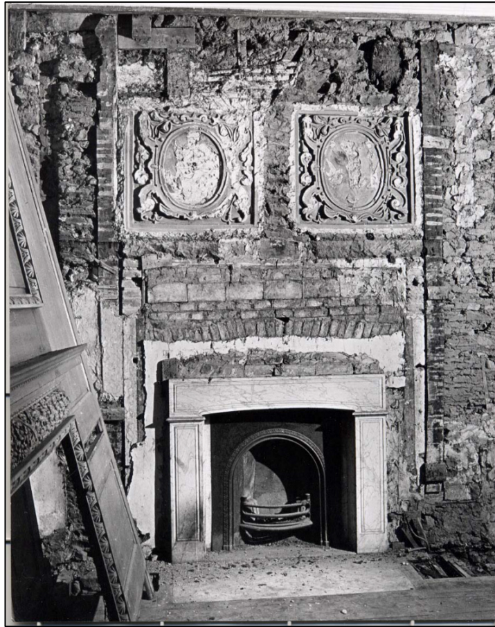
View of the north wall during conservation, with panelling removed Fig 161
