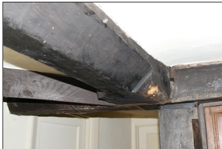
Detail of the beam arrangement adjacent to the mezzanine rooms Fig 200
