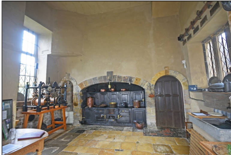
The eastern half of the Kitchen Fig 128
