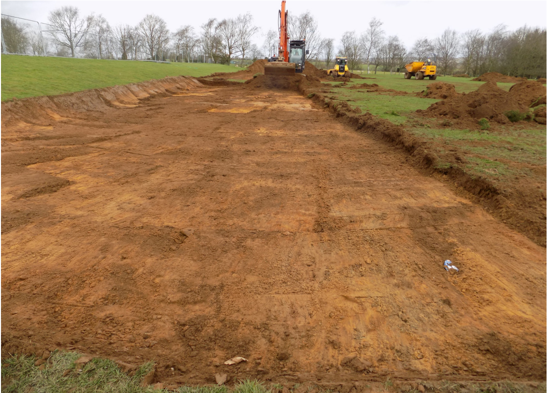
Stripping area for tennis courts, looking north
