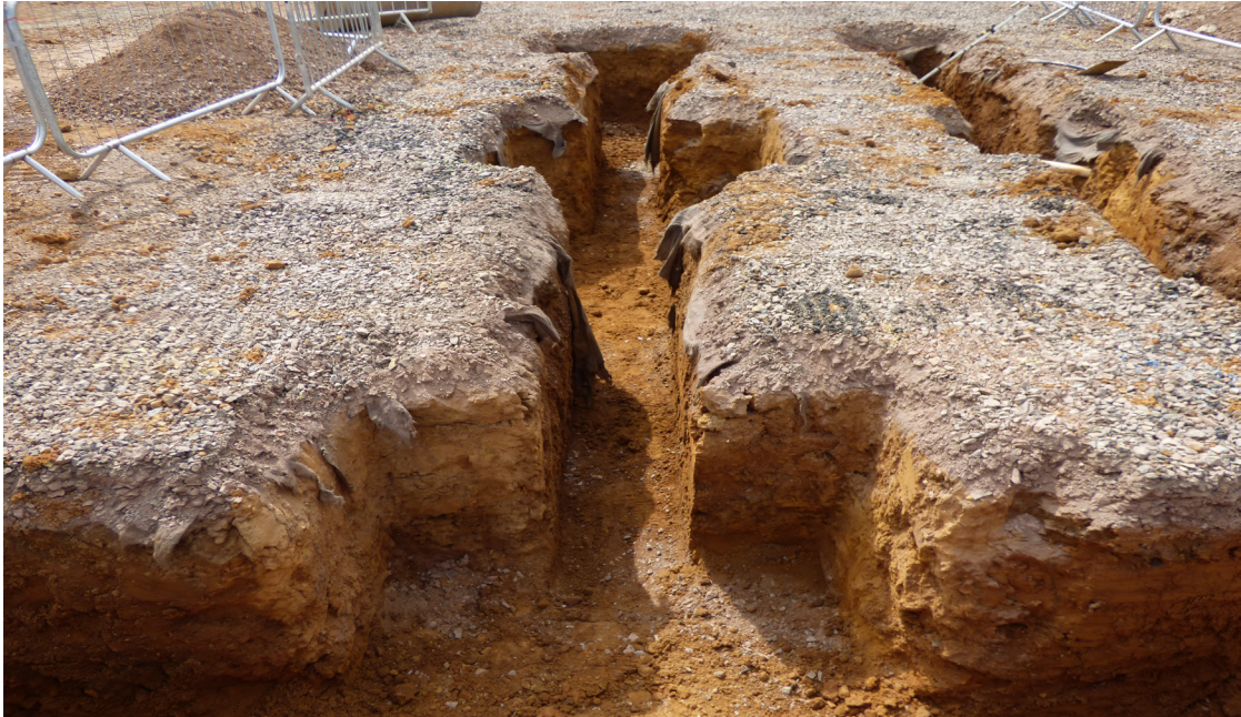
Changing rooms footings
