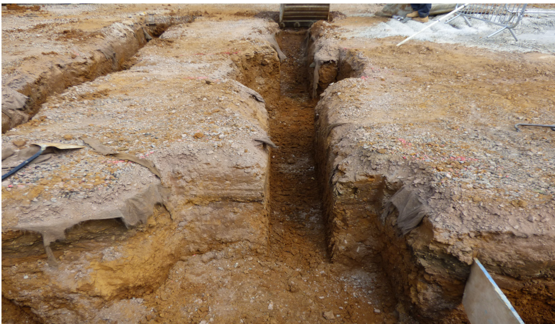
Changing rooms footings
