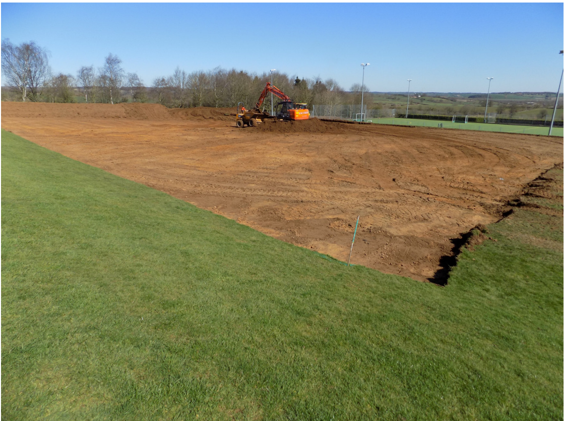
Area stripped for tennis courts, looking north-east
