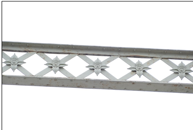
Detail of the girder rosettes Fig 21
