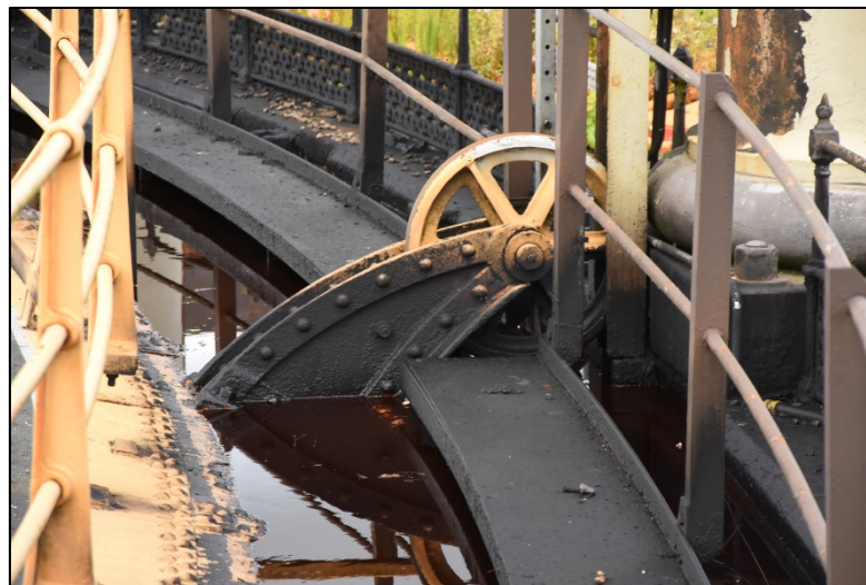
Example of the roller carriages Fig 24
