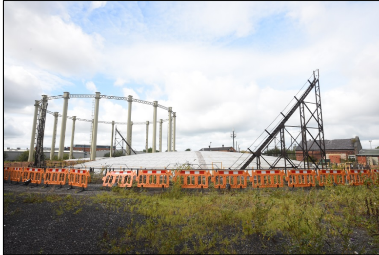
Gasholder 1, looking north-west Fig 9
