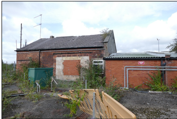
The Governor House and electrical switch room, looking north Fig 30
