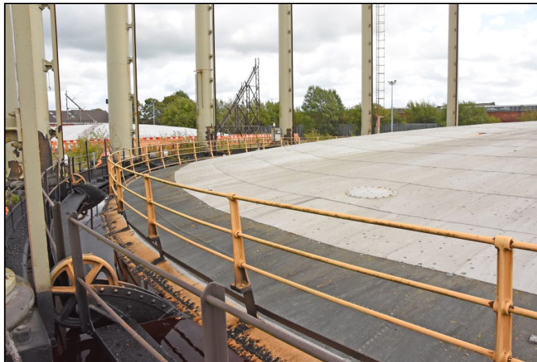
The crown top curb, also showing manhole access, looking south-east Fig 27
