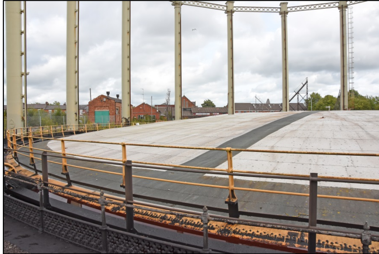
General view of the gasholder crown, looking north-east Fig 26
