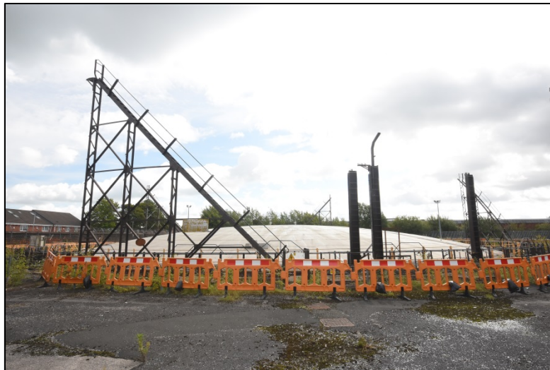
Gasholder 1, looking south-east Fig 10
