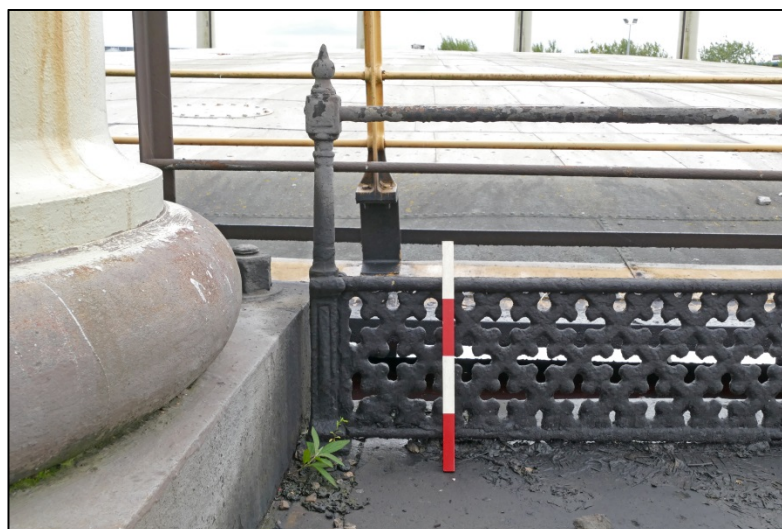
Detail of the decorative railings Fig 25
