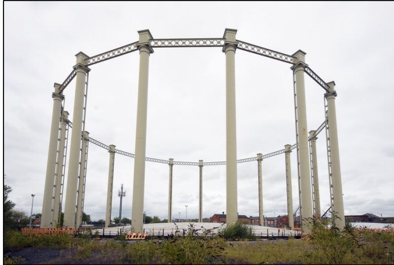
Gasholder 2, looking north Fig 18
