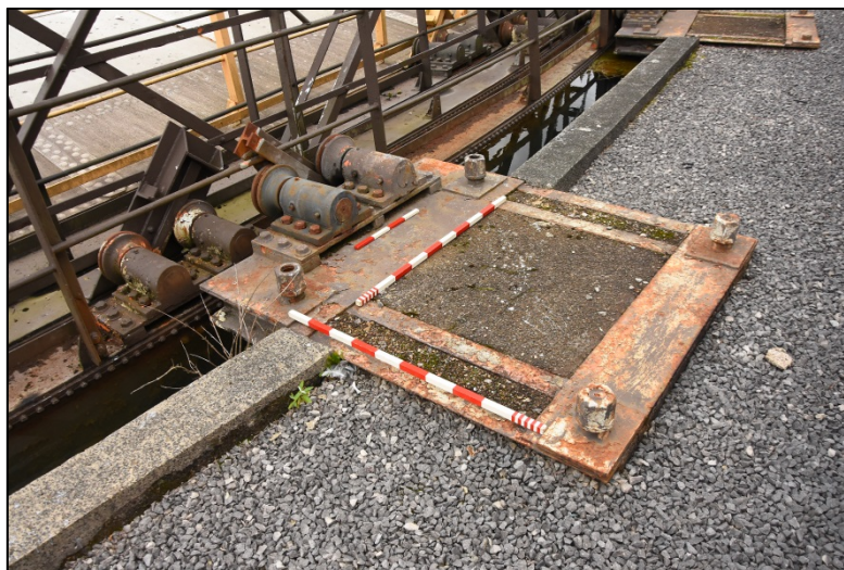
Example of the outer roller carriages Fig 14
