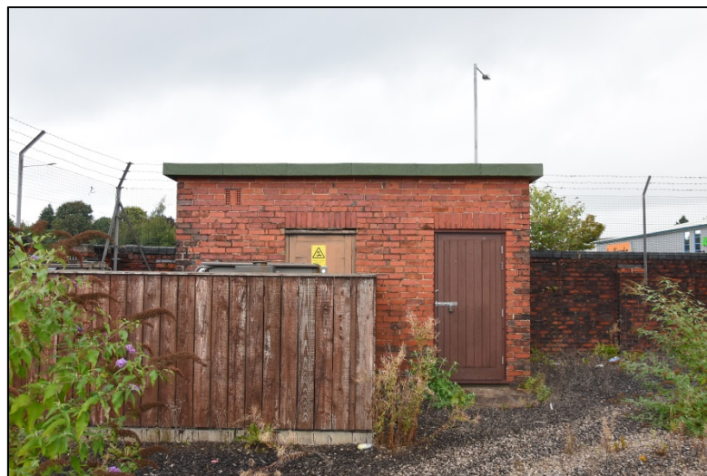
The Meter House / Substation Fig 36
