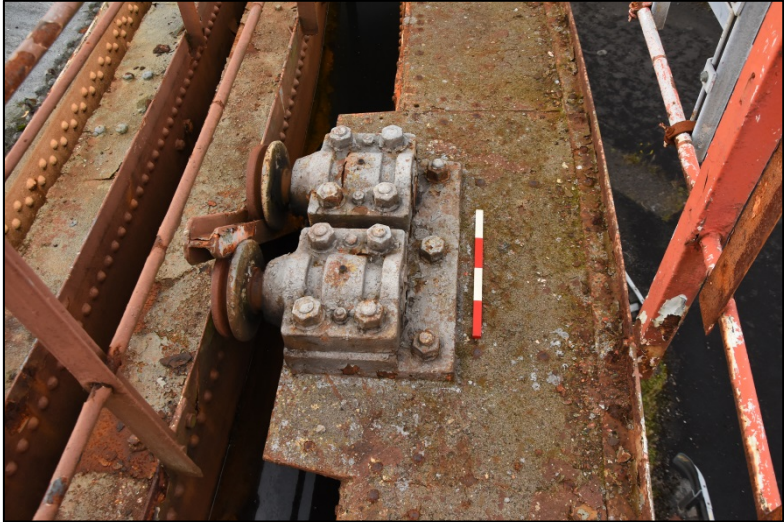
Example of the outer roller carriages Fig 29
