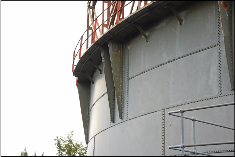
The walkway supports Fig 21
