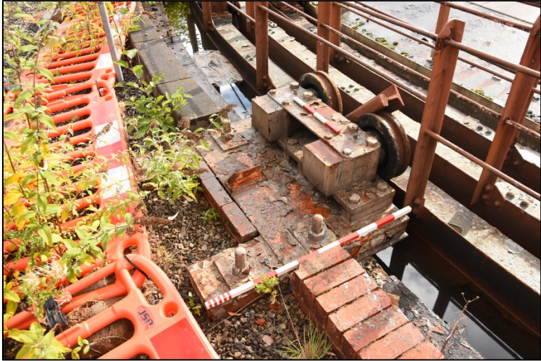
Example of the outer roller carriages Fig 11
