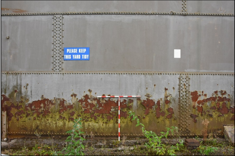
Detail of the tank construction Fig 20
