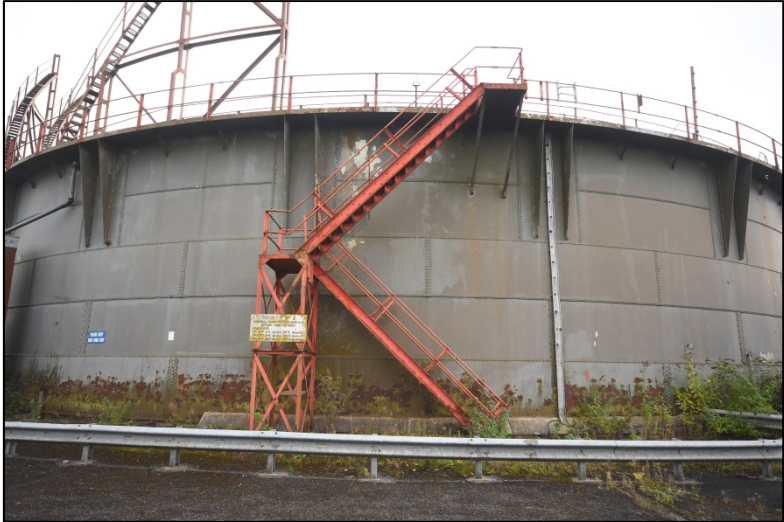
The tank stairs Fig 22
