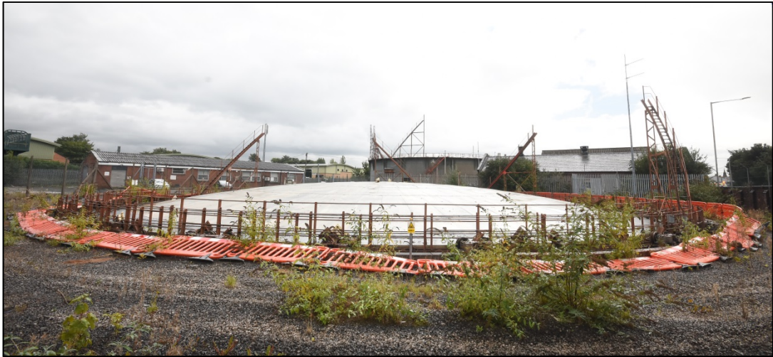
General view of Gasholder 1, looking south-east Fig 9
