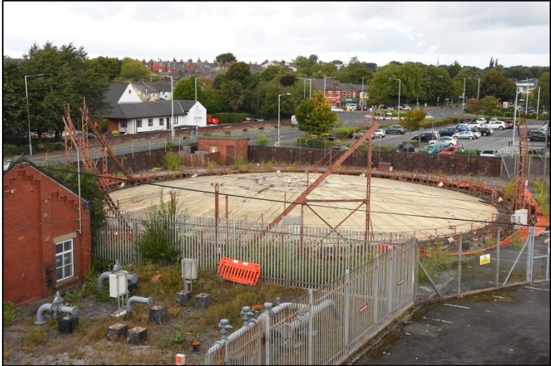
View of Gasholder 1, looking north-west Fig 8
