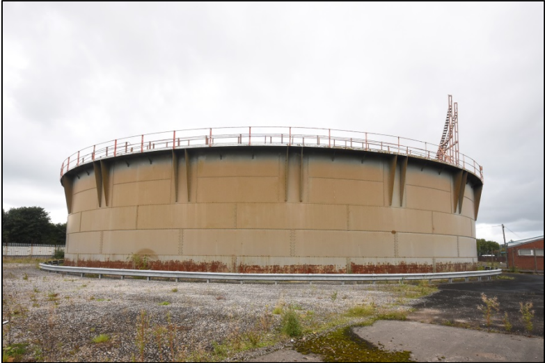
Gas holder 2, looking north-west Fig 19
