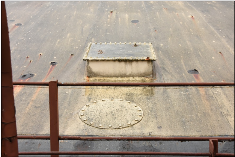
Circular and raised square manholes at the south side of the crown Fig 14
