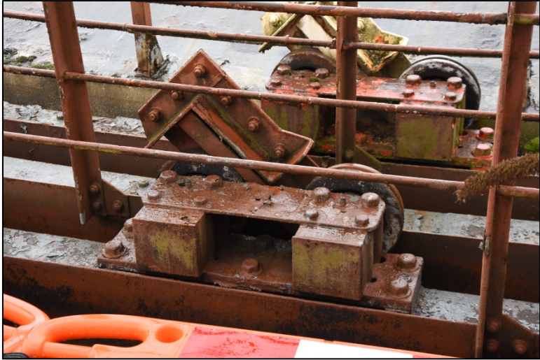
Example of the lift roller carriages, note run-out stops Fig 12
