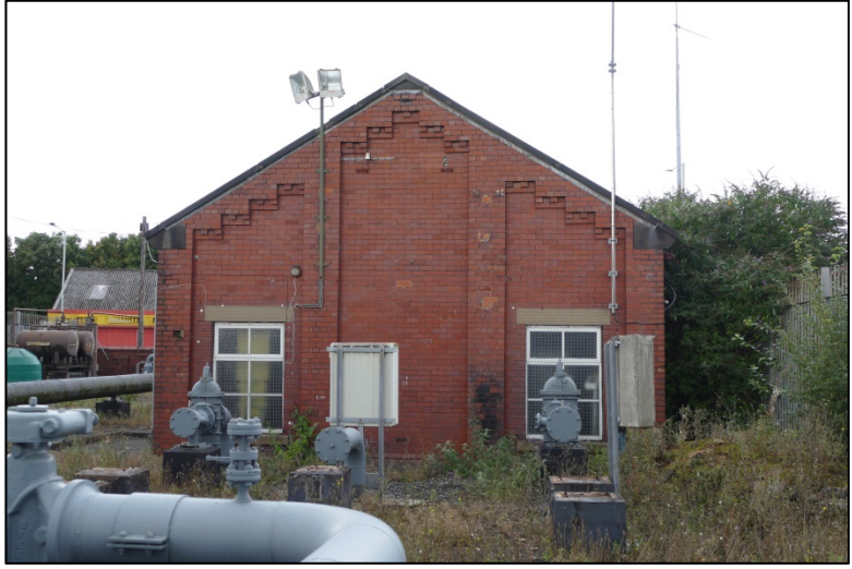
The east elevation Fig 33
