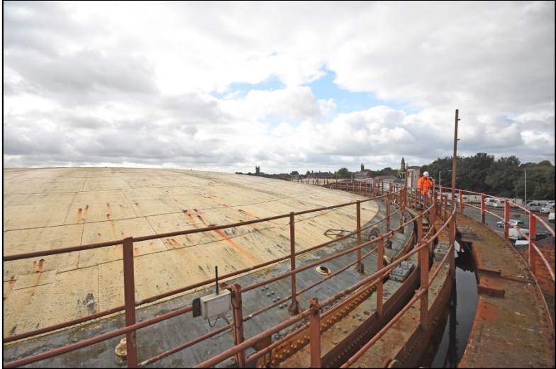
General view of the lift grips and crown, looking south-west Fig 26
