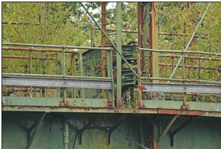
Example of the roller carriage sets Fig 12
