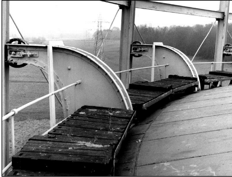
View of the roller carriages (undated photograph NGA Ref: XG01090) Fig 13
