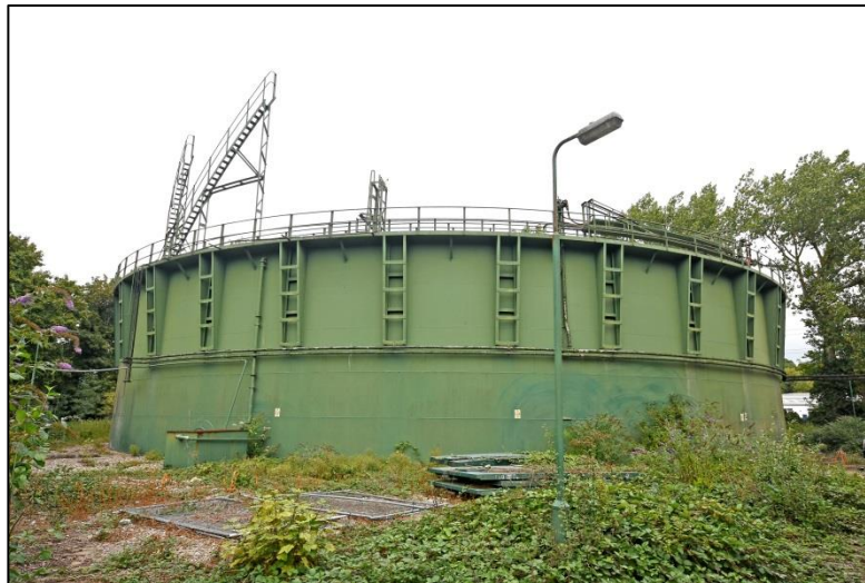
General view of Gasholder 2, looking north-west Fig 20
