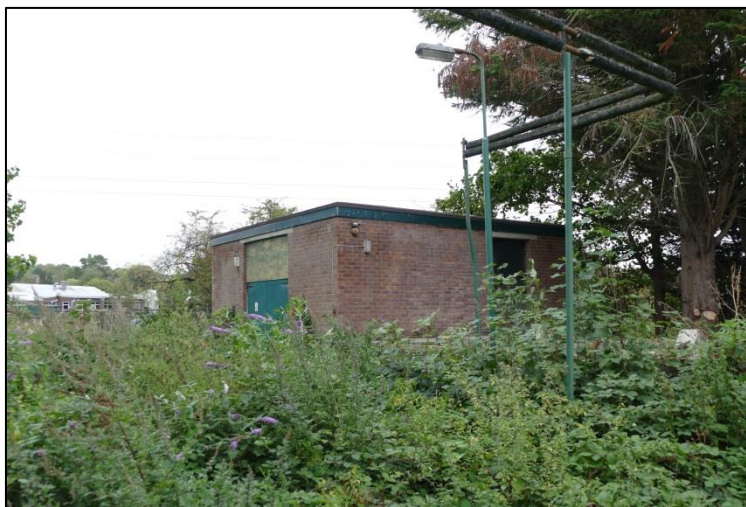
The former Boiler House, looking north-east Fig 29
