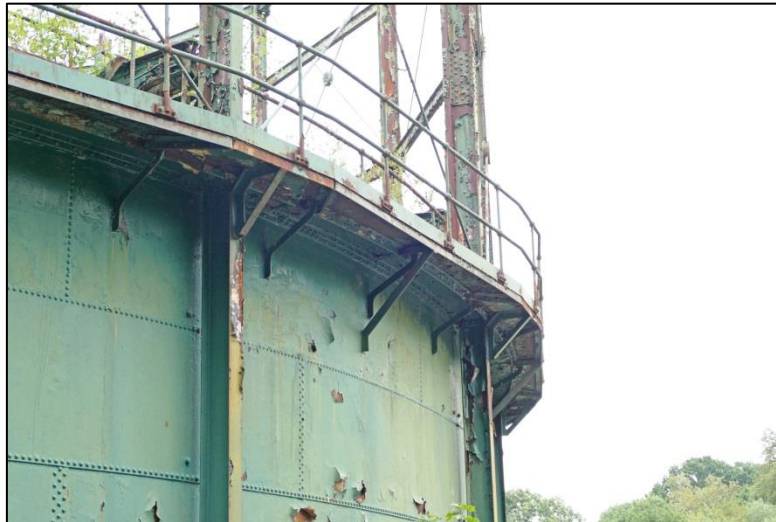
The underside of the tank walkway, showing brackets and bracing Fig 11
