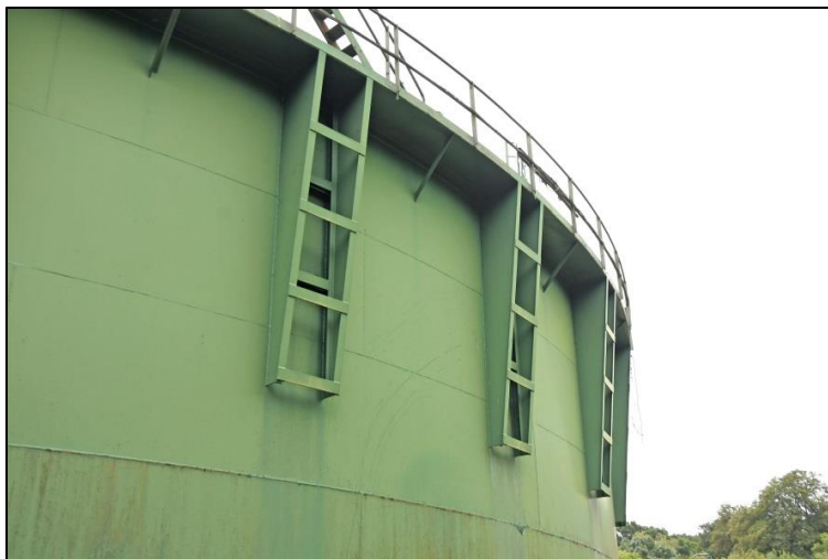
The walkway and supporting brackets Fig 24
