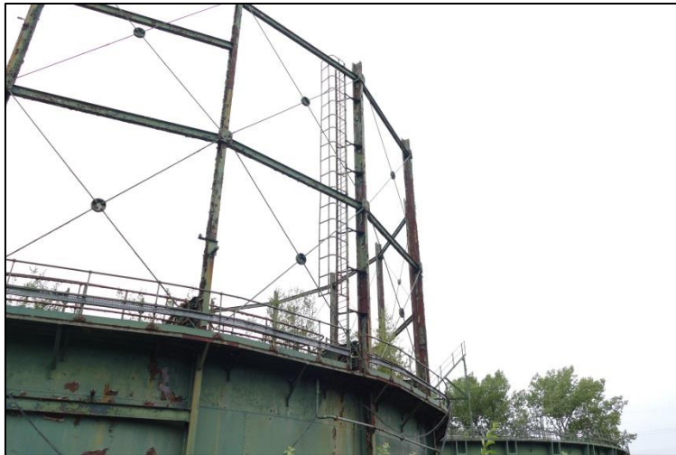
General view of the framing Fig 14
