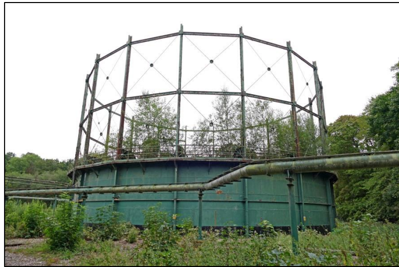
General view of Gasholder 1, looking south Fig 8
