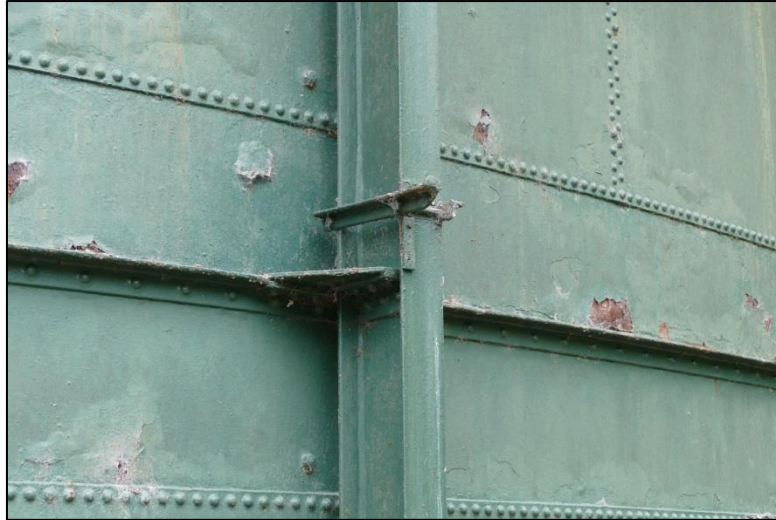
Detail of the standard and mid-tank collar Fig 10
