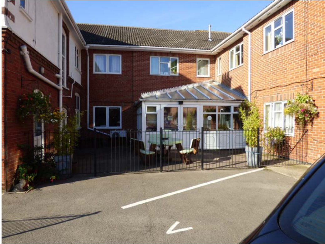
The conservatory to be replaced by single-storey flat-roof extension, looking north Fig 4
