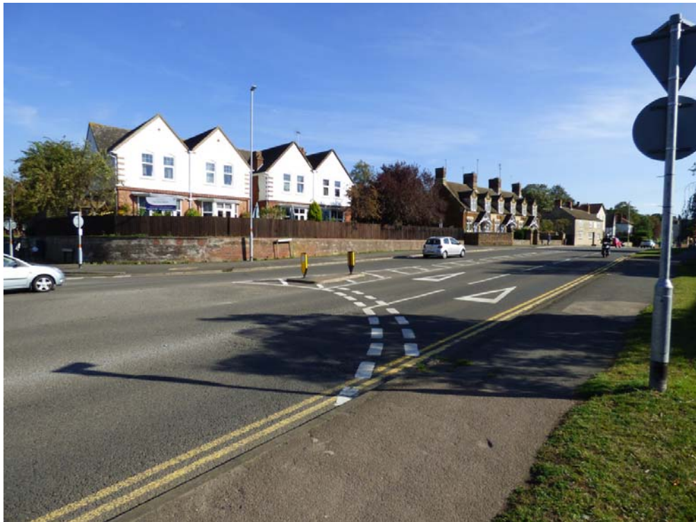
View of The Shrubbery and almshouses, looking south-east into the conservation area Fig 20
