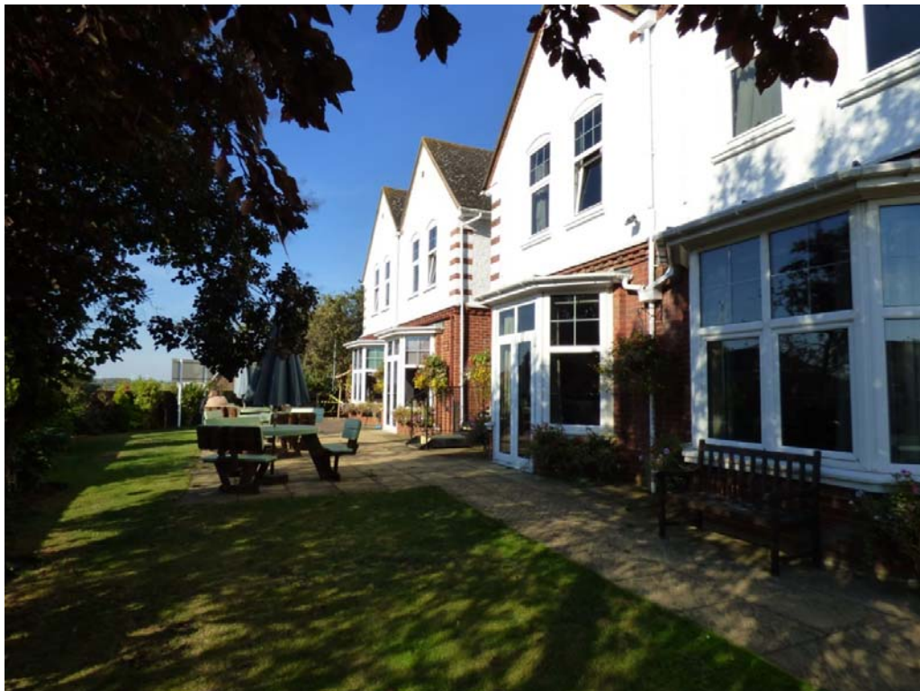
Western elevation of The Shrubbery, looking north, the northern section to be extended west Fig 3
