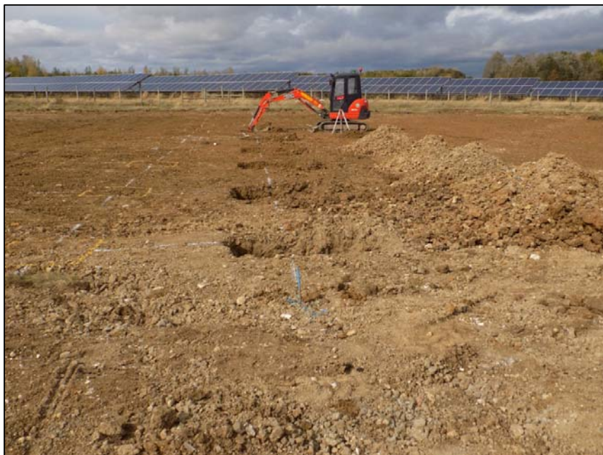
View of pits undergoing excavation, looking south-east Fig 4
