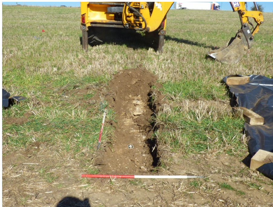
Soakaway 28, general view, looking north
