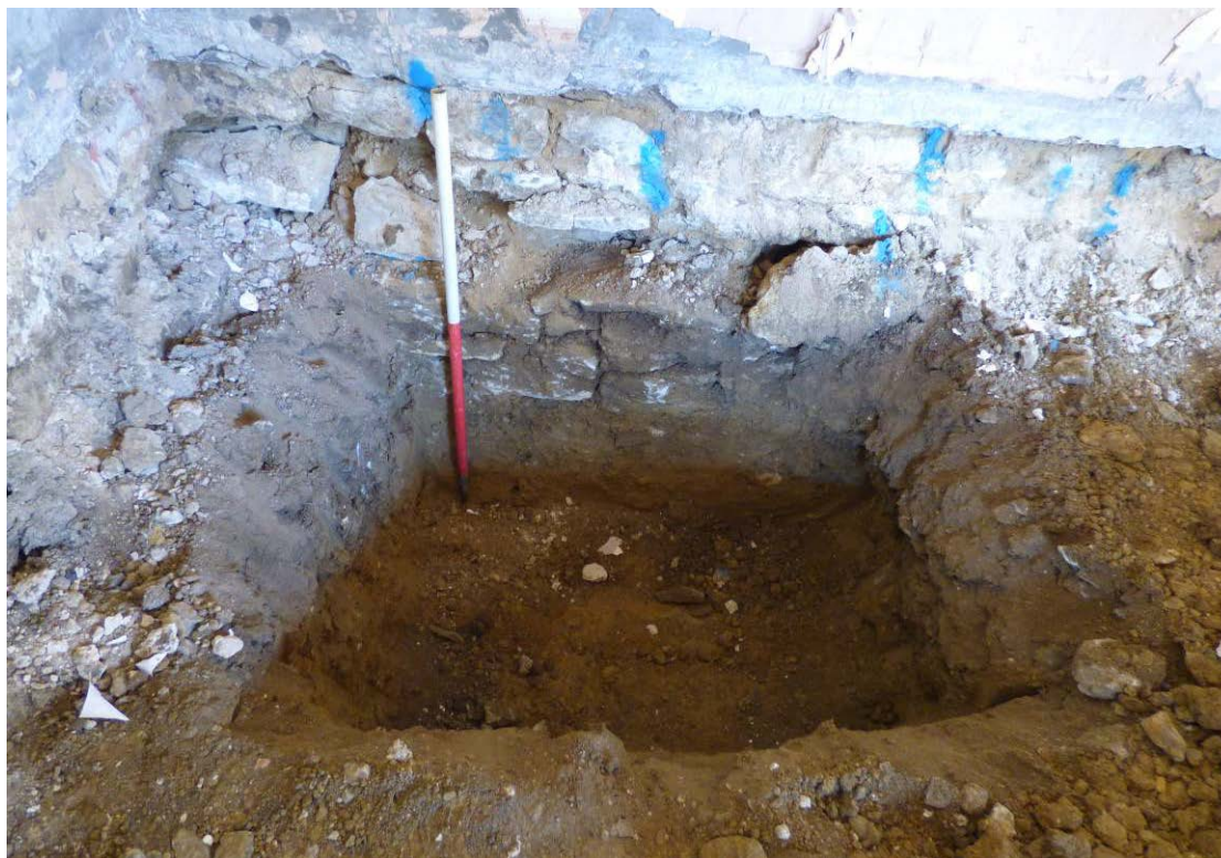
Underpinning pit 1 (plot 1), looking north Fig 4
