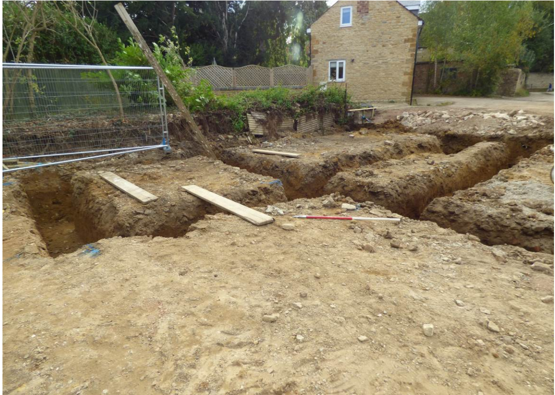
Plot 5 foundation trenches, looking south-west Fig 2
