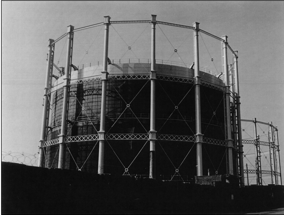
Gasholder 4, photograph c1983 (Manchester Archive ref 665-7) Fig 7
