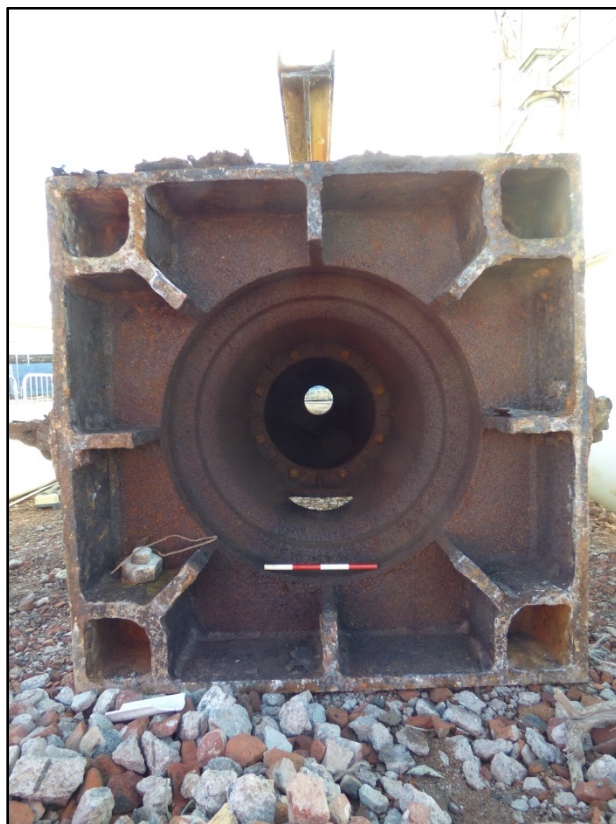
Underneath the base of the column Fig 29
