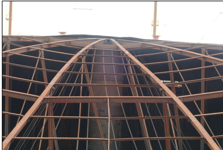
The central pipe with primary rafters and tie bars Fig 48
