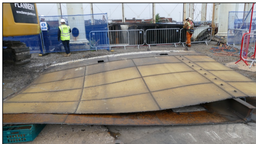
Example of the removed lift sheets Fig 25
