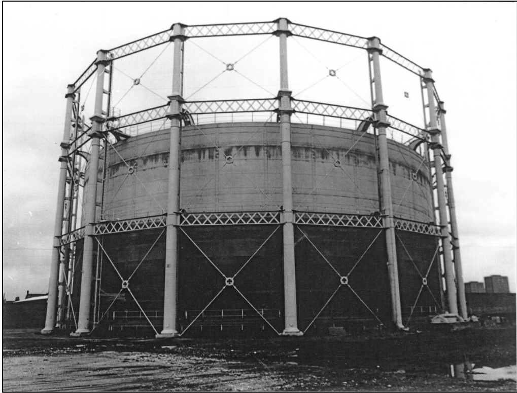
Gasholder 3, photograph c1988; note lattice girders at the upper level (Manchester Archives ref 725-4) Fig 6
