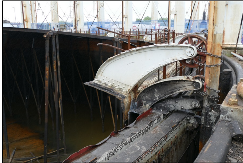
View of the roller carriages and section of the top curb Fig 17
