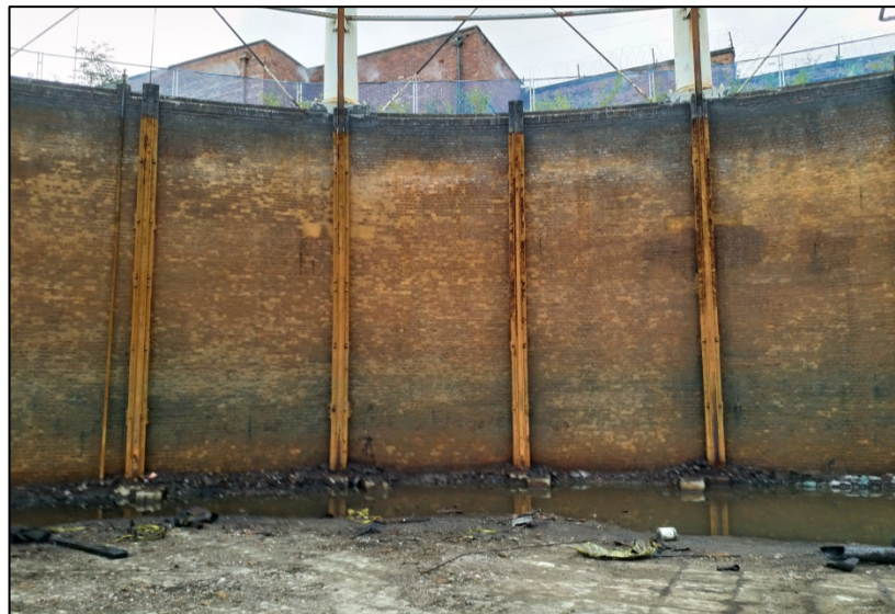
View of the brick tank and guide rails Fig 24
