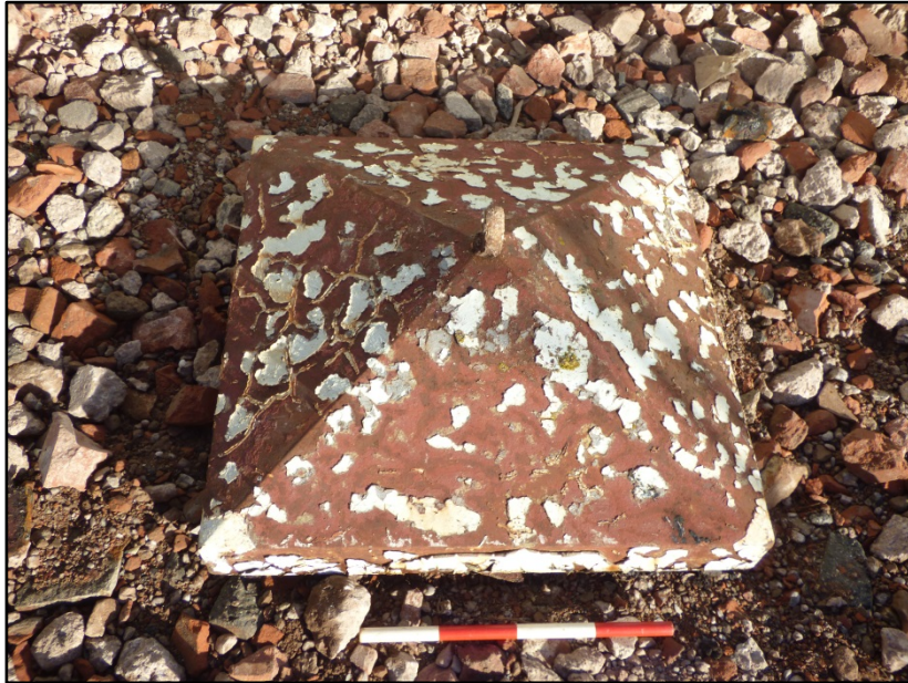
Cap on top of columns Fig 26
