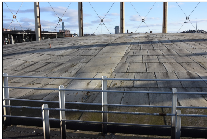
View of the crown with walkway Fig 41
