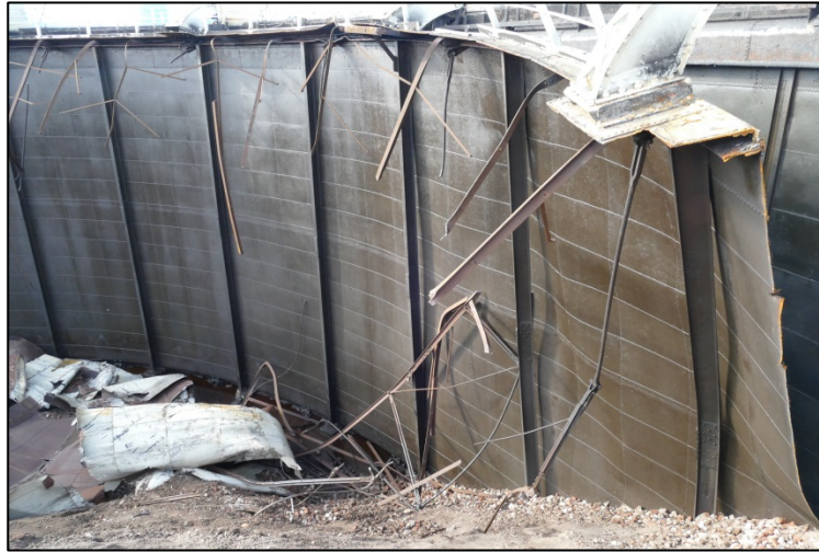
View of the lift sheeting with vertical stiffeners Fig 50
