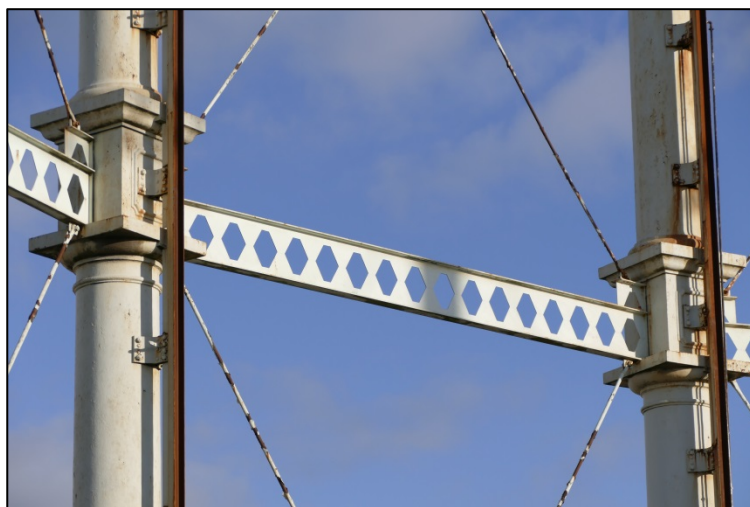
The castellated girders, also showing the roller guide channels Fig 35
