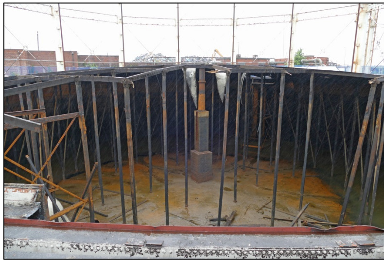
The exposed timber crown support, looking south-east Fig 21
