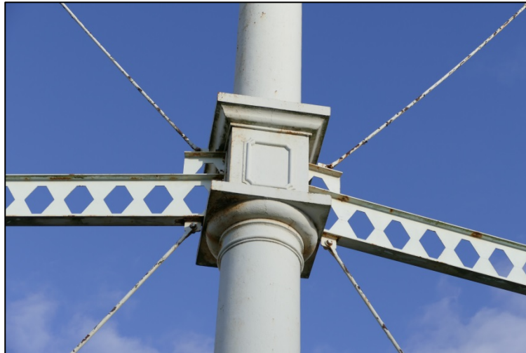
Example of the first-tier entablature boxes; note the stacked girders Fig 34
