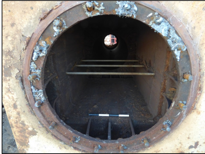
Joint of column with internal bars Fig 56
