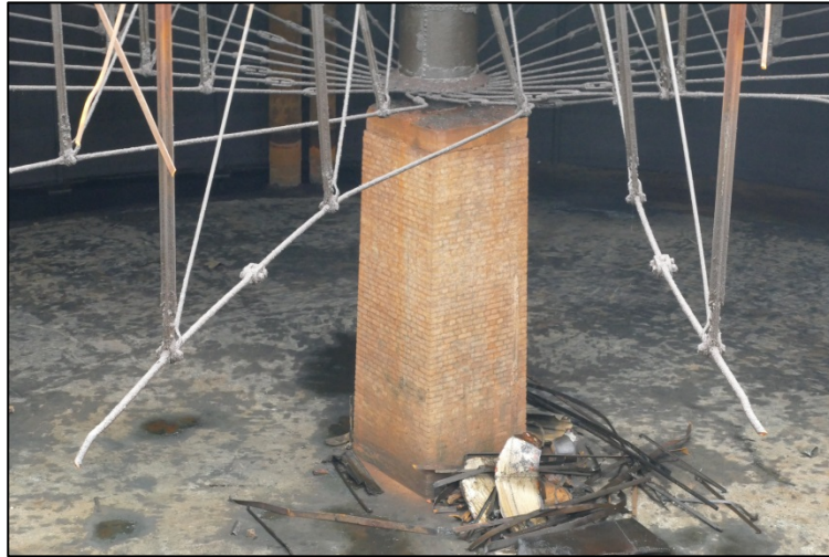
Detail of the brick stanchion Fig 47
