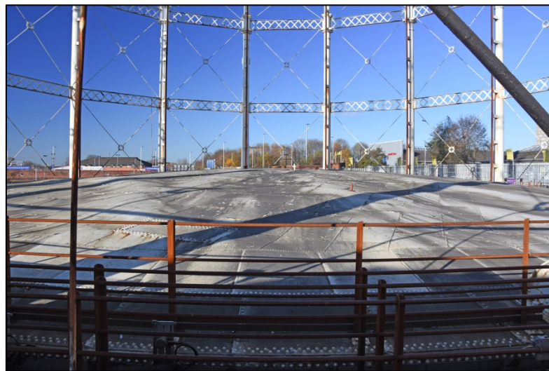
General view of the crown, looking north-west Fig 18
