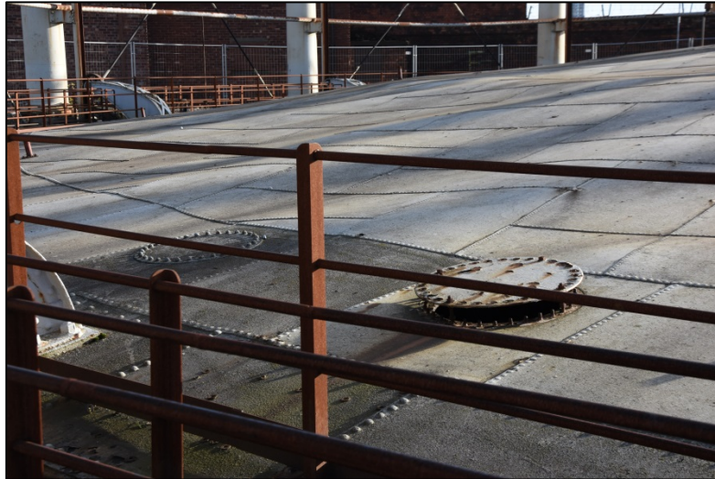
Manholes at the north-west side of the crown Fig 20
