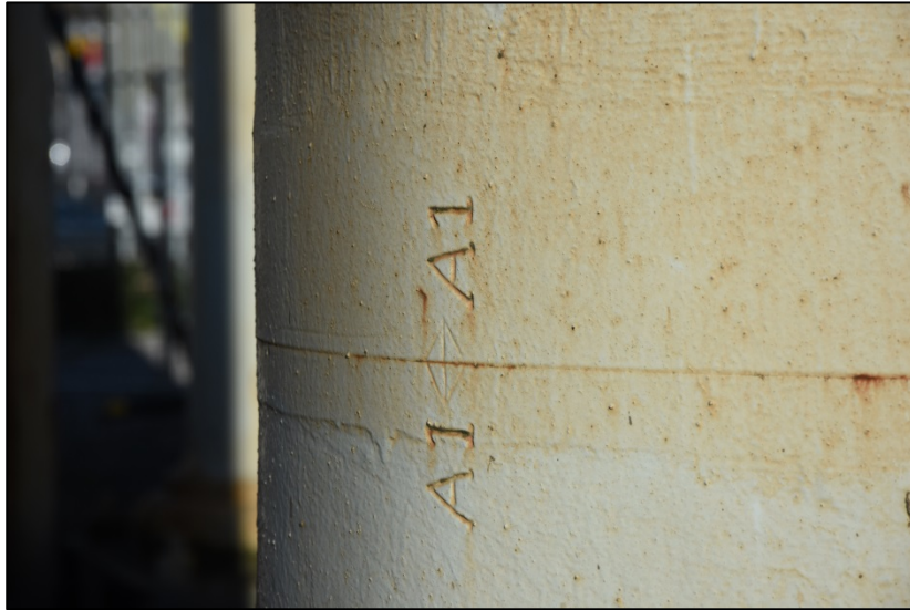
Detail of assembly marks on the column drums (column 14) Fig 11
