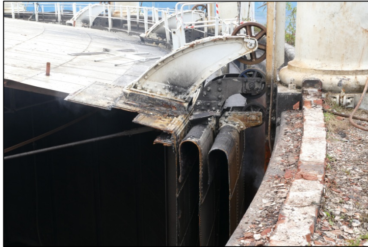
Example of the roller carriage sets, also showing cross-section of the lifts and pressed-plate grips Fig 39
