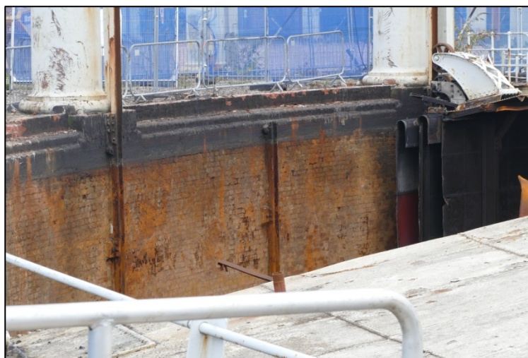
View of the tank brickwork and kerb Fig 52
