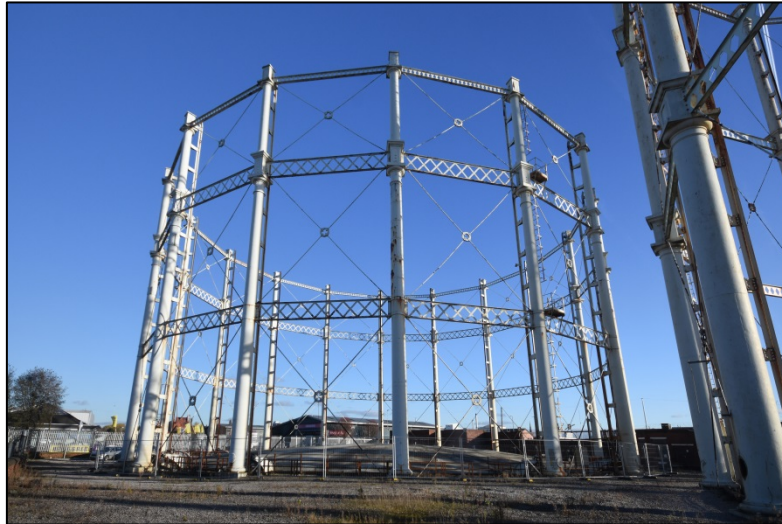
General view of Gasholder 3, looking north-east Fig 8
