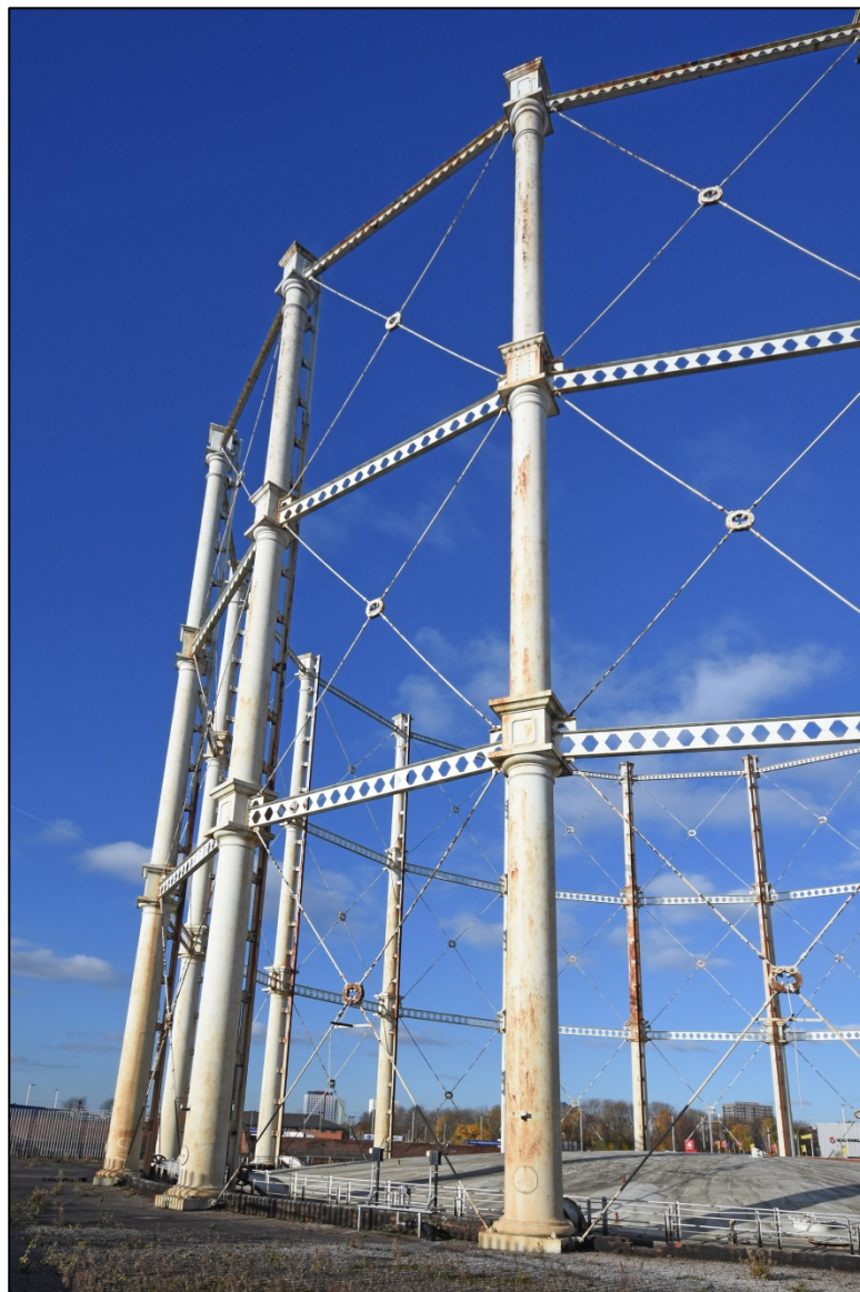
Example of the Gasholder 4 columns Fig 32
