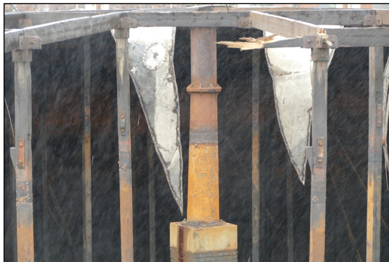
Detail of the central support Fig 22
