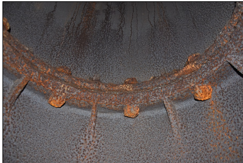
Internal view of column footing flanged joint Fig 12
