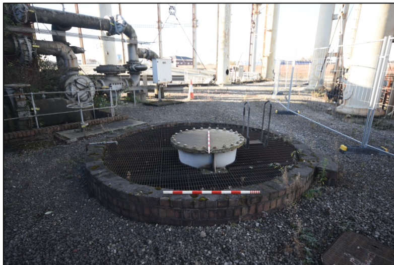
Gasholder 3 dry well Fig 54
