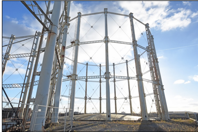
General view of Gasholder 4, looking north-east Fig 31
