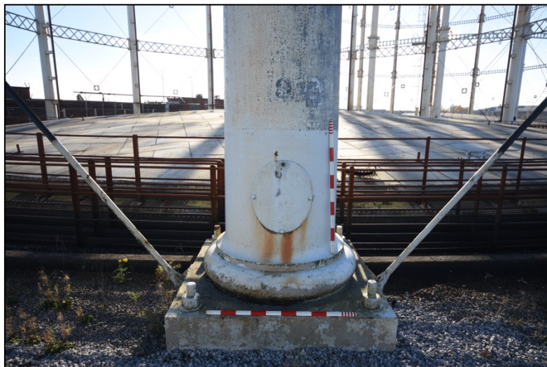
Example of the Gasholder 3 column bases (column 9) Fig 10
