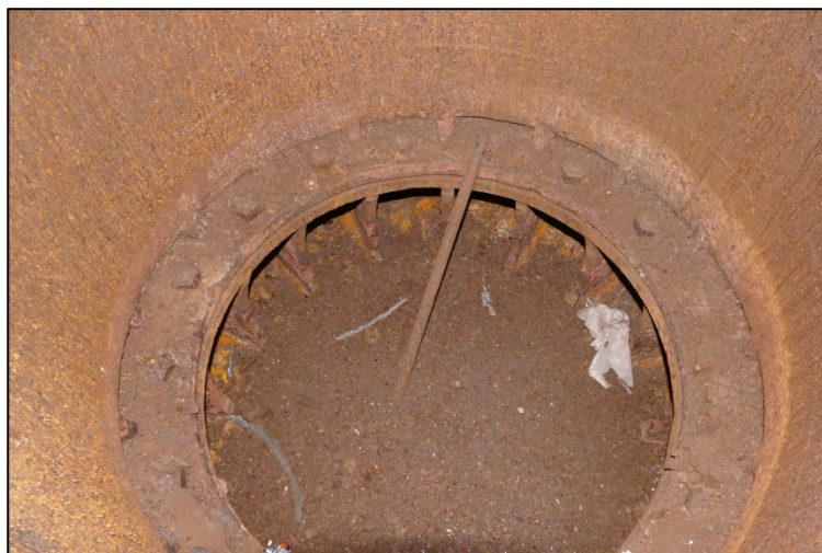
View of the internally flanged column / footing joins Fig 38
