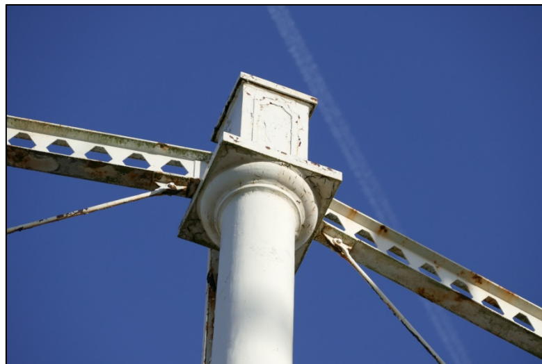
Example of the topmost entablature boxes and girders Fig 13
