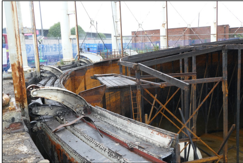
The crown support, looking east; note elevated platform Fig 23
