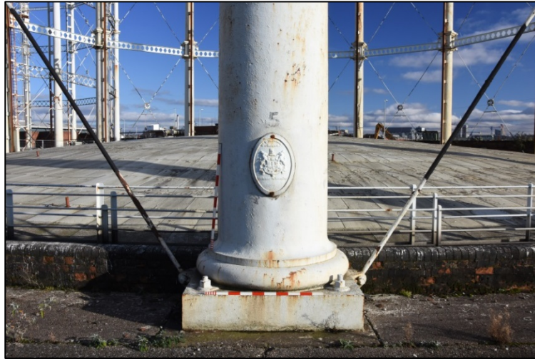
Example of the column footings with commemorative plaque Fig 36
