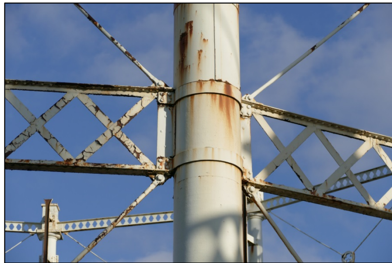
Example of the first tier girder collars Fig 15
