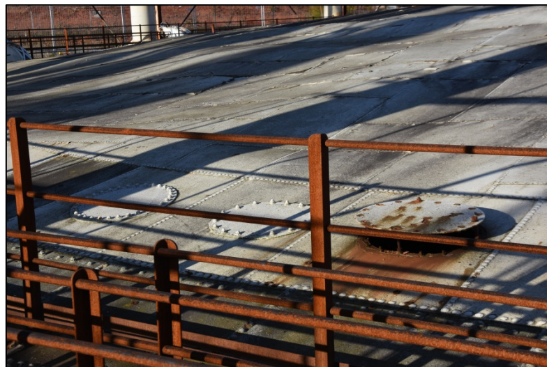
Manholes over inlet and outlet pipes at the south-east side of the crown Fig 19
