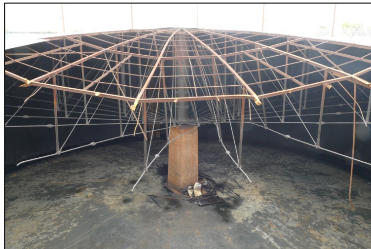
View of the crown frame and central stanchion Fig 46
