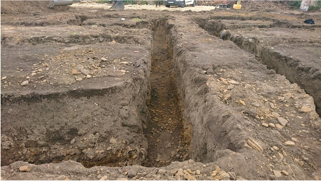
Foundation trenches, plots 1–2, looking east Fig 5
