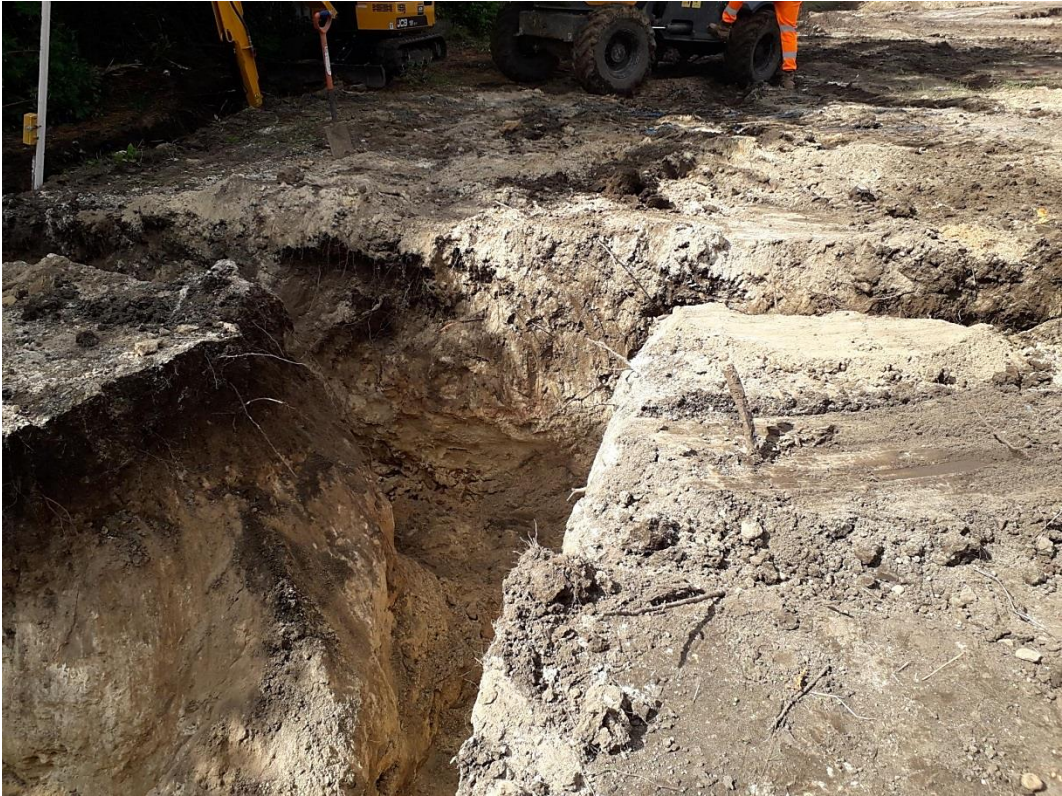
Foundation trench, plot 2, looking south Fig 7
