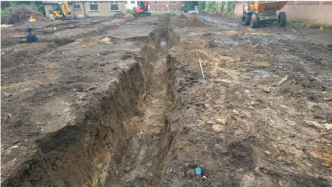
Foundation trenches, plots 1–2, looking south Fig 4
