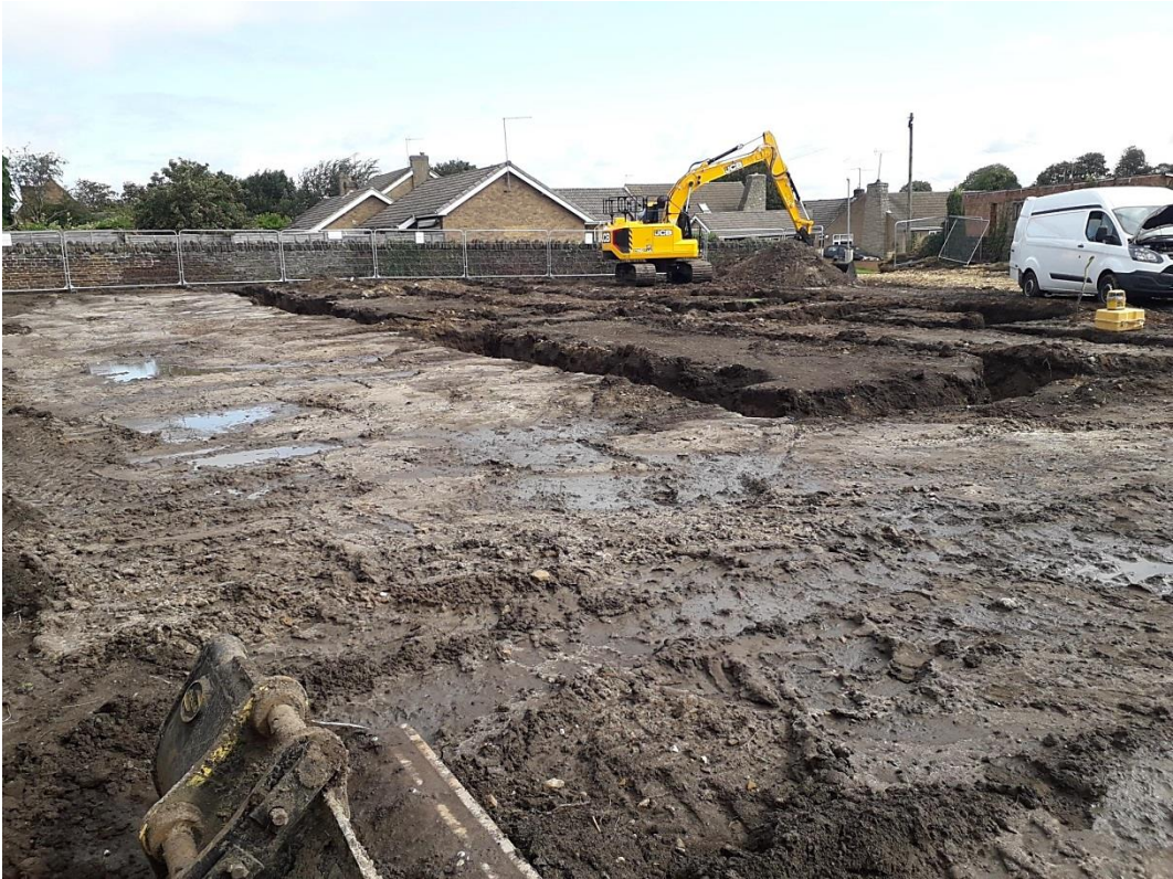
Partial topsoil and subsoil strip, looking north-east Fig 3
