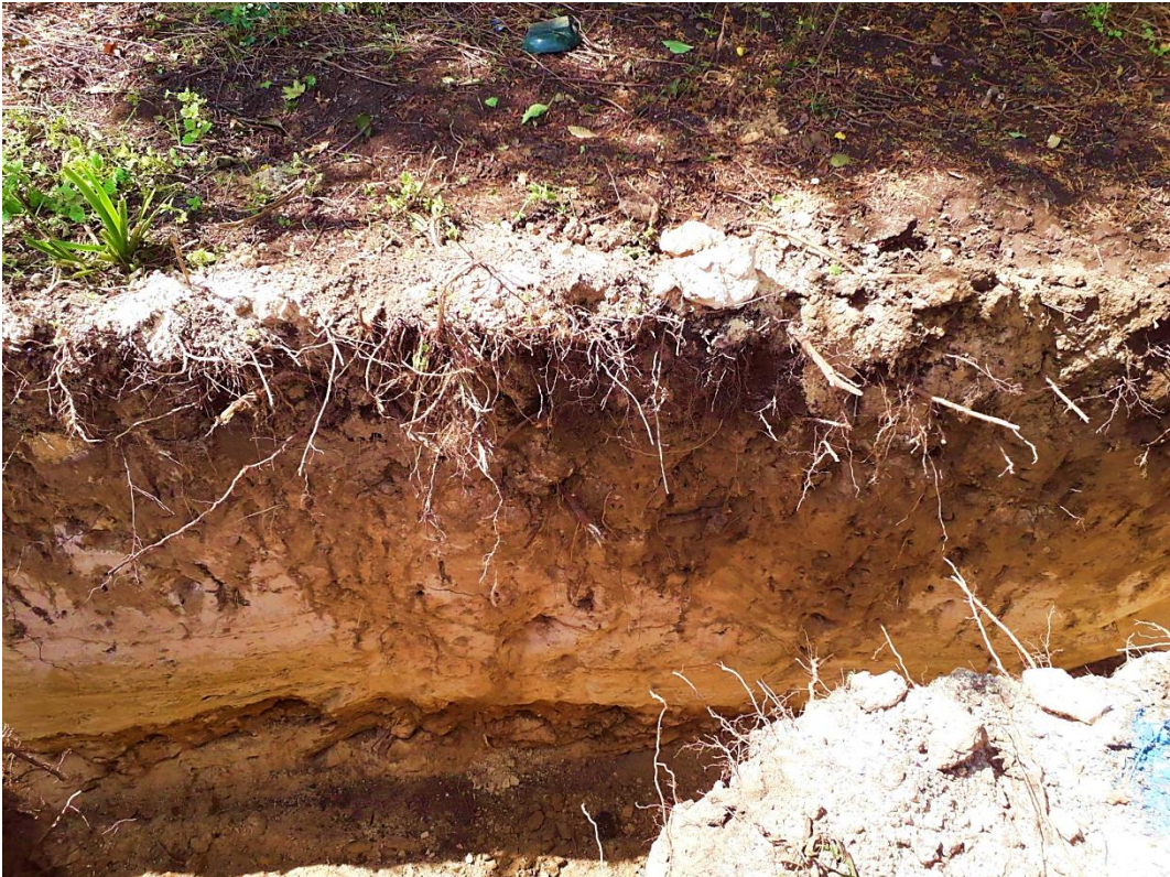
Foundation trench, plot 1, looking west Fig 6
