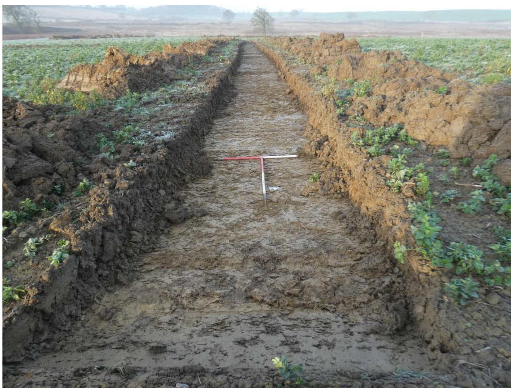
Fig 37: Trench 25, looking west
