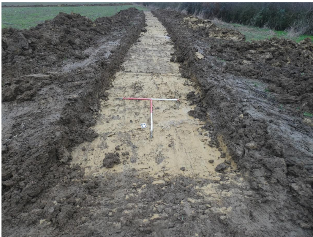
Fig 18: Trench 6, looking south-south-west
