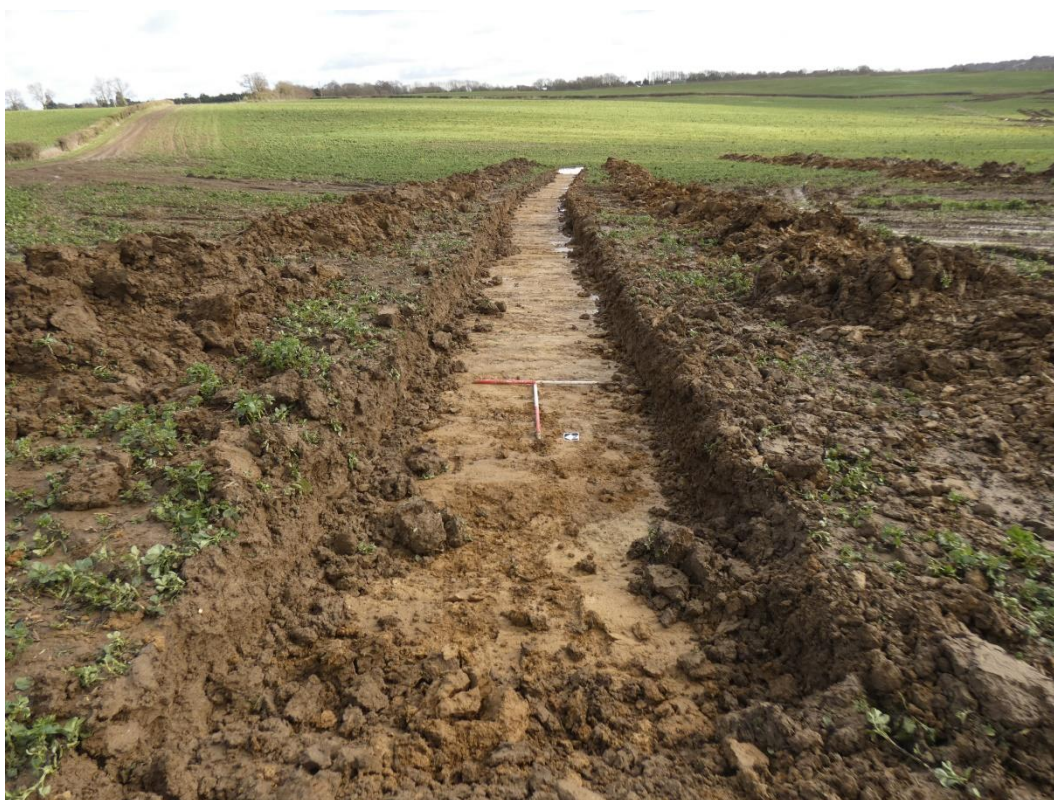
Fig 54: Trench 42, looking east
