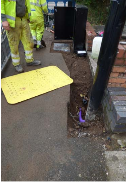
15 Service Trench looking east
