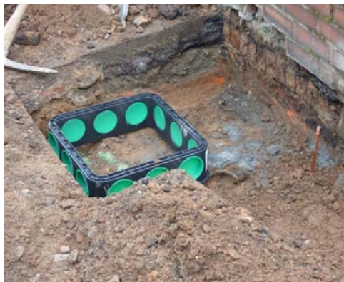
11 Service Trench looking south-east
