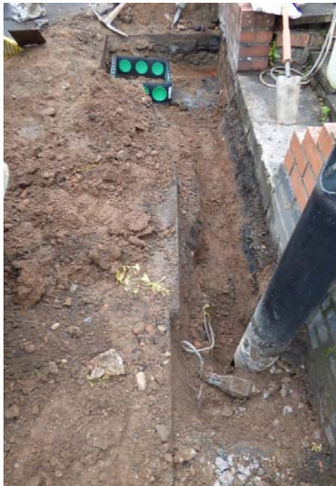
7 Service Trench looking east
