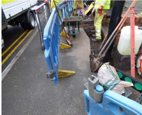
1 Service Trench looking east
