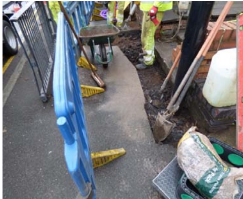
2 Service Trench looking east
