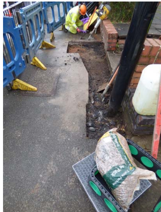
5 Service Trench looking east
