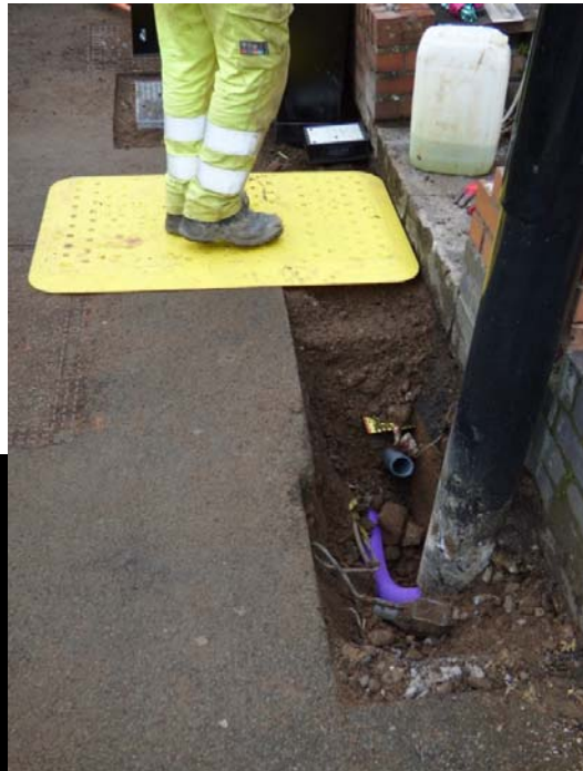
14 Service Trench looking east
