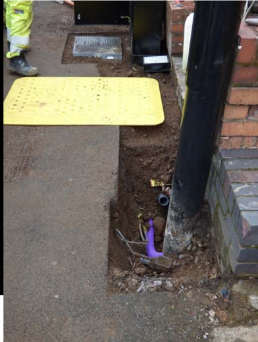
13 Service Trench looking east
