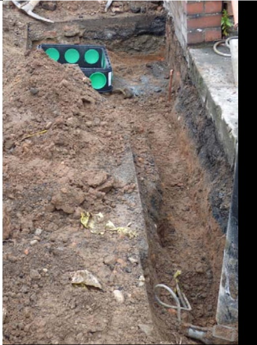
10 Service Trench looking east
