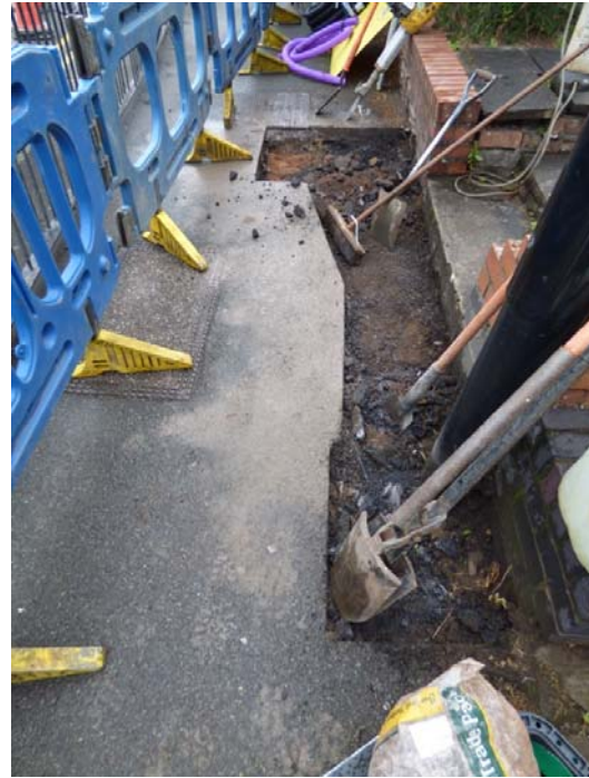
4 Service Trench looking east
