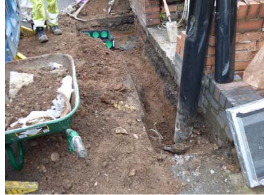
8 Service Trench looking east
