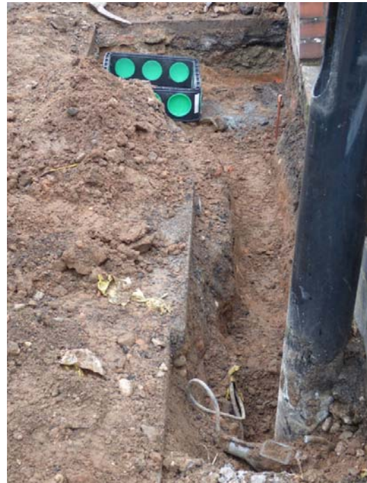
9 Service Trench looking east
