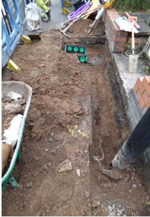
6 Service Trench looking east
