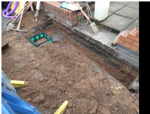
12 Service Trench looking east
