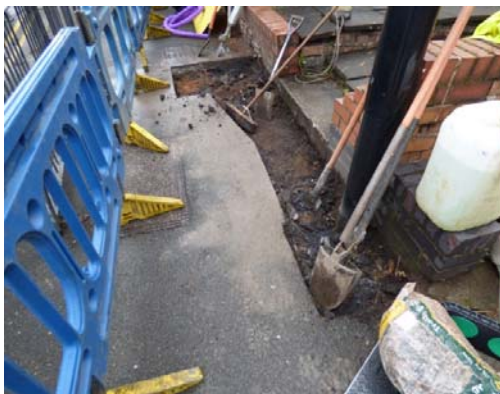
3 Service Trench looking south-east
