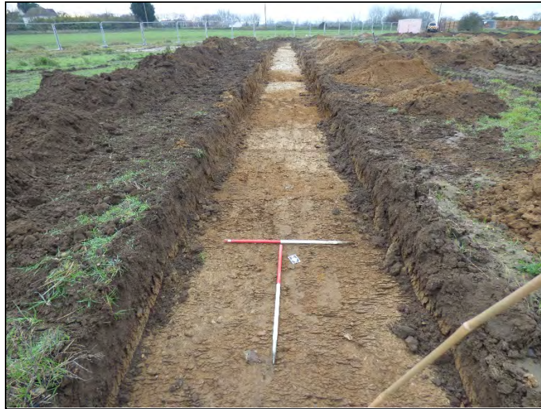
General view of Trench 4, viewed looking south-west
