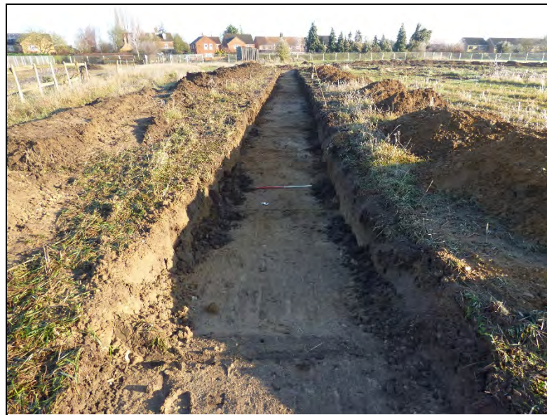
General view of Trench 13, viewed looking north-east
