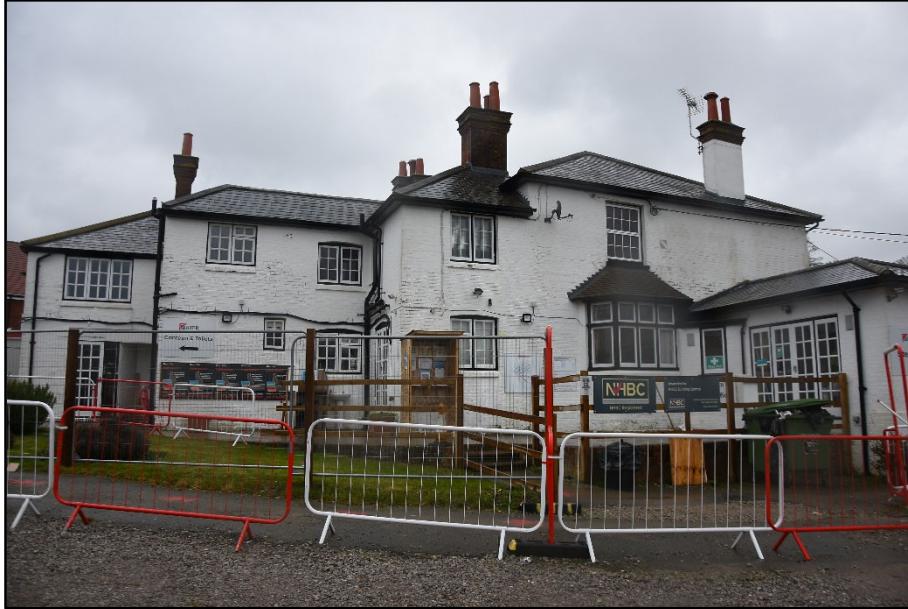
The south elevation, looking north-east Fig 13
