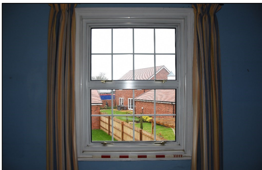
Window in FF06, looking north-east Fig 87
