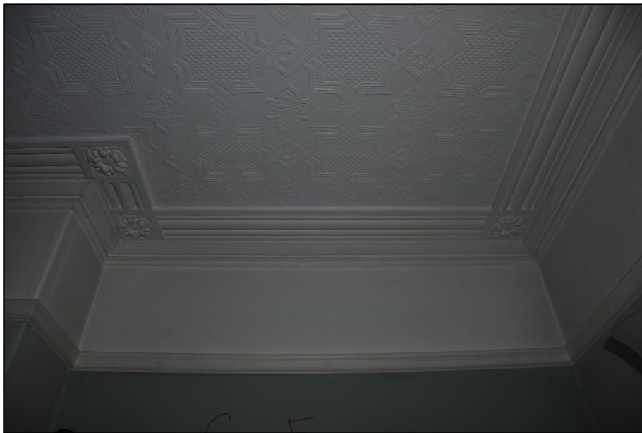
Detail of the cornice in GF02, looking north-east Fig 27
