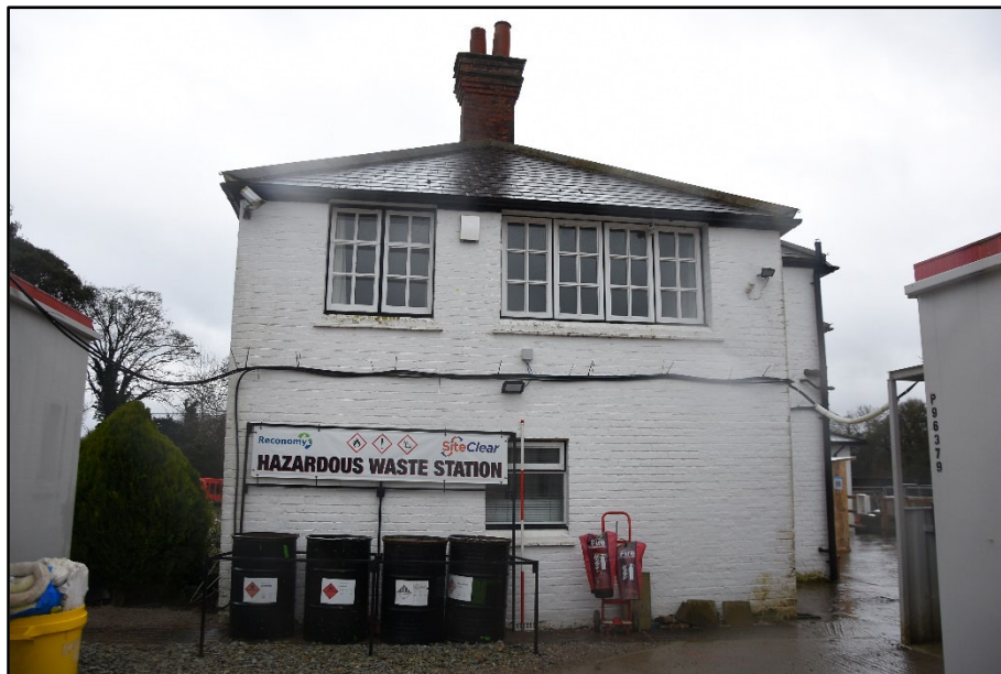
The west elevation, looking east Fig 11
