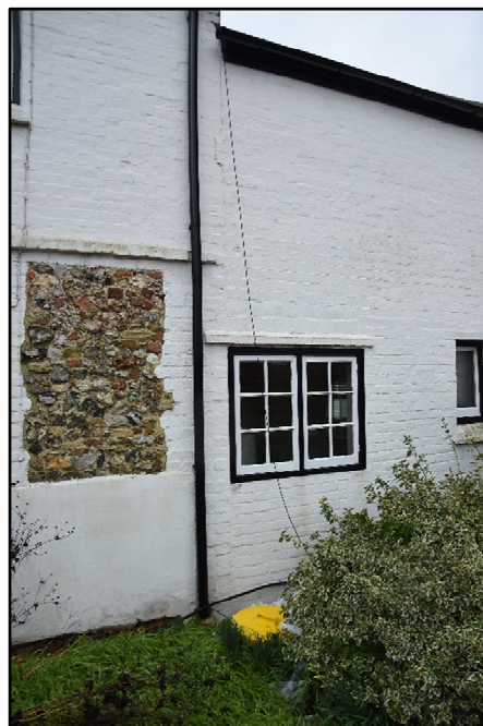
The join in the rear ranges between phases, looking south-west Fig 9
