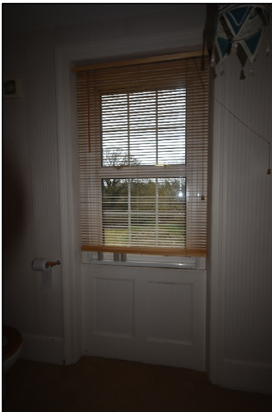
Window in FF03, looking south-east Fig 83
