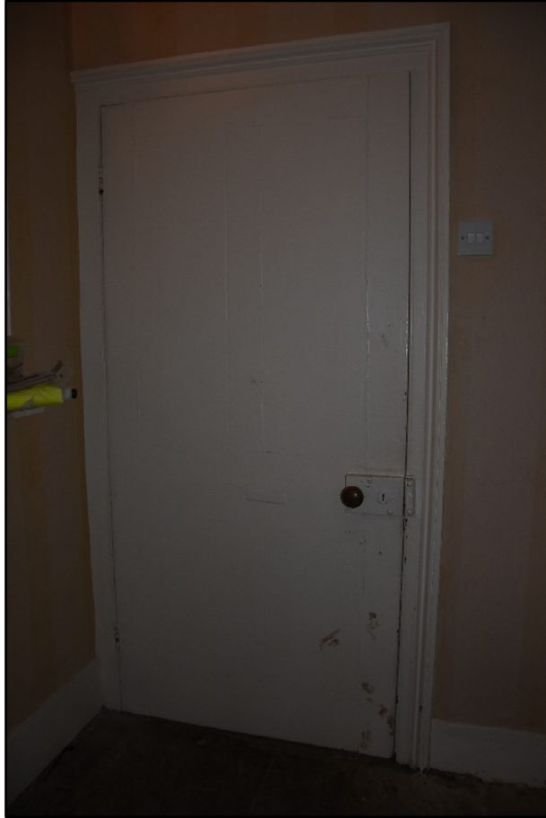
Door from GF01 in GF03, looking west Fig 35
