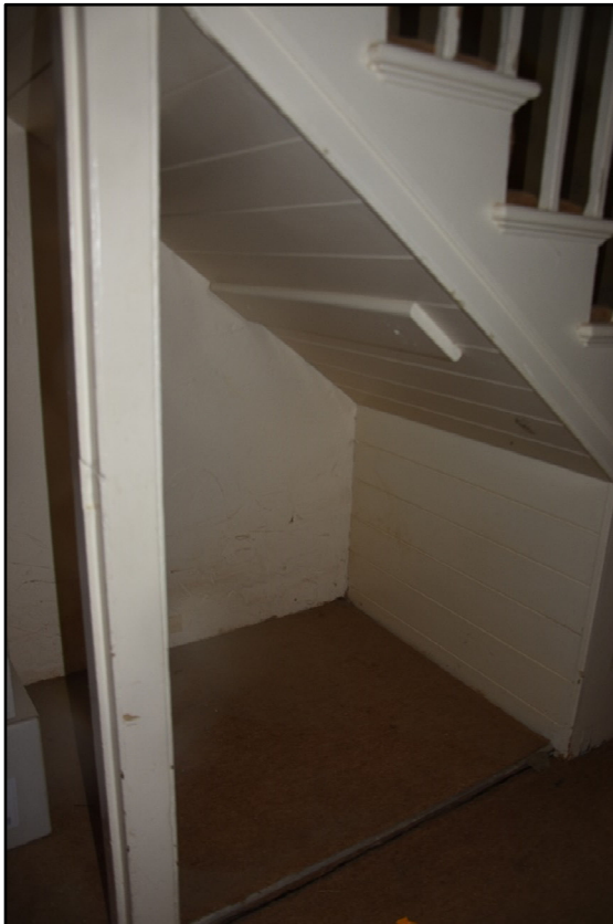
Area beneath the stairs in GF01, looking east Fig 24
