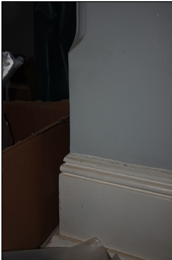
Chamfered and stopped corner to the bay window aperture, looking east Fig 31
