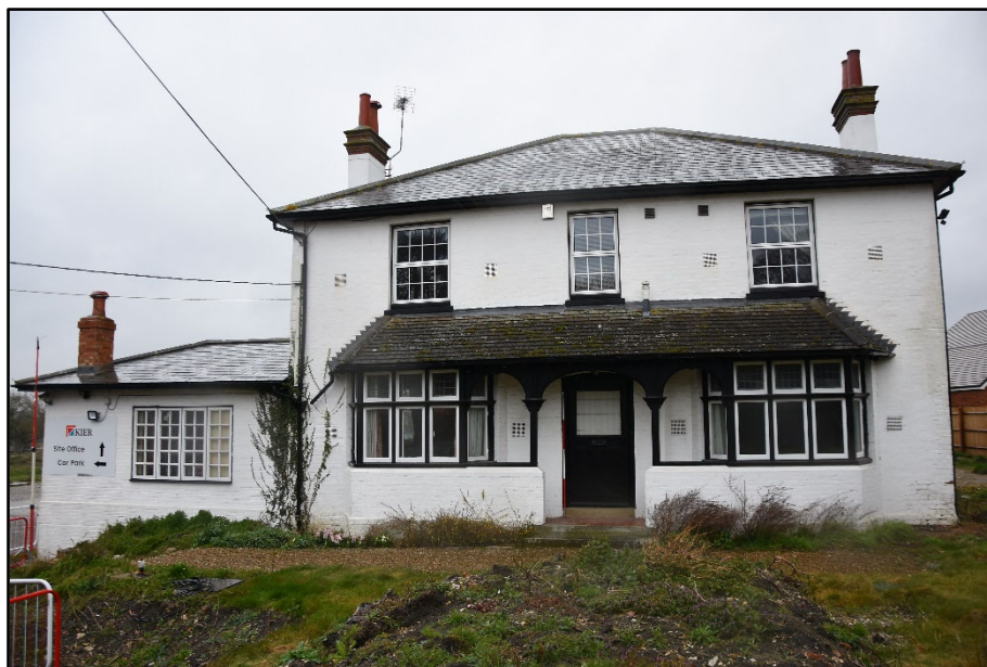
The east elevation comprising the main range, looking north-west Fig 5
