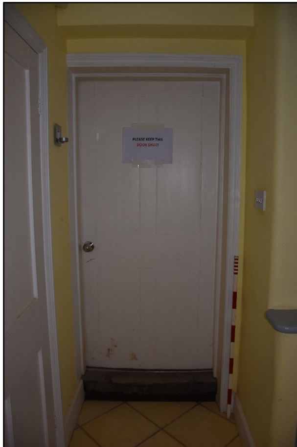
Door from GF01 into GF07, looking east Fig 47
