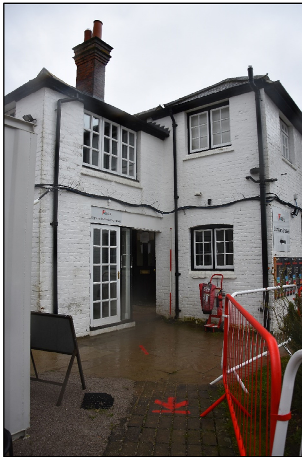
Junction of rear ranges along the south elevation, looking east Fig 15
