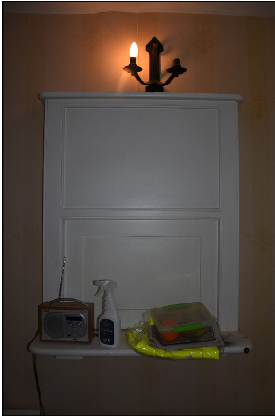
Service hatch through to GF02, looking south Fig 37
