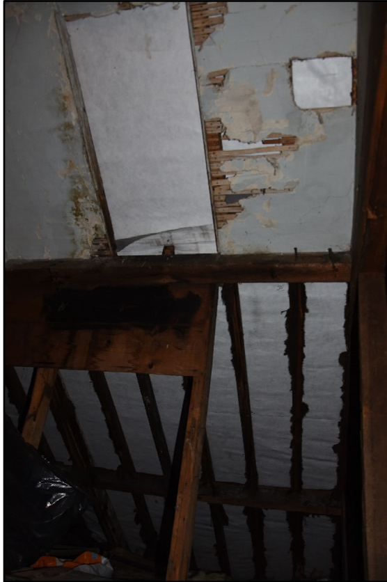
Lath and plaster around a former roof light, looking west Fig 112
