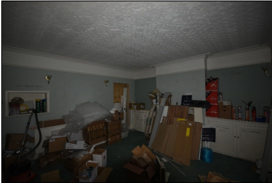
General view of GF02, looking north Fig 26
