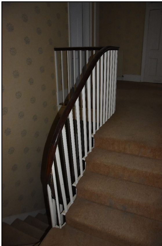
Section of balustrade in FF01, looking east Fig 70
