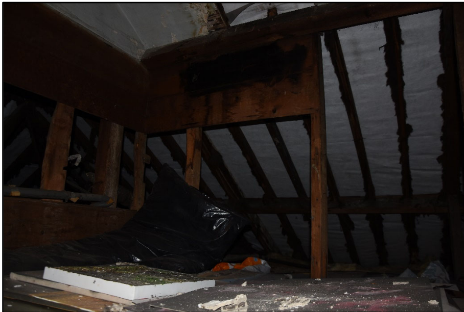
Formerly boarded attic space over the main range, looking west Fig 111
