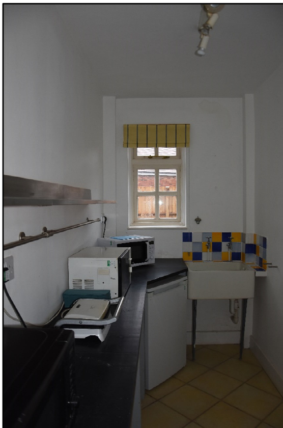
Interior of GF09, looking north Fig 56
