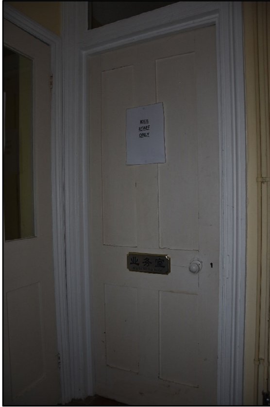
Door to GF10a, from GF10, looking north-east Fig 60
