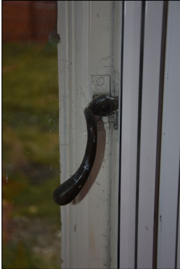
Window catch in GF02, looking south-east Fig 32
