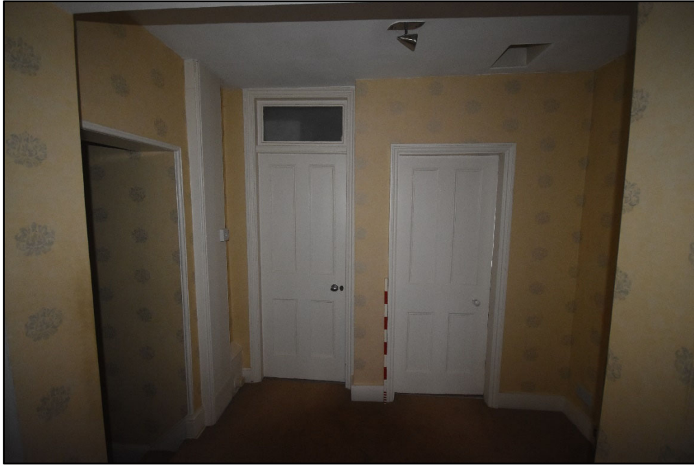
South wall of FF07, looking south-west Fig 89
