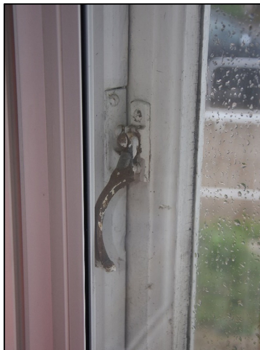
Window catches in GF04, looking south-east Fig 39
