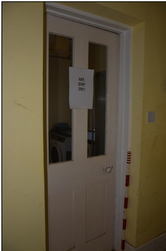
Door to GF10 from GF08, looking south-west Fig 57
