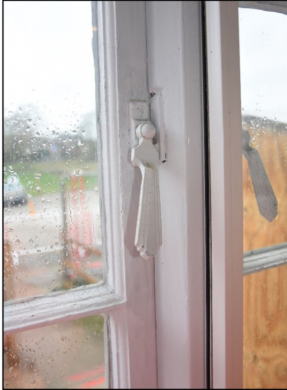
Decorative window catches in GF07, looking south-west Fig 50
