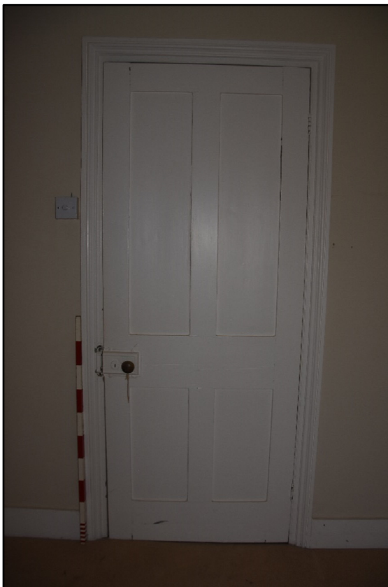
Door from FF07 into FF09, looking south-west Fig 96
