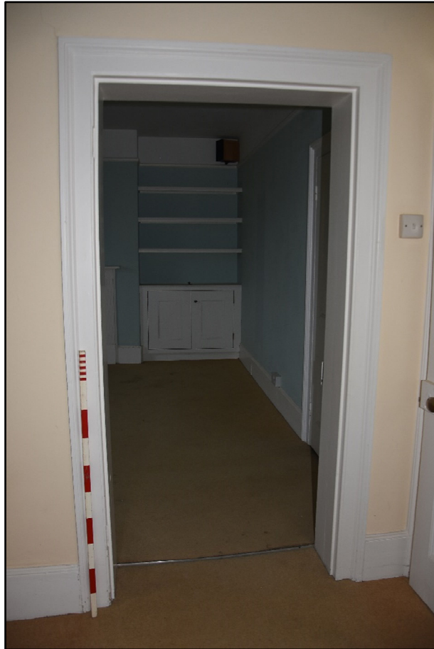
Doorway between FF03 and FF05, looking north-west Fig 81
