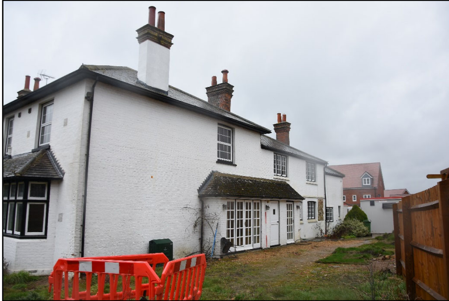
The long north elevation, looking west Fig 7
