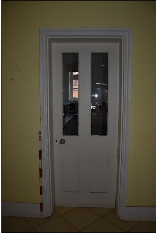
Door to GF09 from GF08, looking north Fig 55
