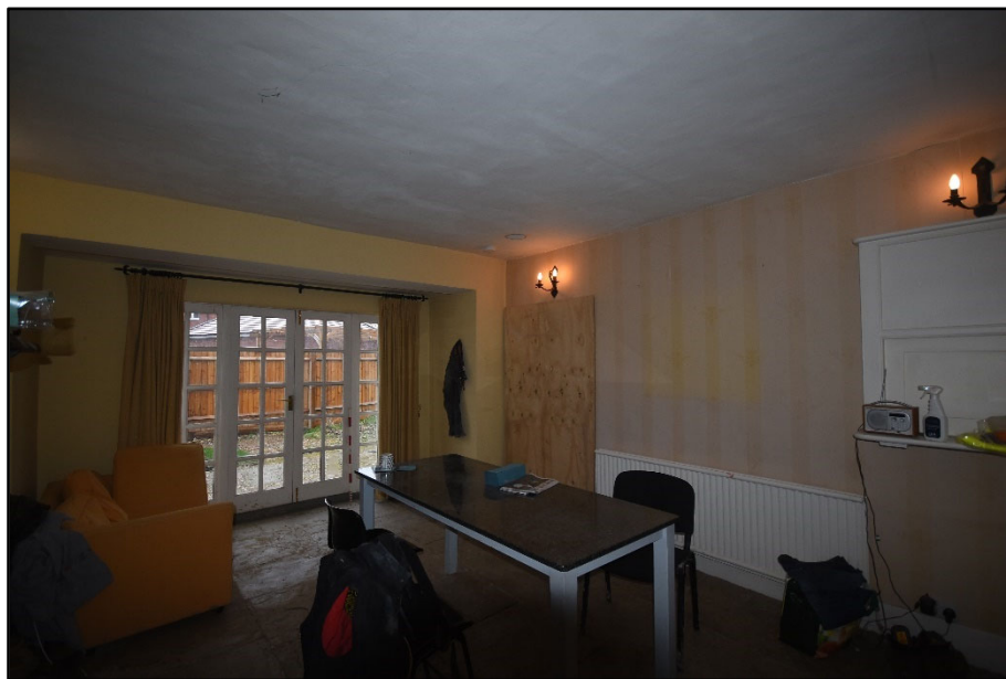
General view of GF03, looking north-east Fig 34
