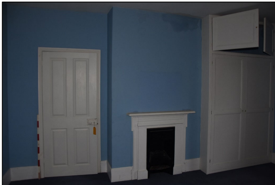
Interior of FF06, looking north-west Fig 86
