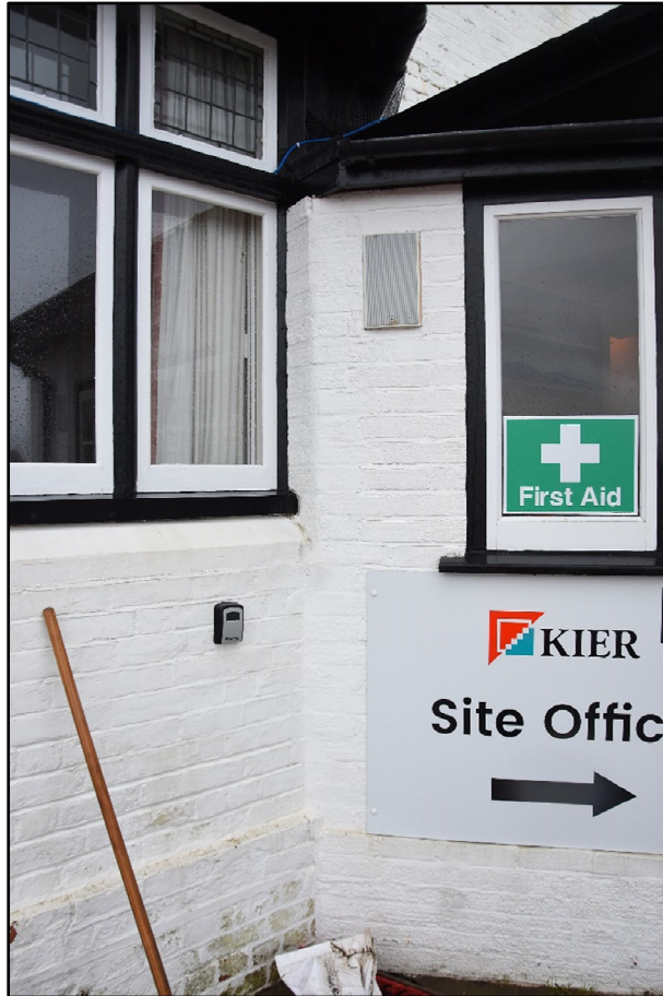
Canted section of wall between the bay window and southern extensions, looking north Fig 14
