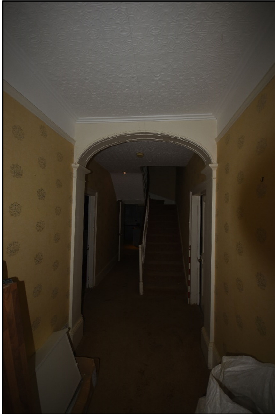
General view of GF01, looking north-west Fig 19
