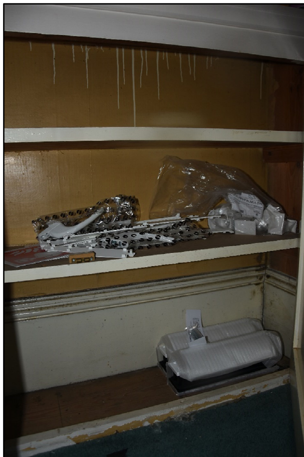
Interior of the cupboards in GF02, looking north-east Fig 29
