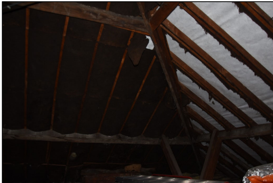
Roof structure over the main range, looking north-east Fig 113
