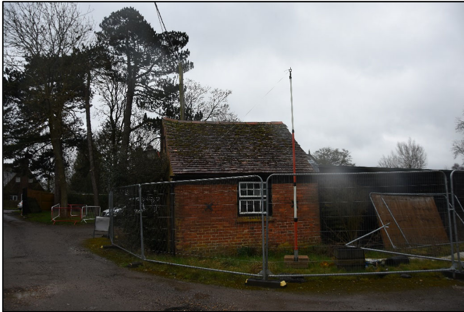
Outbuildings to the south-east of the house, looking south-east Fig 17
