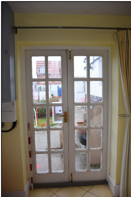
Double doors in GF07, looking west Fig 51
