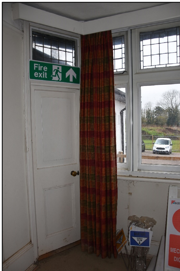
Door to GF06 from GF05, looking south-east Fig 43
