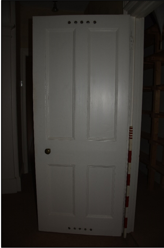
Rear of the door to FF01a, looking north Fig 73
