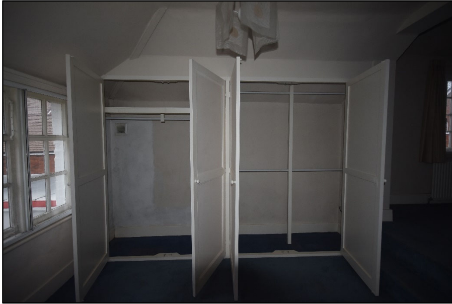
Interior of the cupboards in FF13, looking north-east Fig 109
