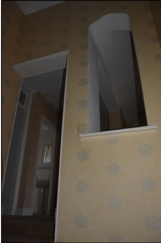
Area above the stairs looking west towards FF07 Fig 69
