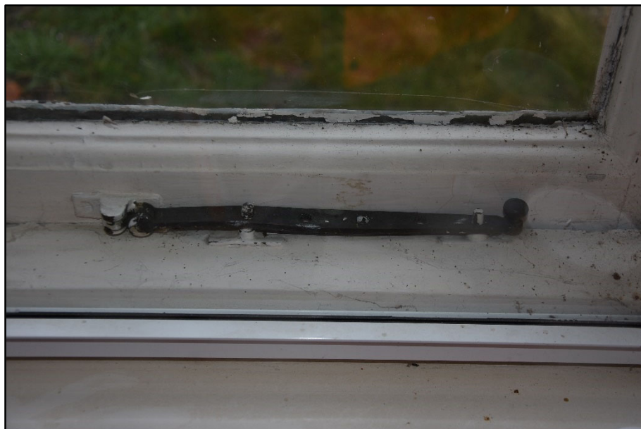
Window stay bar in GF02, looking south-east Fig 33
