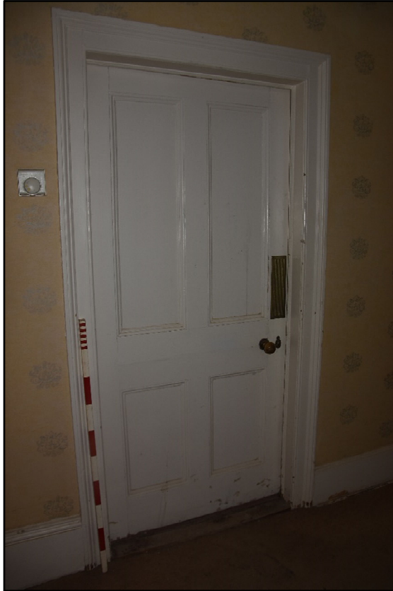
Typical door type seen in the main range, looking south-east Fig 21
