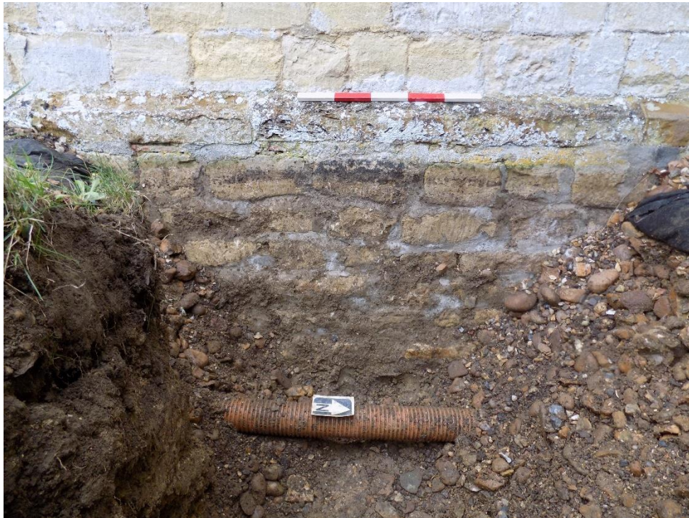
The southern church wall [1005/1025] with plastic pipe, looking west Fig 5
