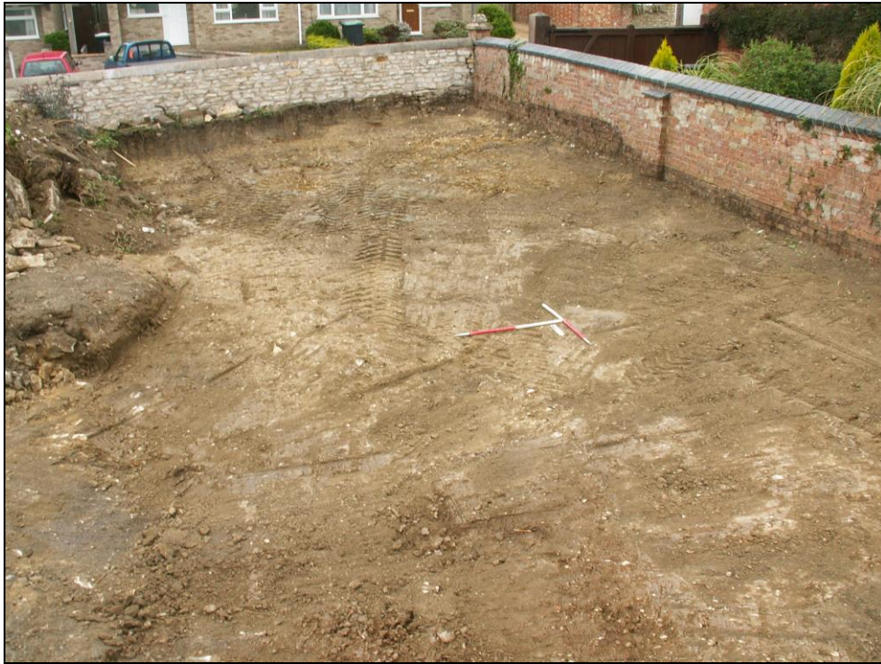
Figure 3. Overview of site after stripping of topsoil (101). Southwest facing photo.
