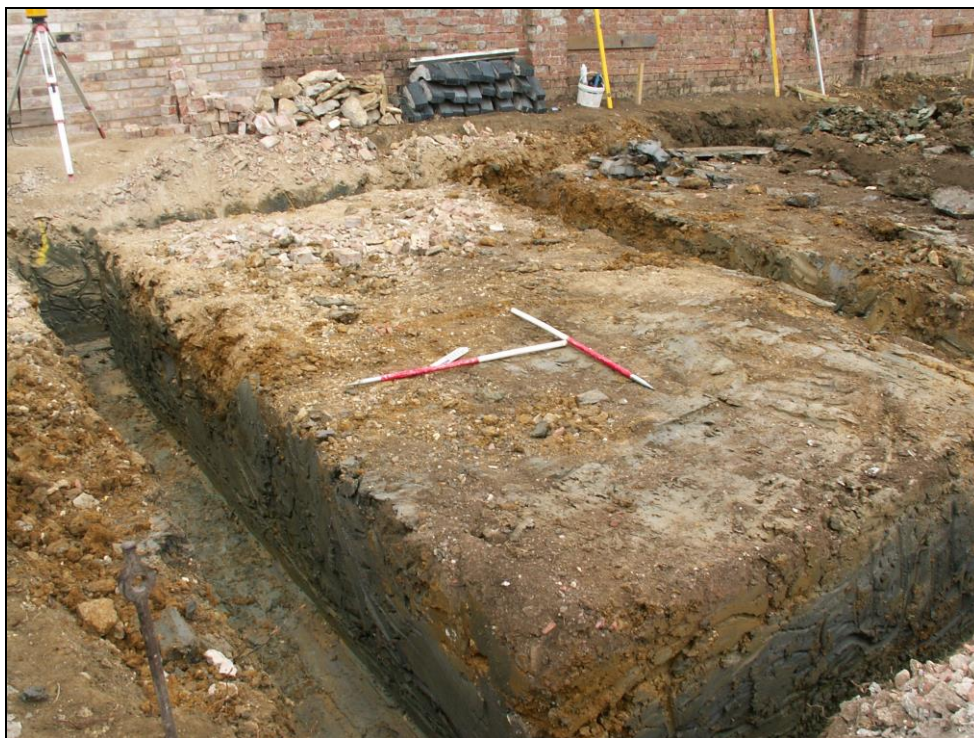
Figure 5. Foundation trenches in the southern part of site. Northwest facing photo.
