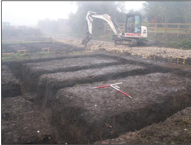
Figure 3. Overview of site from Plot 1. North east facing photo.
