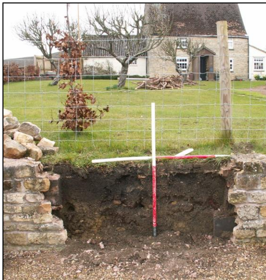
Figure 3. The deposits behind the modern retaining wall were about 0.60m thick, and were made up of modern garden soil.
