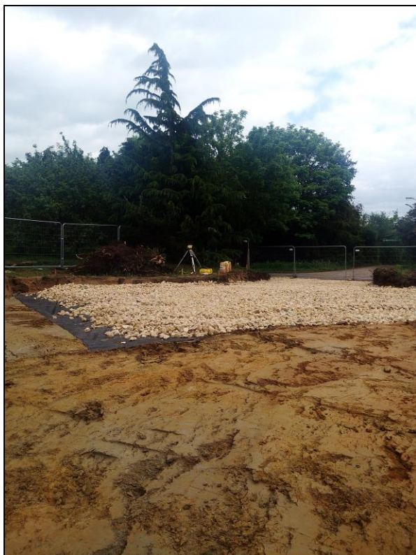
Figure 3. A large area in the southeast corner of the development site was initially stripped down to natural deposits in order to allow a geotextile cloth and hardcore to be put in. This was necessary to allow access for heavy transports. The entrance area from northwest.
