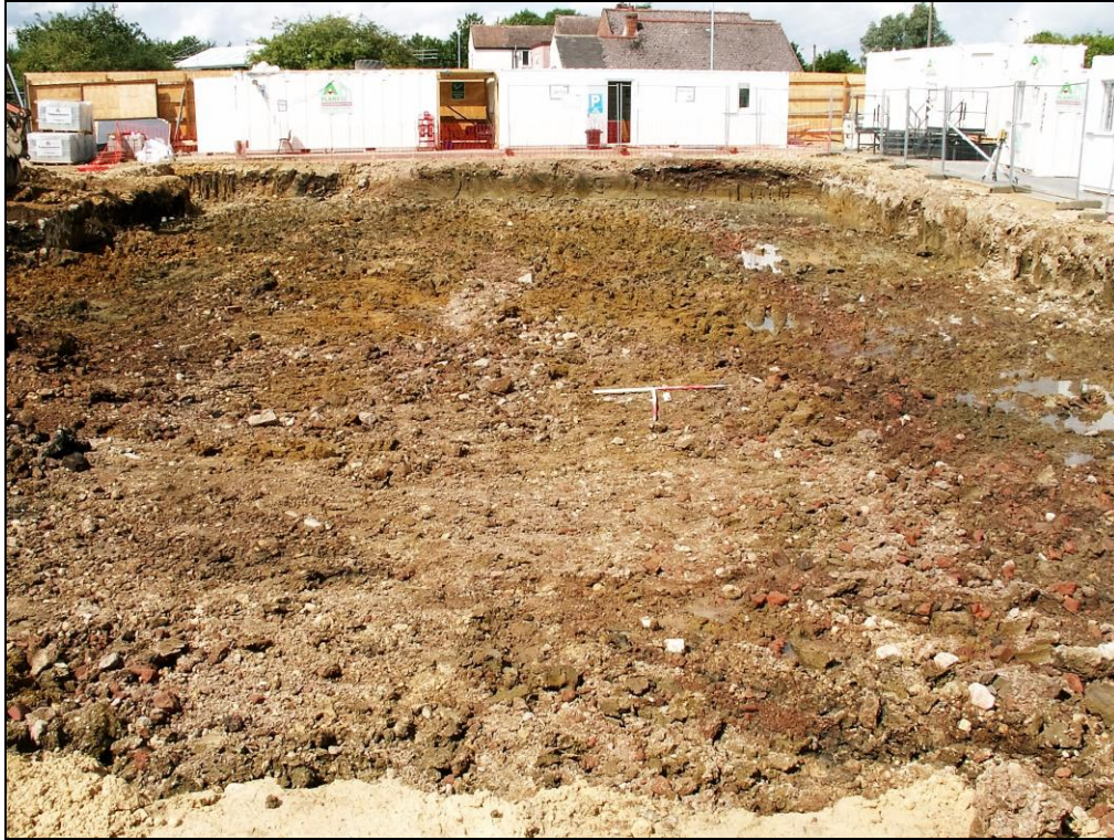
Figure 4. Overview of the area facing north. The ground was showing clear signs of having been previously disturbed down to a depth of about 0.7m below the present ground level.
