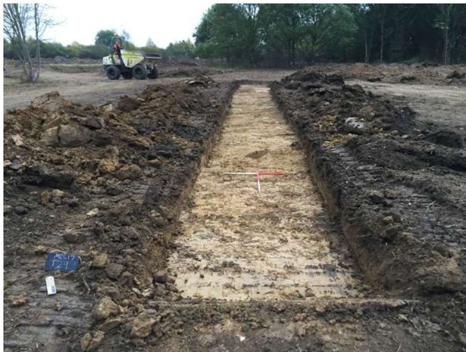
Photo 6: Trench 29 Looking north east
