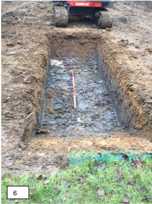
Figure 6: Trench 3 facing north showing concrete casing north-west corner of trench
