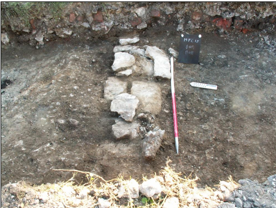
Figure 5. Stone wall foundation [102] in the southern part of Trench 1 was possibly from a former Post Medieval farm building within the area.
