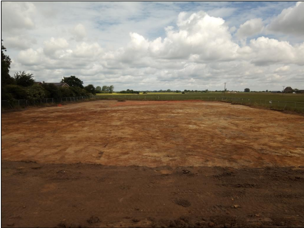
Figure 10. Overview photo of the northern half of the investigation area after stripping.
