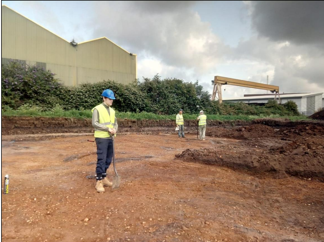
Figure 4. Working photo from the stripping of the site.
