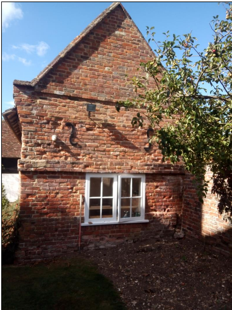
Figure 20. The north east wall of the coach house.
