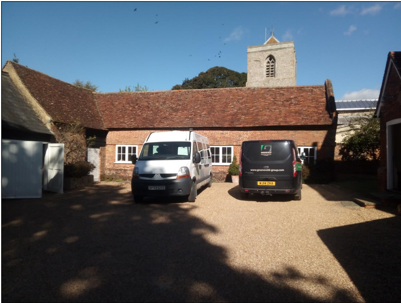
Figure 19. The 17 th century coach house from south east.
