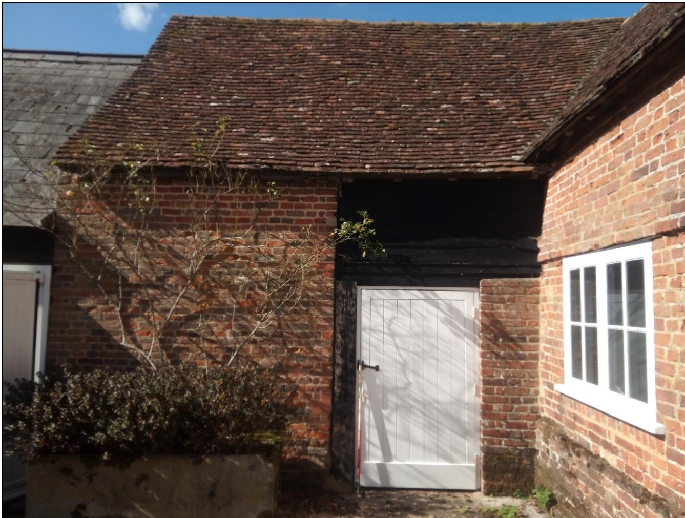
Figure 26. The section where the wooden outbuildings met the brick-built part of the coach house. South west facing photo.
