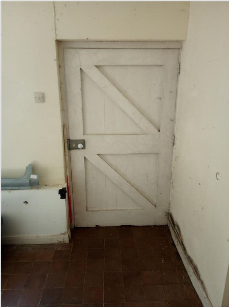
Figure 33. A door in the 17 th century coach house. South east facing photo.
