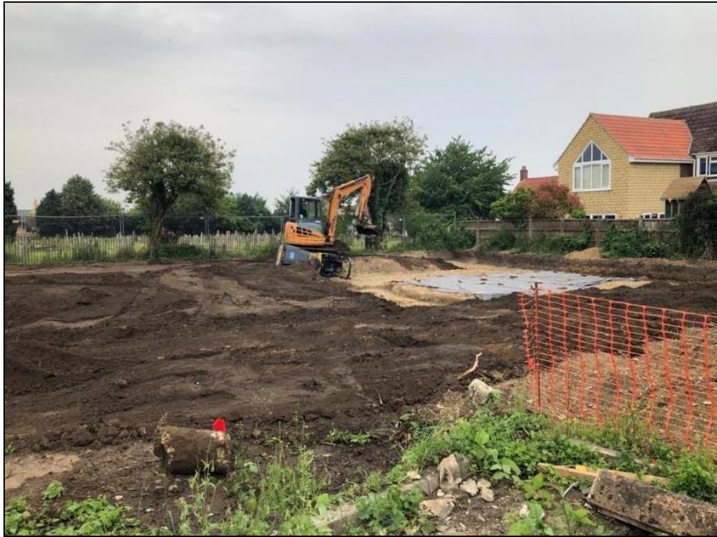
Figure 5. The laying out of the geotextile over the Roman house. Photo from southwest.
