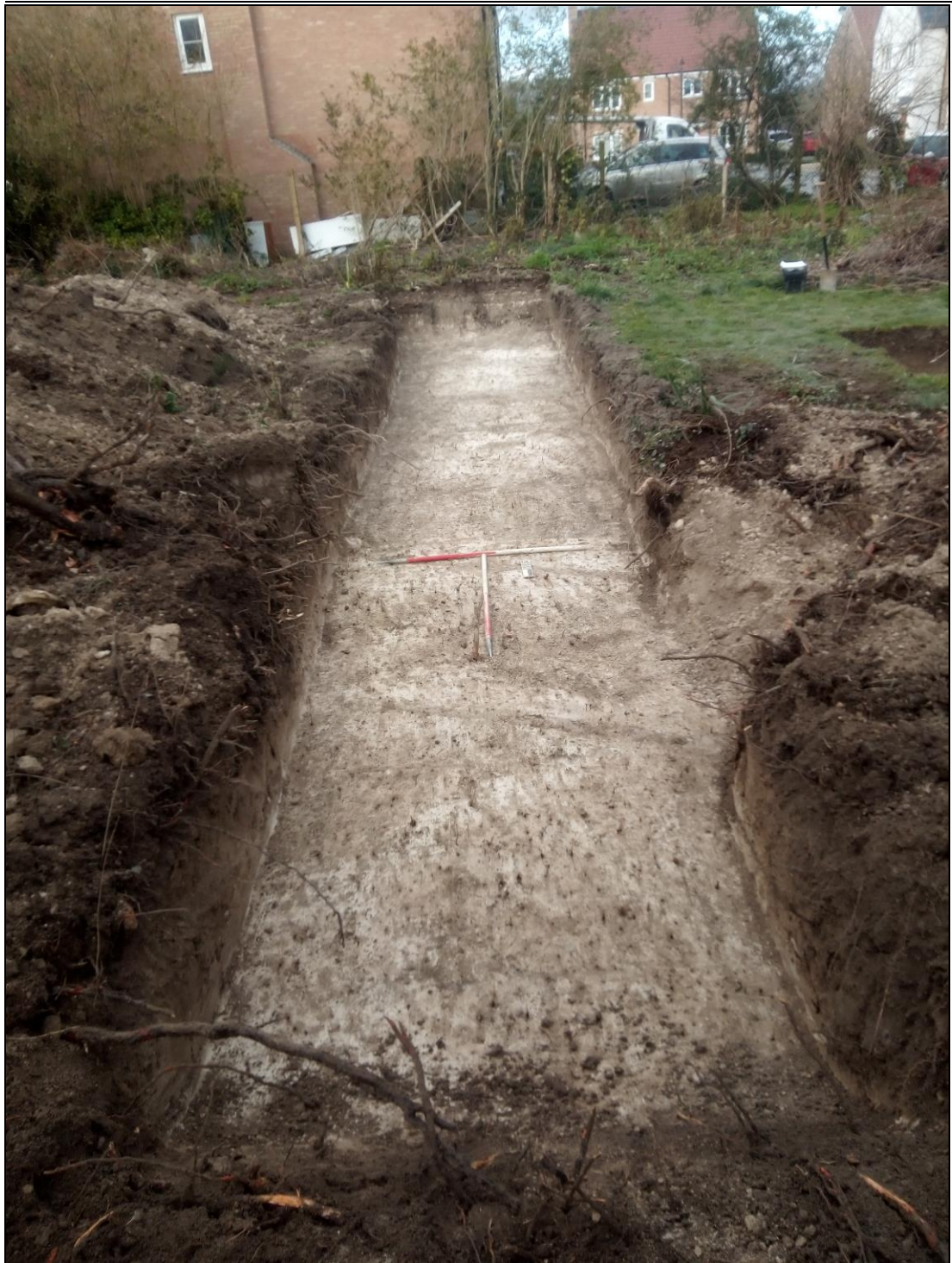
Figure 6. Trench 2 from south.
