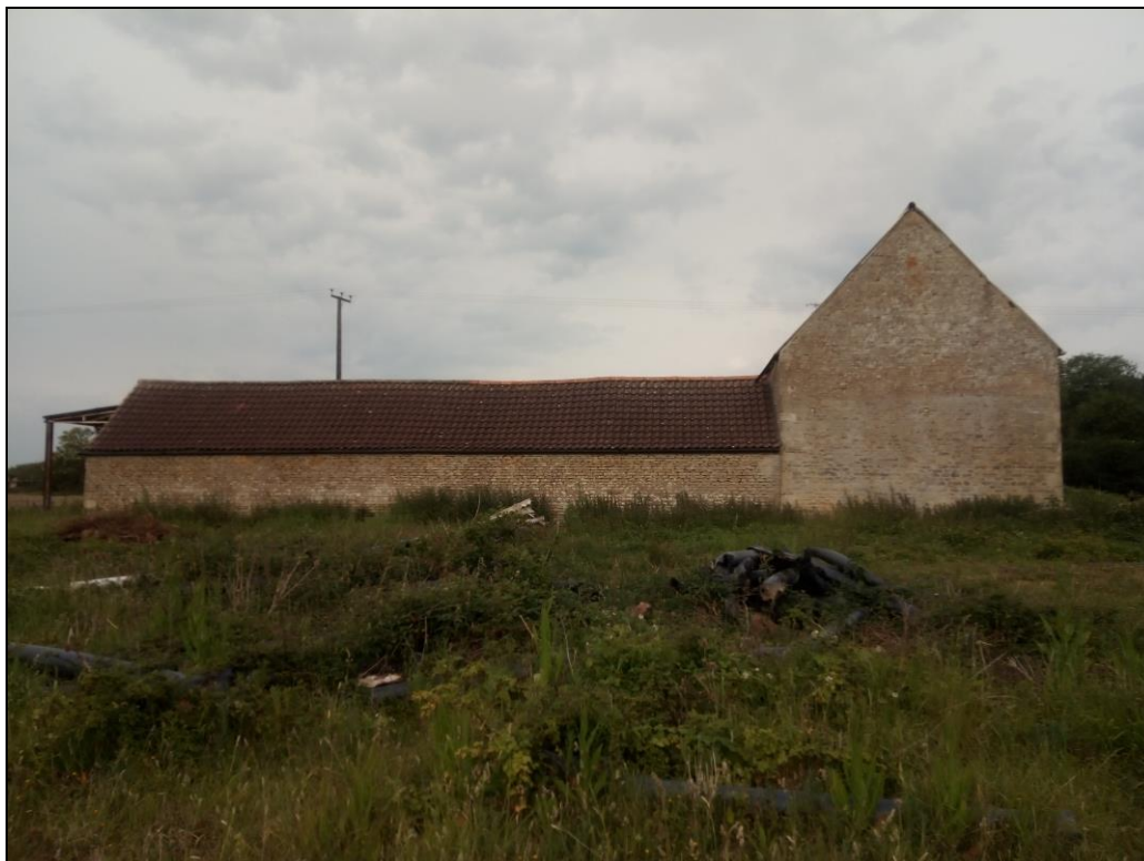
Figure 11. The barn complex from east.
