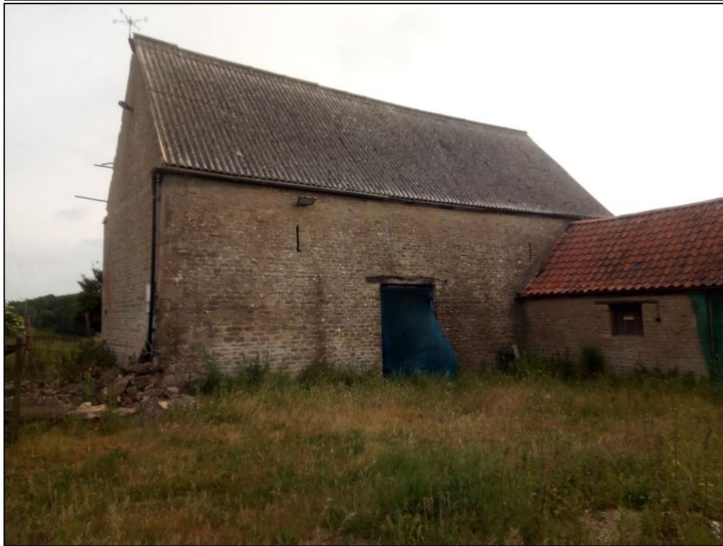
Figure 14. The original barn and the later stone extension from southwest.
