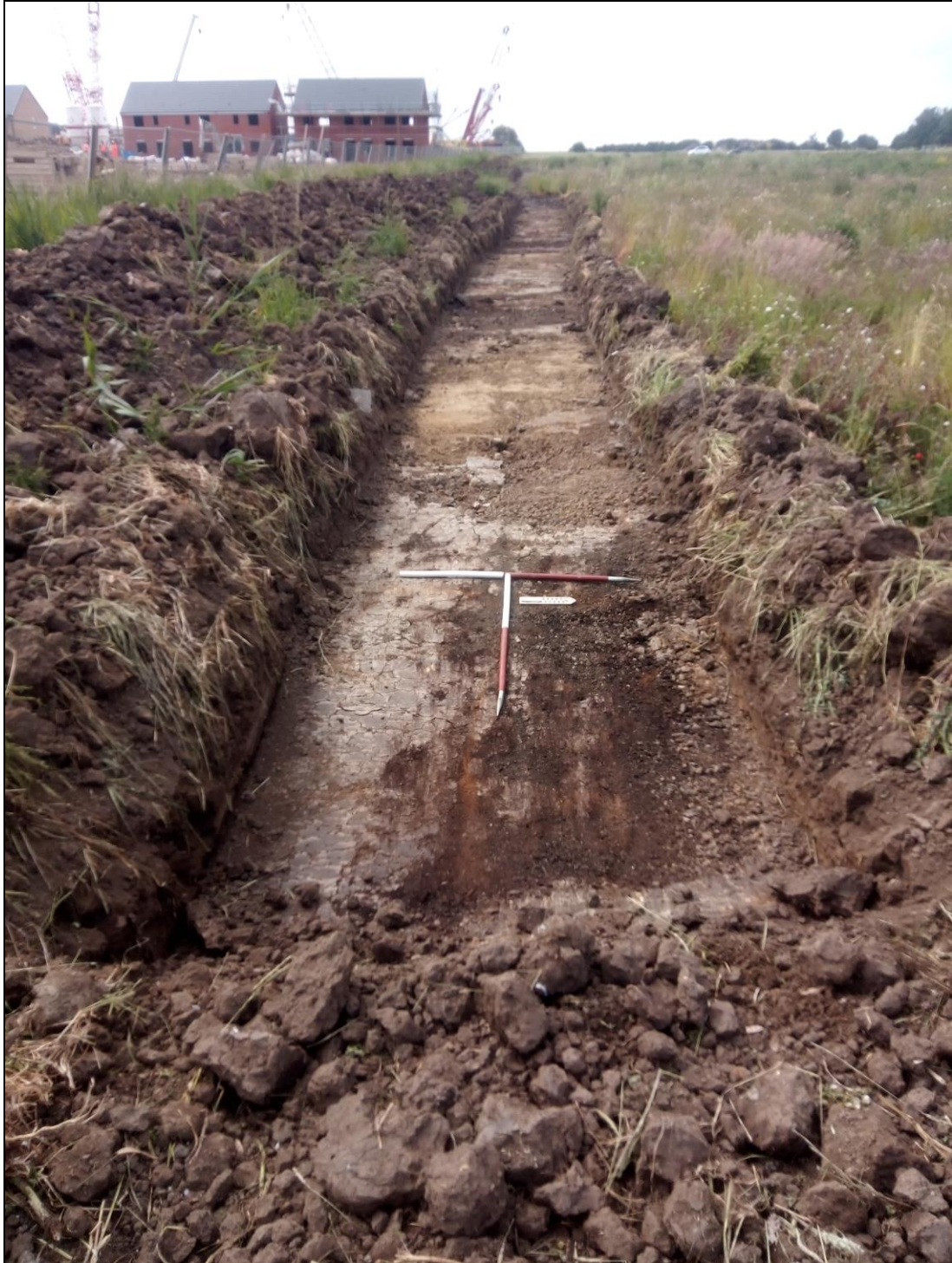
Photo 8: Overview of Trench 7 from east.
