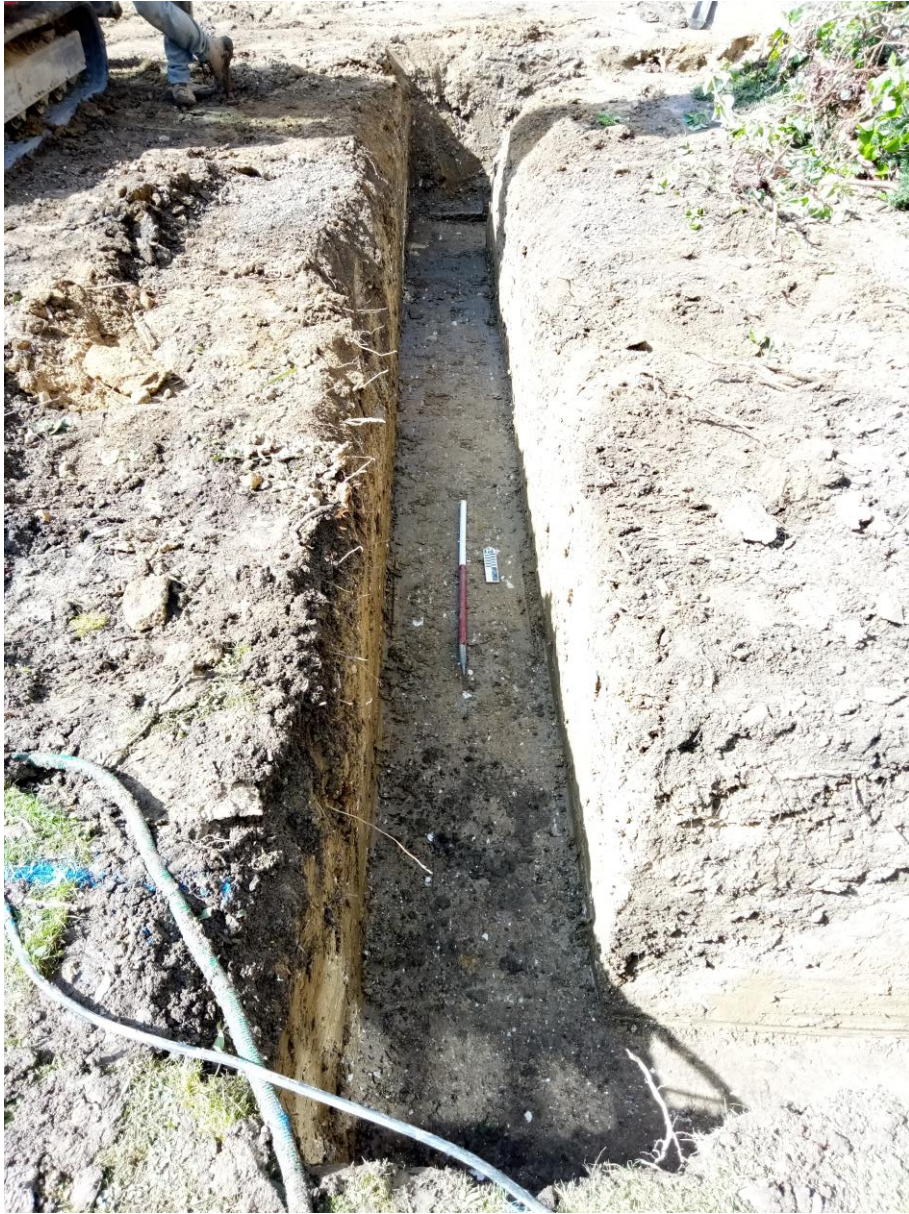
Figure 5. North facing photo of the new footings in west.
