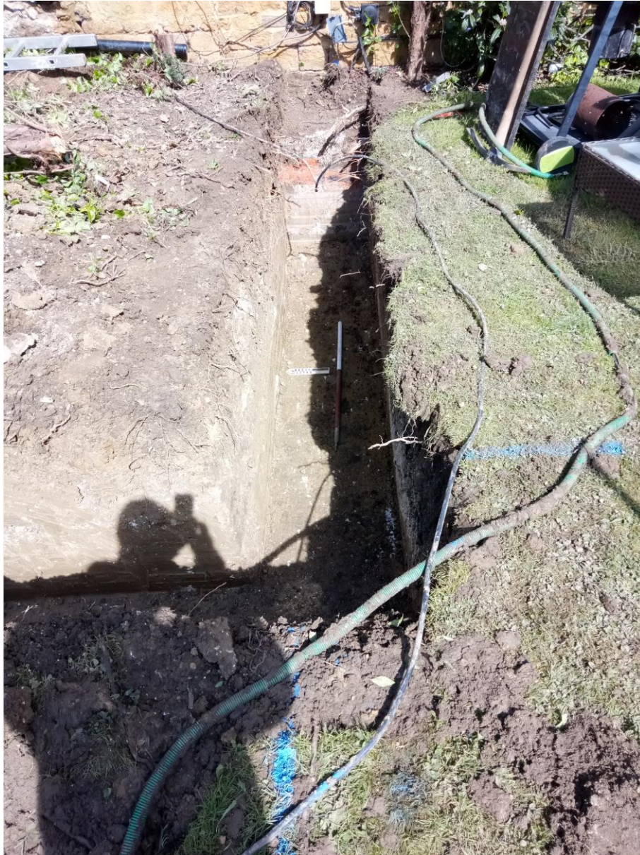
Figure 6. East facing photo of the new footings in south.
