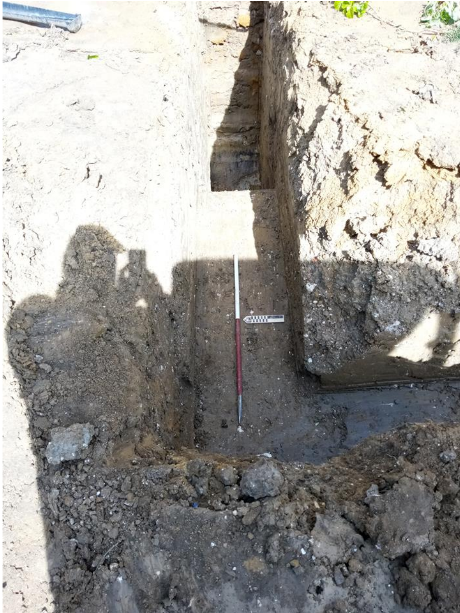
Figure 4. East facing photo of the new footings in north.
