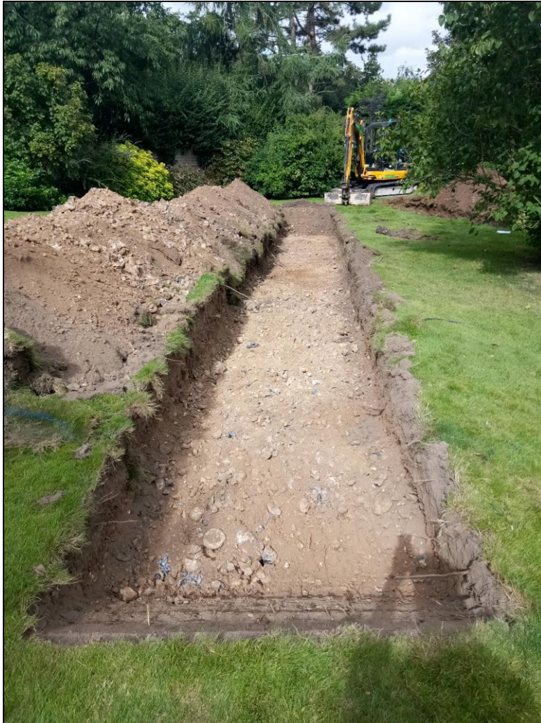
Photo 1: Overview of Trench 1 from north west.
