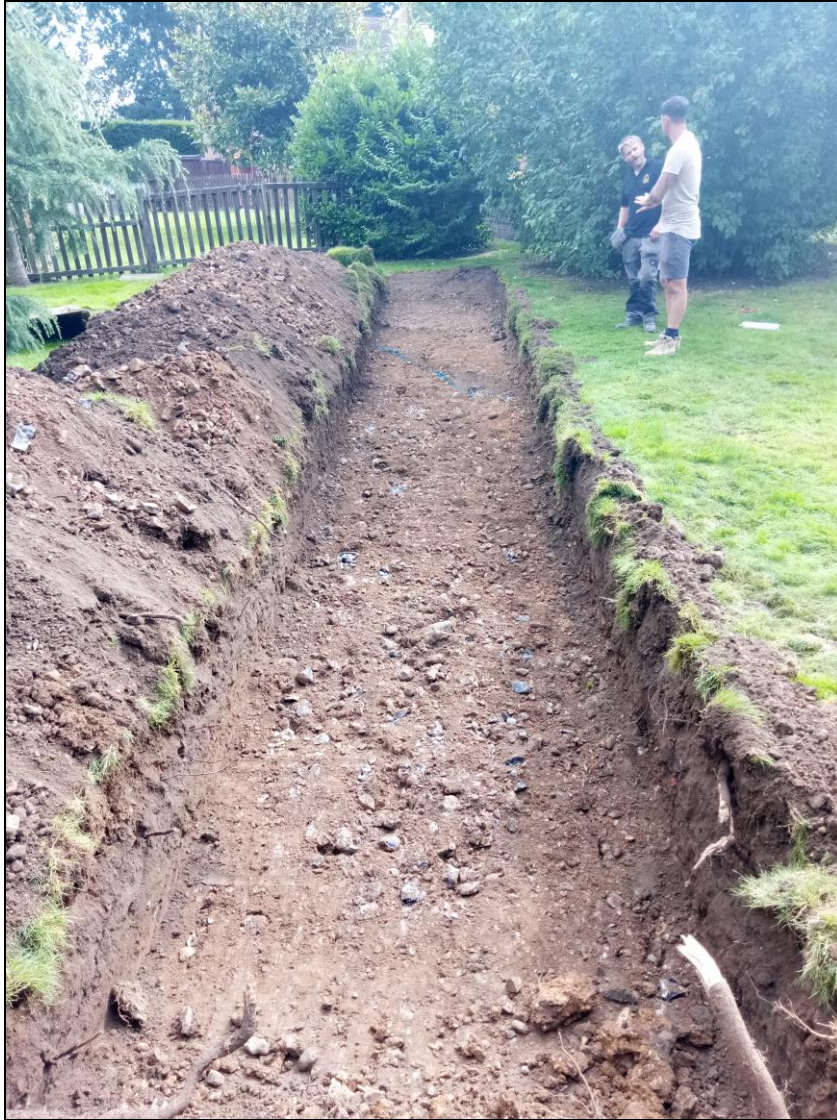
Photo 2: Overview of Trench 2 from west.
