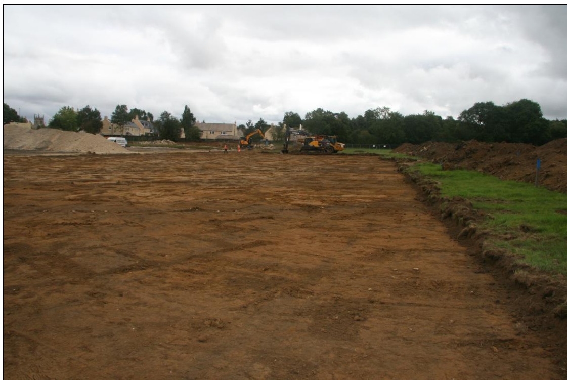
Photo 2: Overview of site from west.
