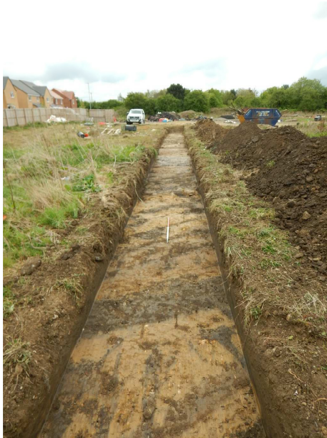
Plate 1: Trench 1 looking south (ENE-WSW service in foreground)
