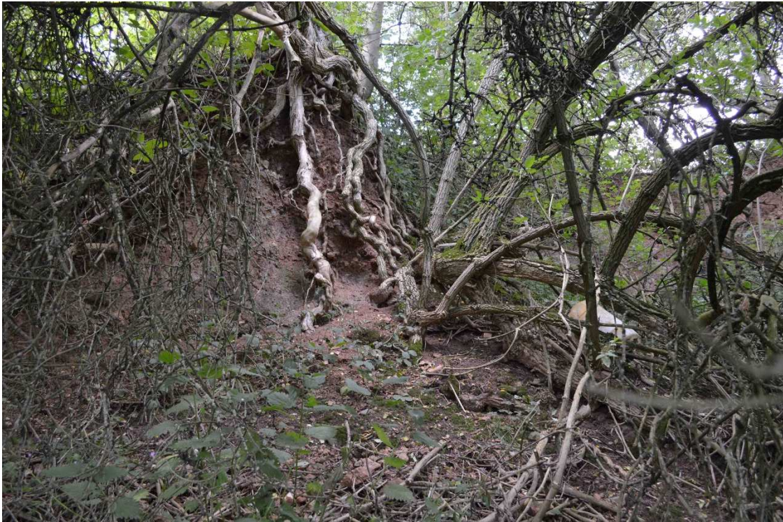
Plate 23: View of the north face of quarry cutting (area B), facing north The diverted stream lies within a dyke immediately beyond the trees on the edge of Field 3
