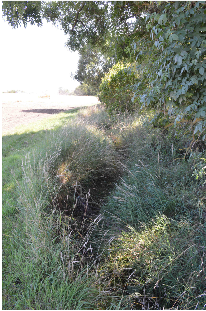
Plate 37: View of the dyke for diverted stream alongside area B, facing east
