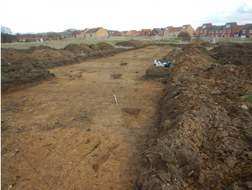
Plate 2: Gully 103 looking east
