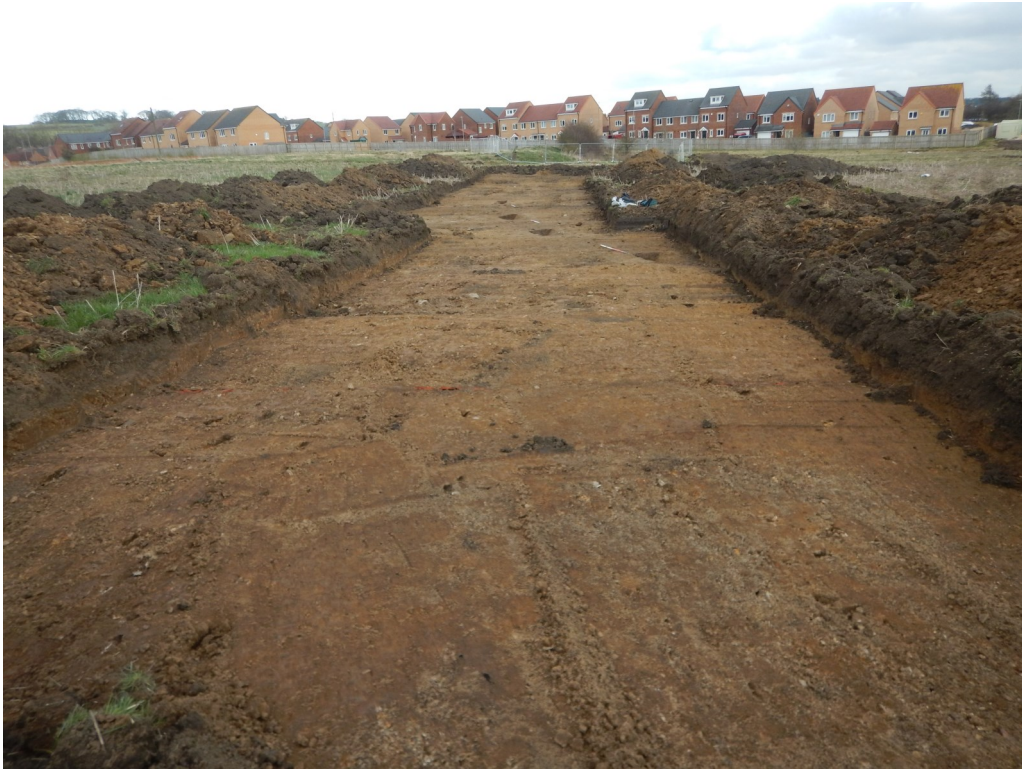
Plate 1: Excavation area looking east-south-east
