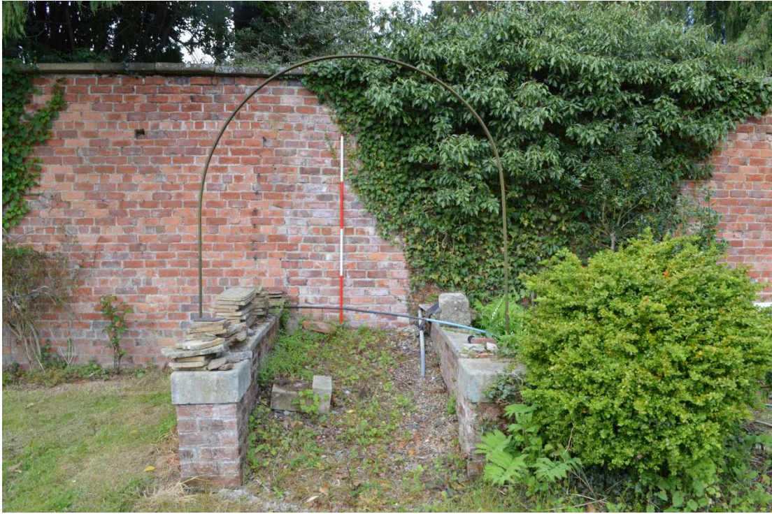
Plate 8: Blocked doorway in southwest garden wall , facing southwest
