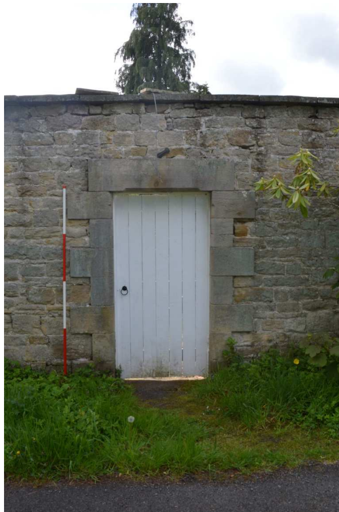
Plate 3: Doorway in the exterior of the northwest wall, facing southeast
