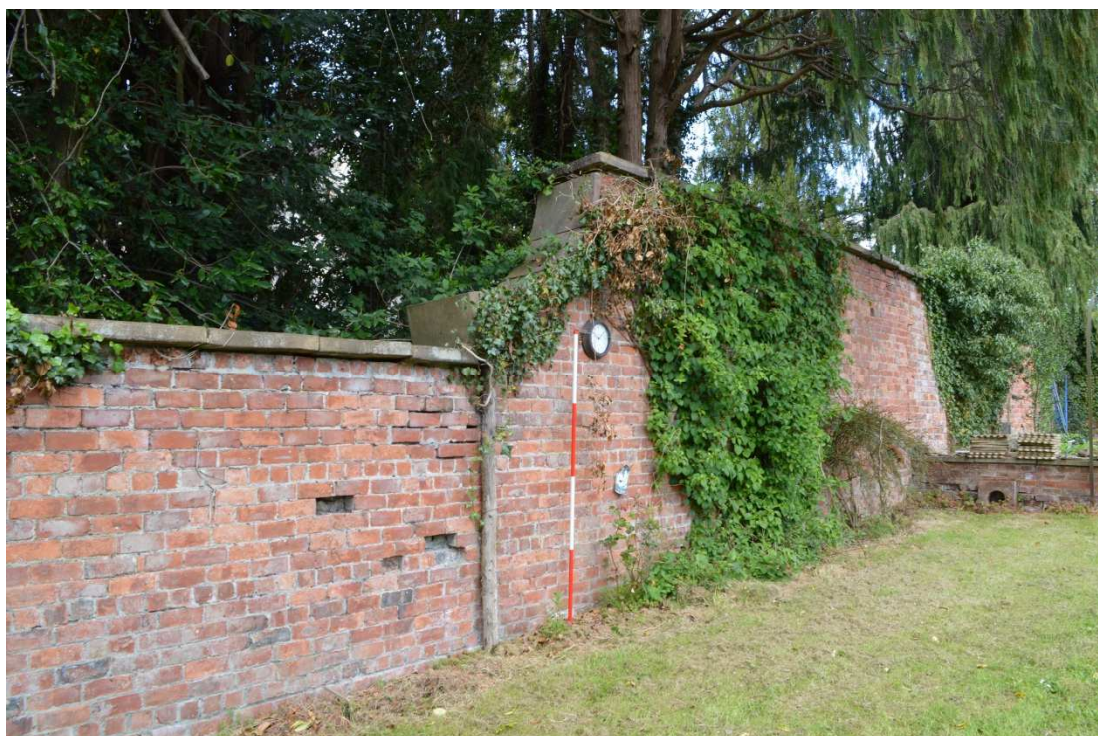
Plate 6: View of northeast garden wall interior, facing north (Note the coping stones missing from the southern length of the wall)
