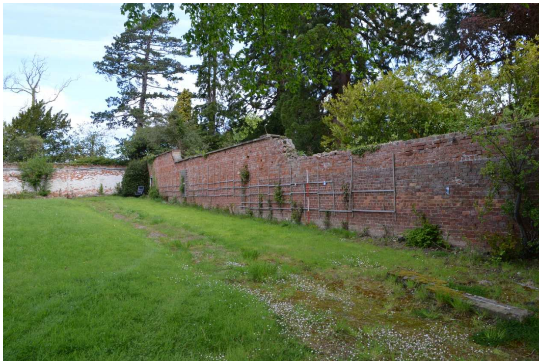
Plate 6: View of northeast garden wall interior, facing north (Note the coping stones missing from the southern length of the wall)
