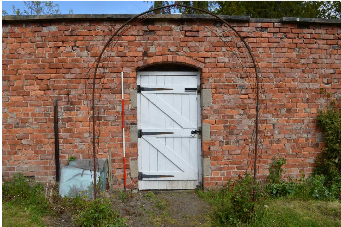
Plate 4: Doorway in the interior of the northwest wall, facing northwest
