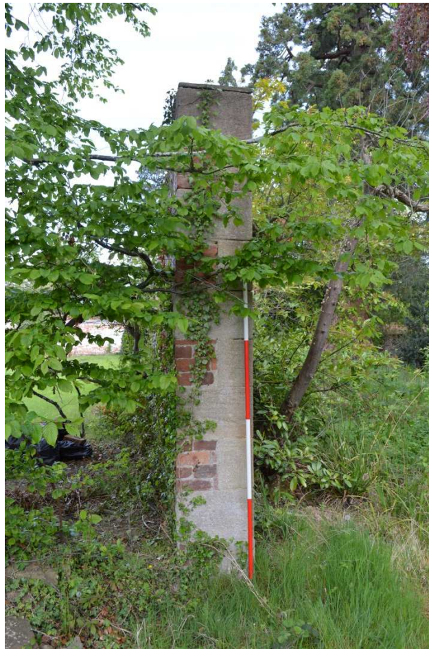
Plate 11: South end of the northeast wall, facing northwest
