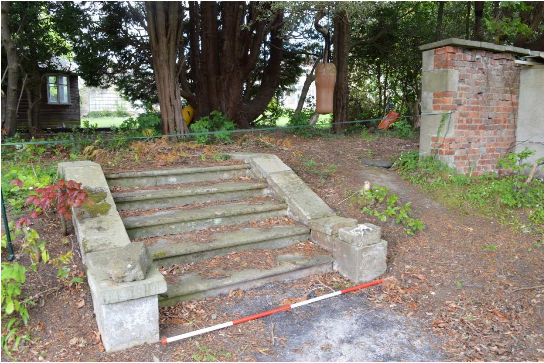
Plate 10: Steps leading from garden with the south end of the southwest wall in the background, facing west
