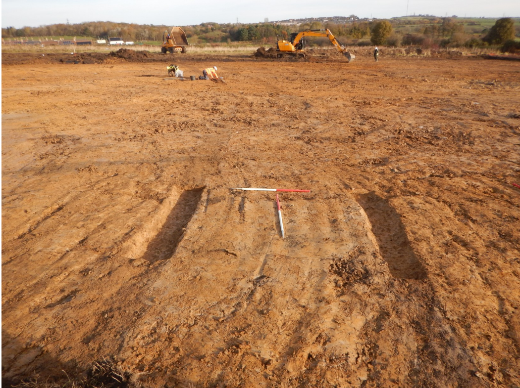
Plate 13 Gullies 1008 & 1010 looking north
