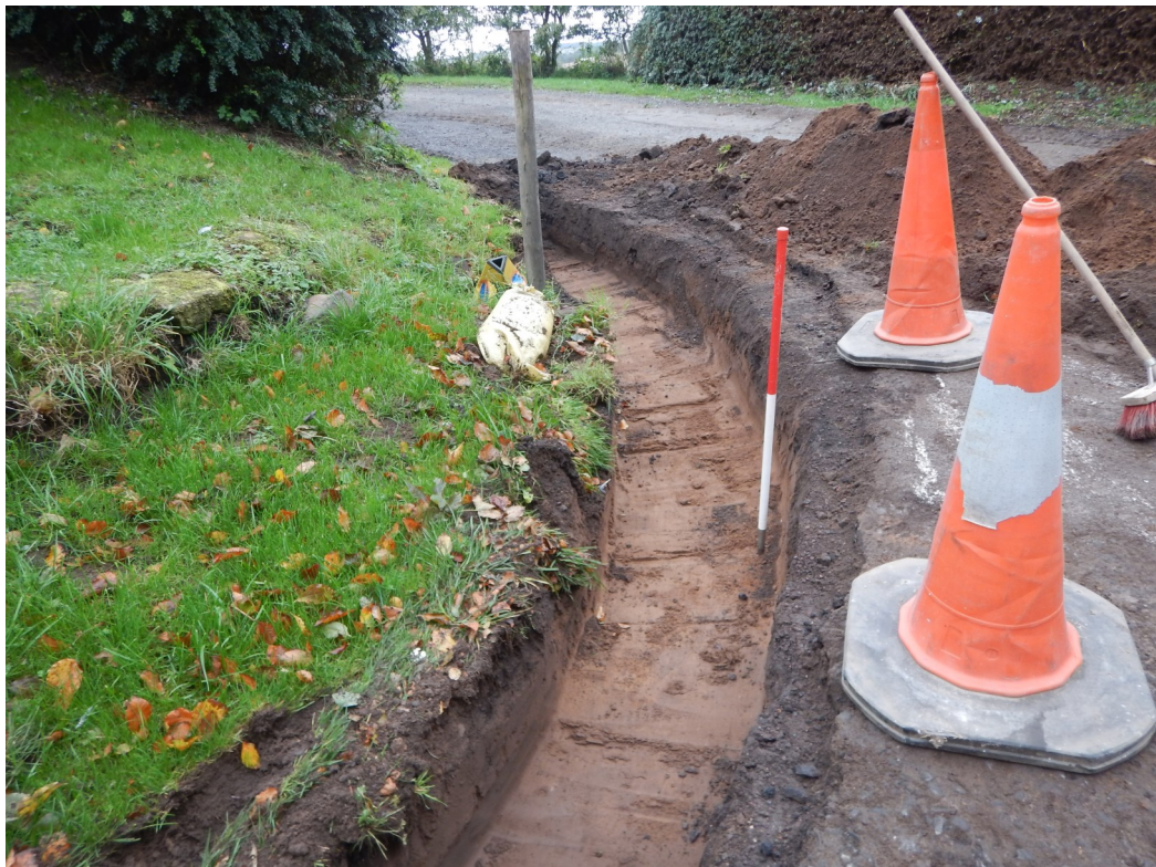
Plate 4 Western trench looking north-west
