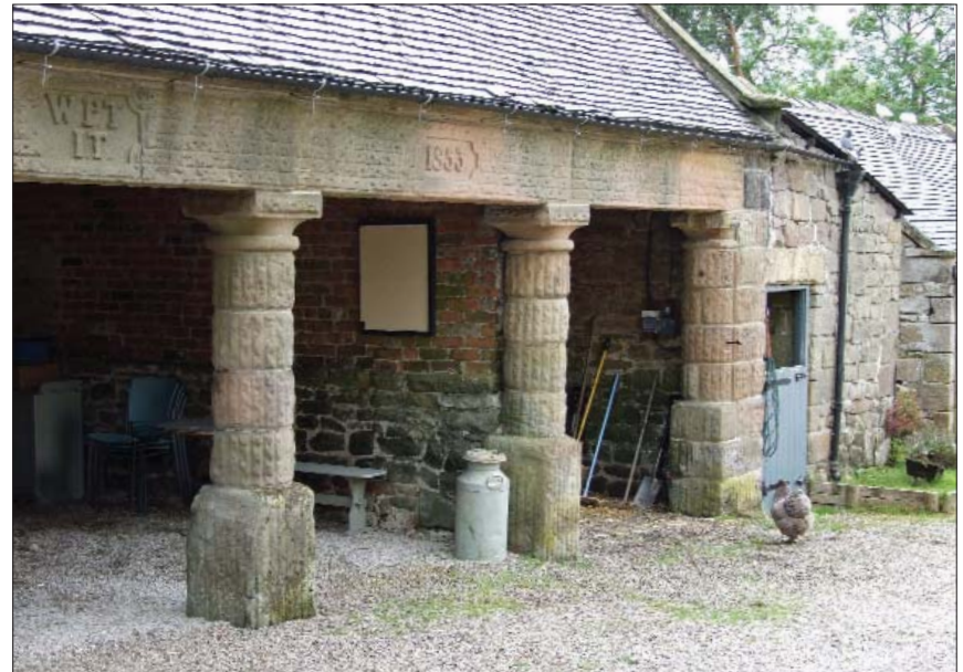
Gratton Grange, near Middleton by Youlgreave, Derbyshire: open-fronted cart shed of coursed granite, constructed in 1853. The shed was provided with four bays separated by rusticated columns that supported stone lintels (photograph: D. Knight)
