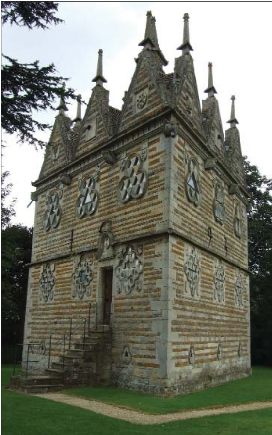
The Triangular Lodge, Rushton. This iconic Northamptonshire building was erected by Sir Thomas Tresham in the 1590s as a two-storey warren lodge. It is imbued with references to the number three, symbolic of the Holy Trinity, and was built in defiance of the prevailing Protestant orthodoxy as a testament to Tresham's strong Catholic faith (photograph: Emily Knight)
