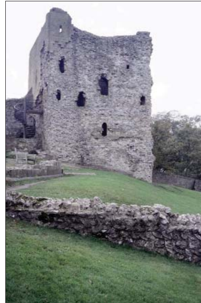
Peveril Castle, Castleton, Derbyshire: late 12th century stone keep (photograph: Richard Sheppard) and aerial view of the castle (NMR20450/18; SK1482/39; 9/11/05; © English Heritage. NMR). The latter shows the location of the keep atop the ridge dividing Cave Dale (above) from the medieval town; Peak Cavern dissects this ridge and separates the eastern stone-walled bailey and keep from the ditch and rampart enclosing the western bailey (right)
