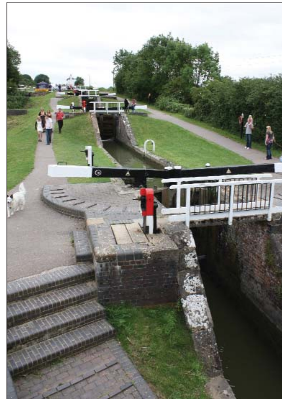
Foxton, Leicestershire: construction of this dramatic flight of two consecutive staircases of locks, each comprising five narrow chambers and separated by a passing pound, was completed in 1812, enabling the Grand Union Canal to ascend some 23m from the Market Harborough level (Palmer and Neaverson 1992, 76–78; photograph: Richard Sheppard)
