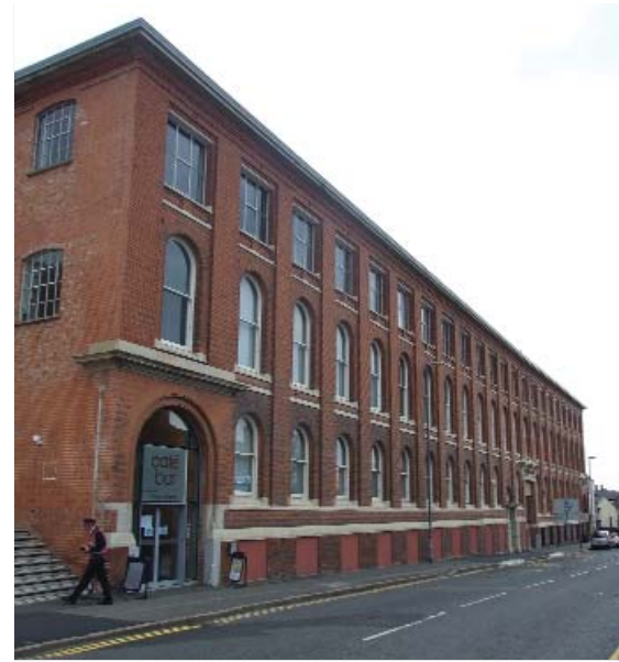
Textile factory in Lower Bond Street, Hinckley, Leicestershire, built mainly between 1877 and 1910 by the hosiery firm of the Atkins. This imposing four-storey building overlooks a row of early framework-knitters' cottages (Objective 9I) and provides a powerful image of the changing scale of the industry (photograph: D. Knight)
