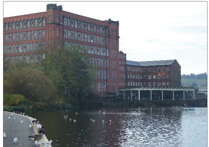
Belper, Derbyshire: the brick-built East Mill with square corner towers, built in 1912, abuts the T-shaped five-storey North Mill, built by William Strutt in 1804 (right). The latter is a very early example of a fire-proofed mill, with cast iron framing and arched brick ceilings (photograph: D. Knight)
