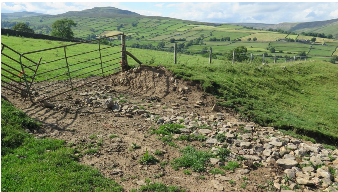
South section across bank SE03639822. IMG_0901 7/7/2015
