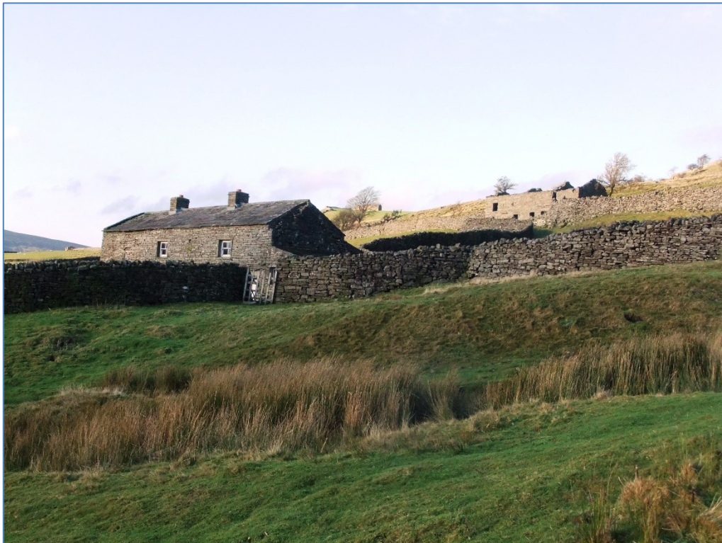
Figure: 55 Heights. Miner-Farmer farms seen from Staneygate. Loaning House which remains occupied in foreground. John Dunn's House in distance and on Figure: 46 below.
