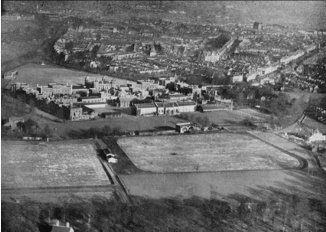
Figure 32: Aerial photograph of the RMA [no date] taken from south, note the blocked casemates (frontispiece to 'The Royal Military Academy', Maj Gen Sir W. Gillman RA DSO, Journal of the Royal Artillery Volume 50, 1924)
