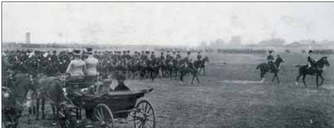
Figure 11: 'H.M. The King's Review at Woolwich, 1913' looking south-west – the Brook Fever Hospital water tower is visible on the horizon. Courtesy of the Royal Artillery Historical Trust AL 100/53
