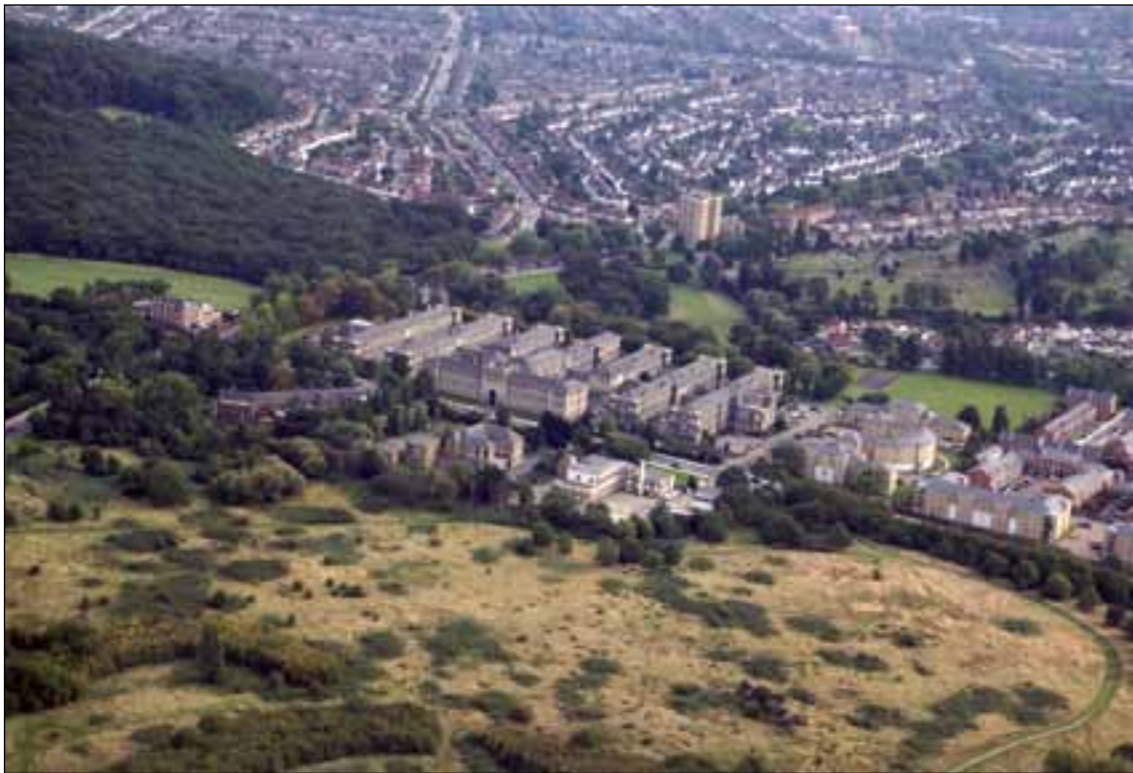
Figure 10: The southern end of Woolwich Common in 2006. The Herbert Hospital is visible at the other side of Shooters Hill Road. To its right is the former site of the Brook Fever Hospital, now redeveloped for housing. NMR TQ4276/36 (24457107) 06-SEP-2006 © English Heritage. NMR
