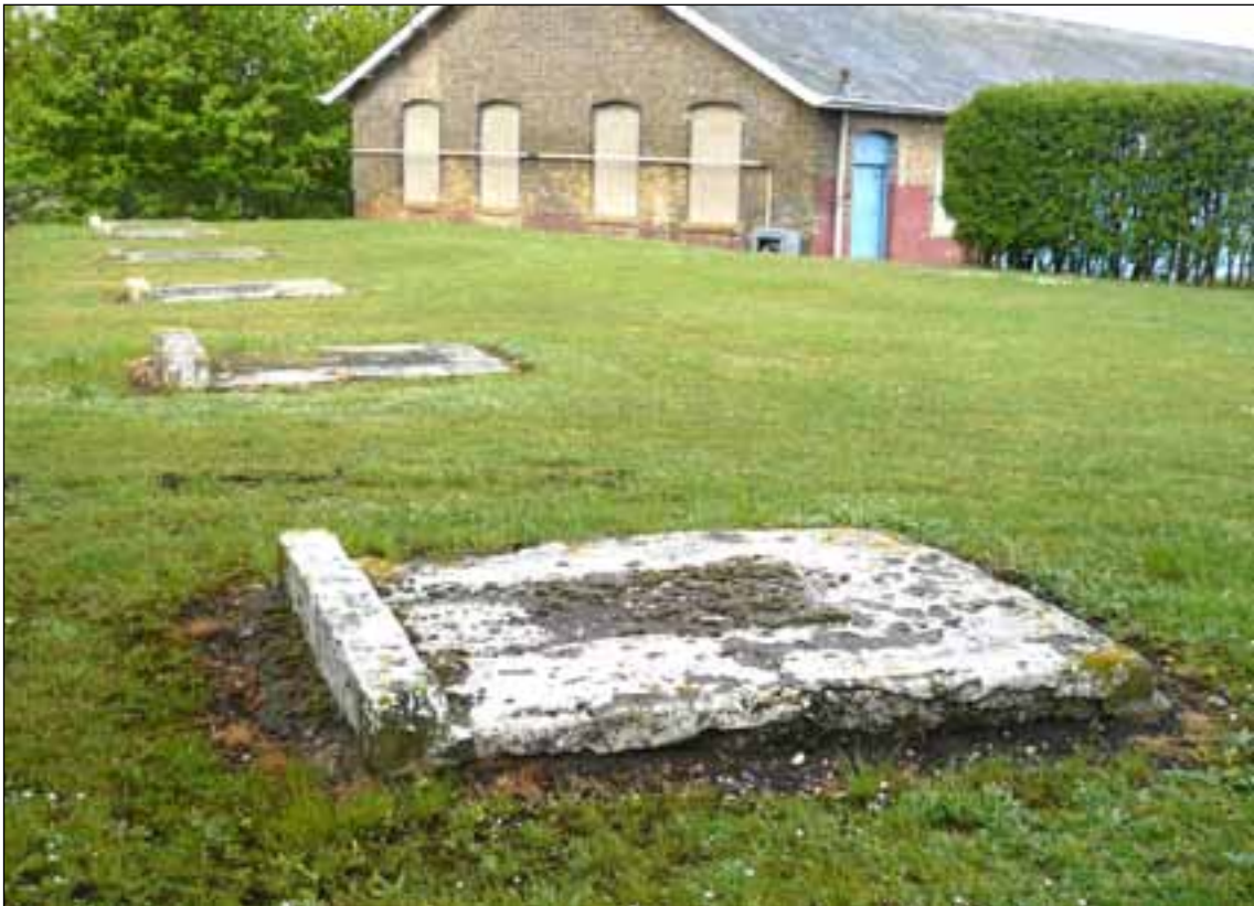
Figure 24: The surviving gun platforms from the ‘Saluting’ battery (Photo: Sarah Newsome)
