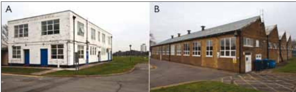
Figure 18: Two surviving buildings which date to the 1934 rebuild of the former SEE/AWRE site. Though its original function is unknown, during the AWRE phase (1957) the building in photograph A (formerly Building B, latterly 10/17) was in use as a surgery, contracts office and drawing office (TNA:PRO ES 11691) . The two most northerly (background) bays of the north-light construction building in photograph B (formerly N, latterly 10/8), are thought to date to 1934, whilst the two southerly (foreground) bays probably date to the 1949/1950 arrival of the AWRE. The SEE used the building as a 'Tank Fitting Shop' and in the AWRE phase it initially housed 60 people involved in coil impregnating, polishing, moulding and winding (P Guillery, pers comm; LMA, GLC/AR/BR/26/WO/M/24/11-2: LBGPA). The main block was extended in the mid-1950s (P Guillery, pers comm; LMA, GLC/AR/BR/26/WO/M/24/11-2: LBGPA) when the building was in use as a machine shop and tool room (TNA:PRO ES 11691). Photographs by Derek Kendall DP093974 / DP093978 © English Heritage
