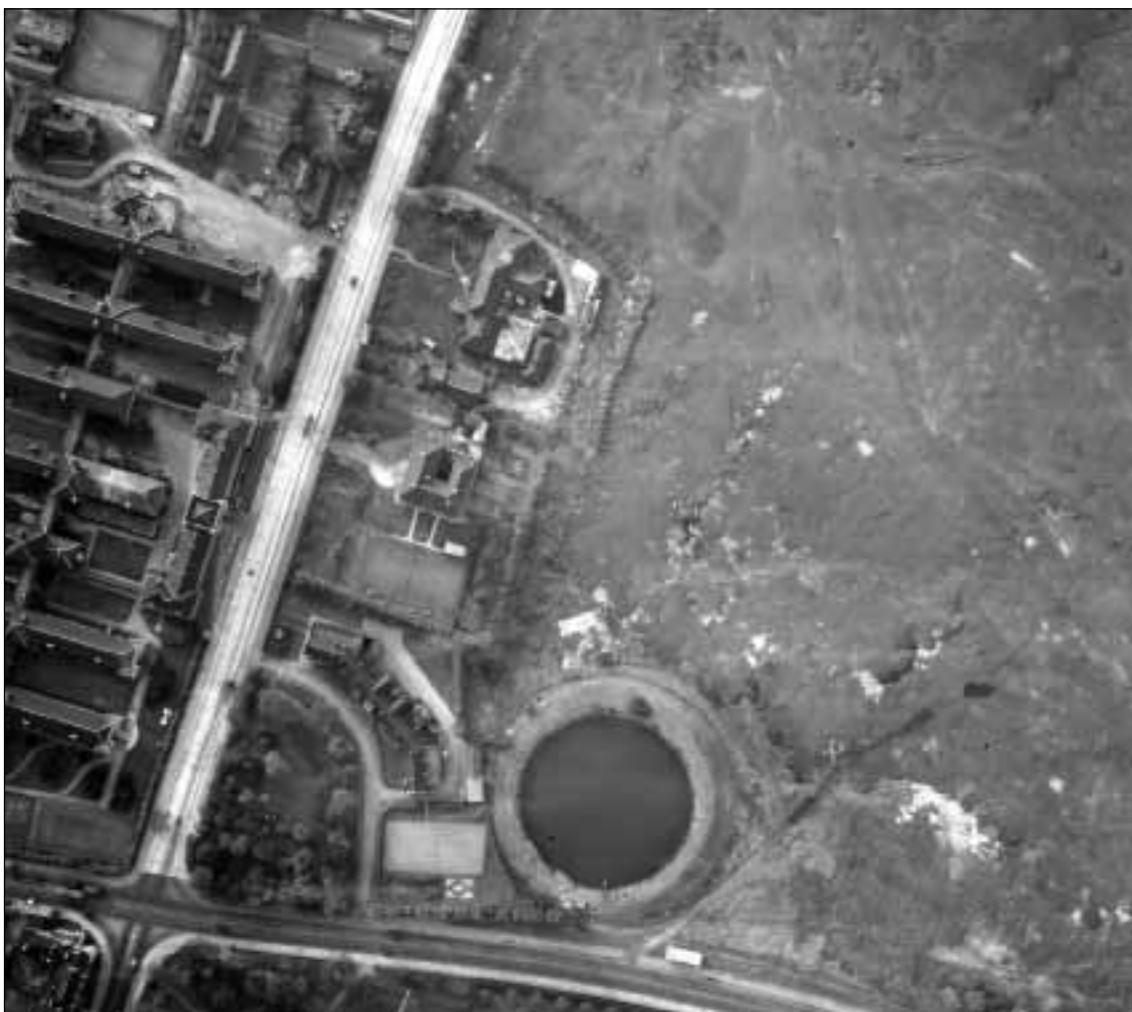
Figure 14: An aerial photograph taken in 1945 showing the south-east corner of the extensive heap of spoil which covered the southern end of Woolwich Common and the circular reservoir built in 1844 (RAF 106G/UK/916 6036 11-OCT-1945) English Heritage (NMR) RAF Photography
