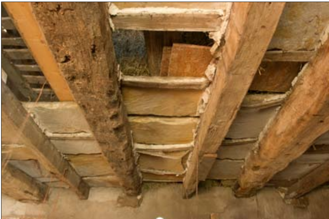
Fig. 21: stone slabs laid over the timber joists of the byre at Annat Walls [DPI09773].
