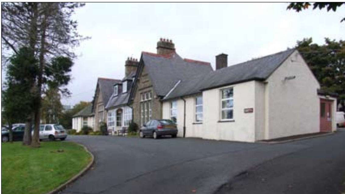
Fig. 78: The Ruth Lancaster James Cottage Hospital, Alston. [DPI35415].
