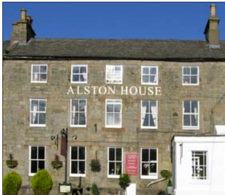
Fig. 11: Rare ashlar masonry on the central part of the mid-18th century Alston House, Townfoot, Alston. [DPI35360]
