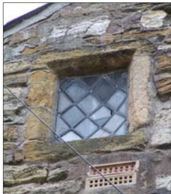
Fig. 29: Small chamfered window in the gable of Church View Cottage, The Butts, Alston. [DPI35369].
