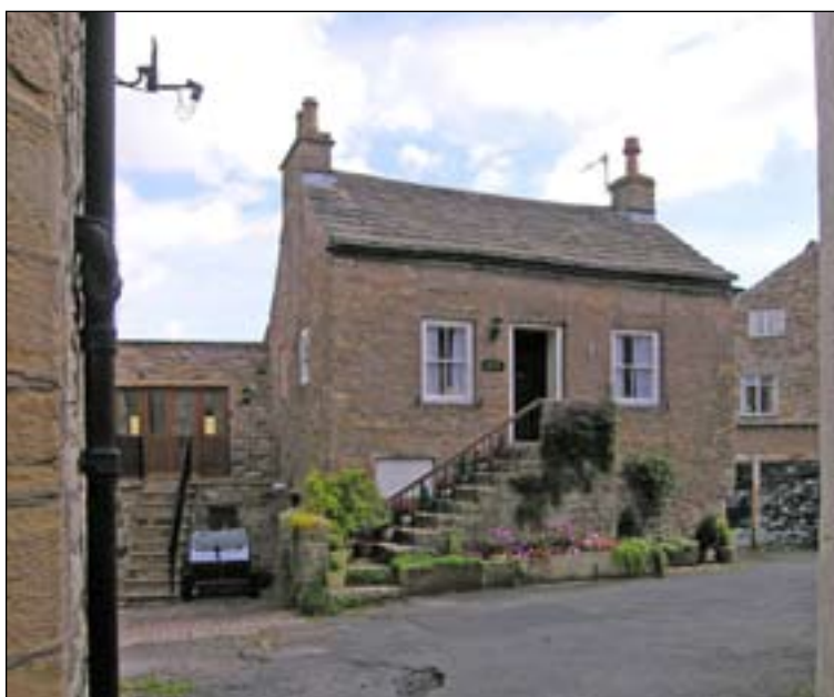
Fig. 119: Jaycott, Back O' the Burn, Alston [DPI35482]
