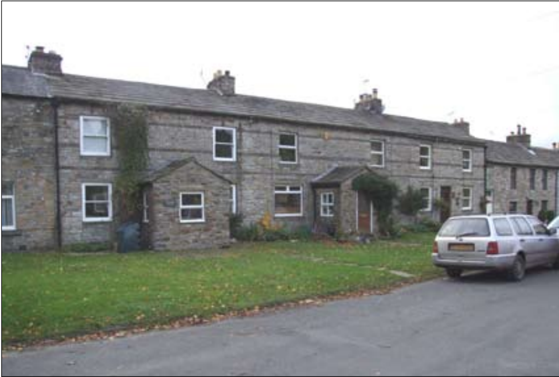
Fig. 60: Tynedale House, Bridge View and neighbour, The Green, Garrigill. [DPI35397].
