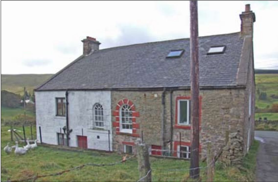
Fig. 65: Chapel House Cottages, the former Primitive Methodist chapel, Whitehall, Nenthead. [DPI35403].
