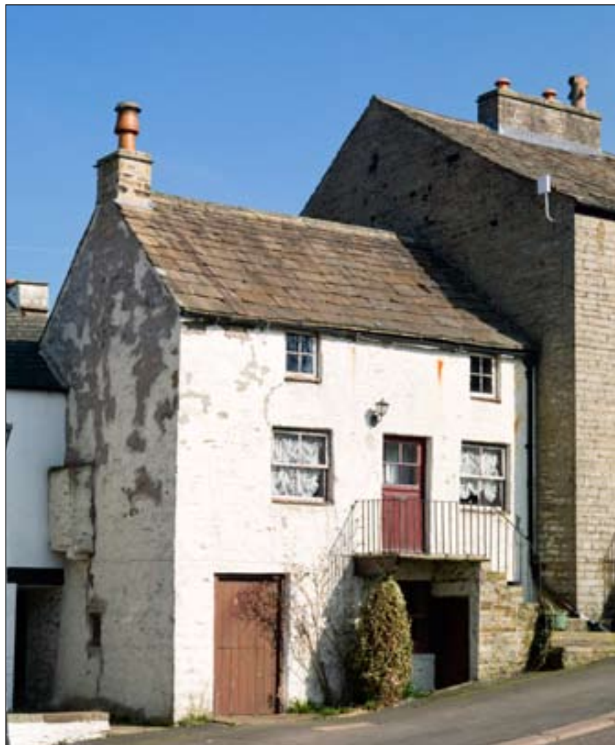
Fig. 30: Later 18th century house with projecting oven on its first floor, western end of Front St, Alston. [DP071459].
