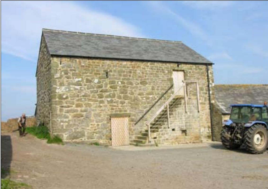
Fig. 18: bastle at The Raw, Hepple, Northumberland. This bastle is much rebuilt, with a later permanent stair and a byre doorway inserted into this elevation. [DPI35346].
