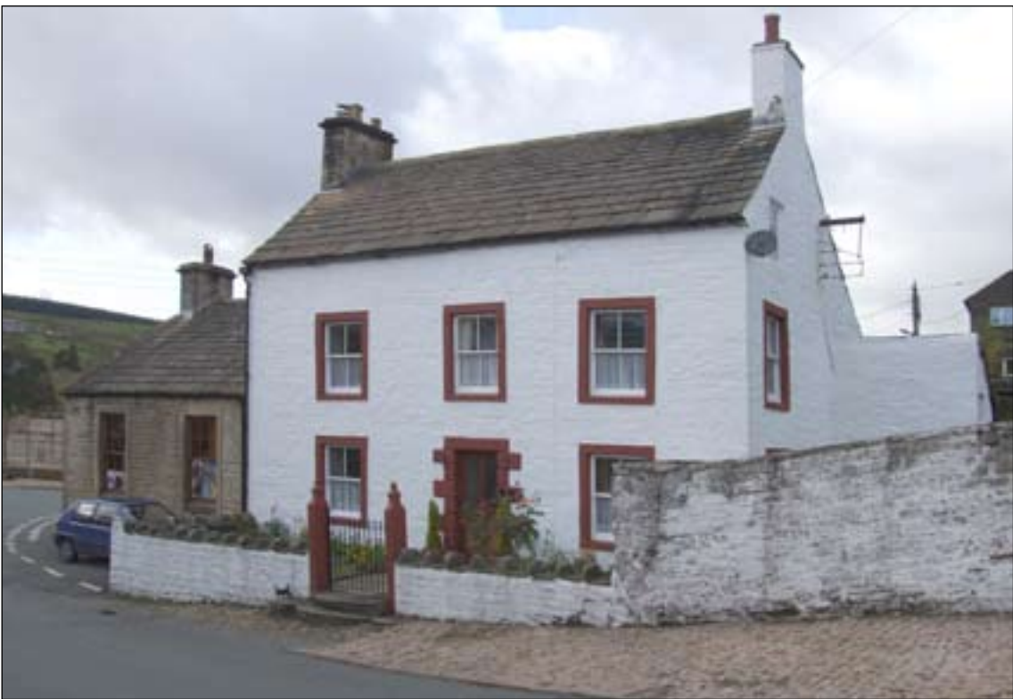
Fig. 45: Ivy House and the attached former Reading Room, now community shop, Nenthead. [DPI35385].
