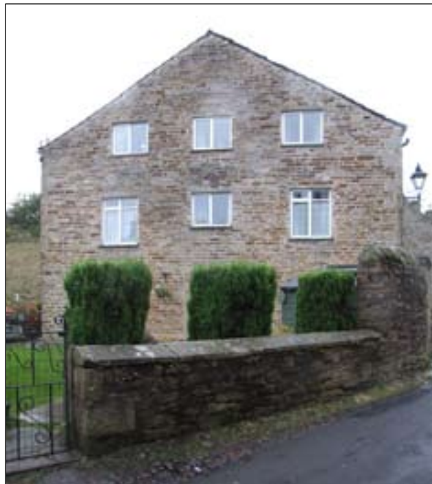
Fig. 51: Former Methodist Chapel, now Chapel House and Holmlea, Back o'the Burn, Alston. [DPI35388].
