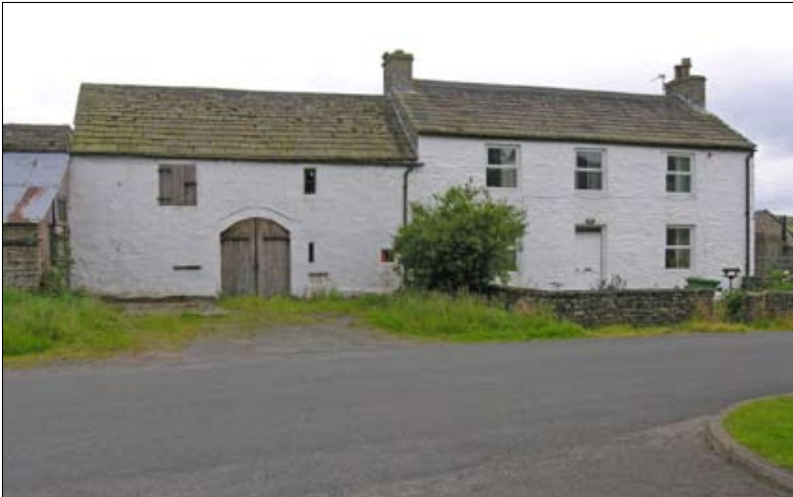
Fig. 104: Gatefoot Farm, Garrigill, showing the earlier phase to the left, now a barn (with ground floor fire window) and the later farmhouse to the right. [DPI35489]
