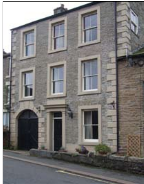
Fig. 63: Albert House, Townhead, Alston. [DPI35399].
