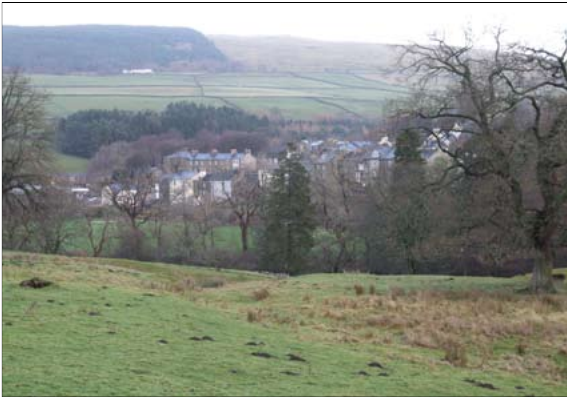
Fig. 100: The view from Raise Bank across the South Tyne to Townfoot. [DPI35474]
