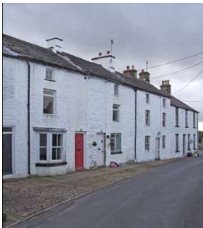
Fig. 46: Houses on the principal street of Overwater, Nenthead. [DPI35386].
