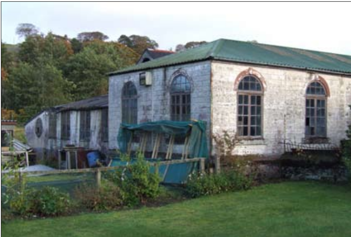
Fig. 112: Motor garage in prefabricated concrete panels, Holmsfoot, Nenthead [DPI35493]
