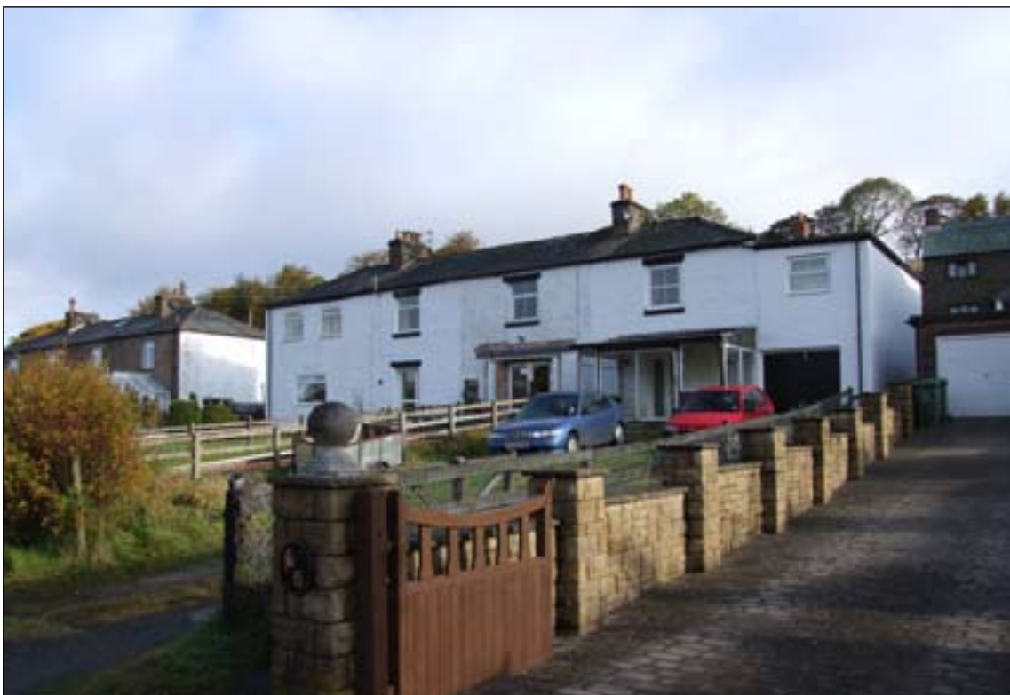
Fig. 59: Groups of 4 terraced houses in Hillersdon Terrace, Nenthead. [DPI35396].
