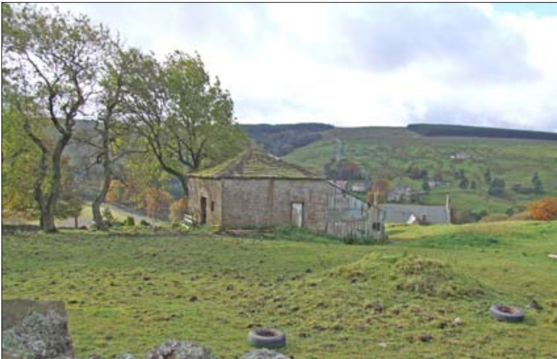
Fig. 110 The Powder House, built by the London Lead Company overlooking the village at some remove from their Nenthead workings [DPI35477].
