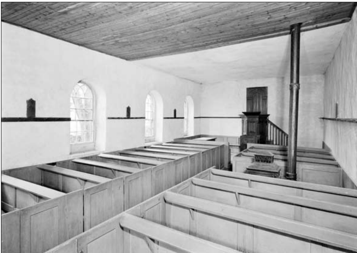
Fig. 50: the interior of Redwing Chapel, taken in 1977. [BB77/03397].
