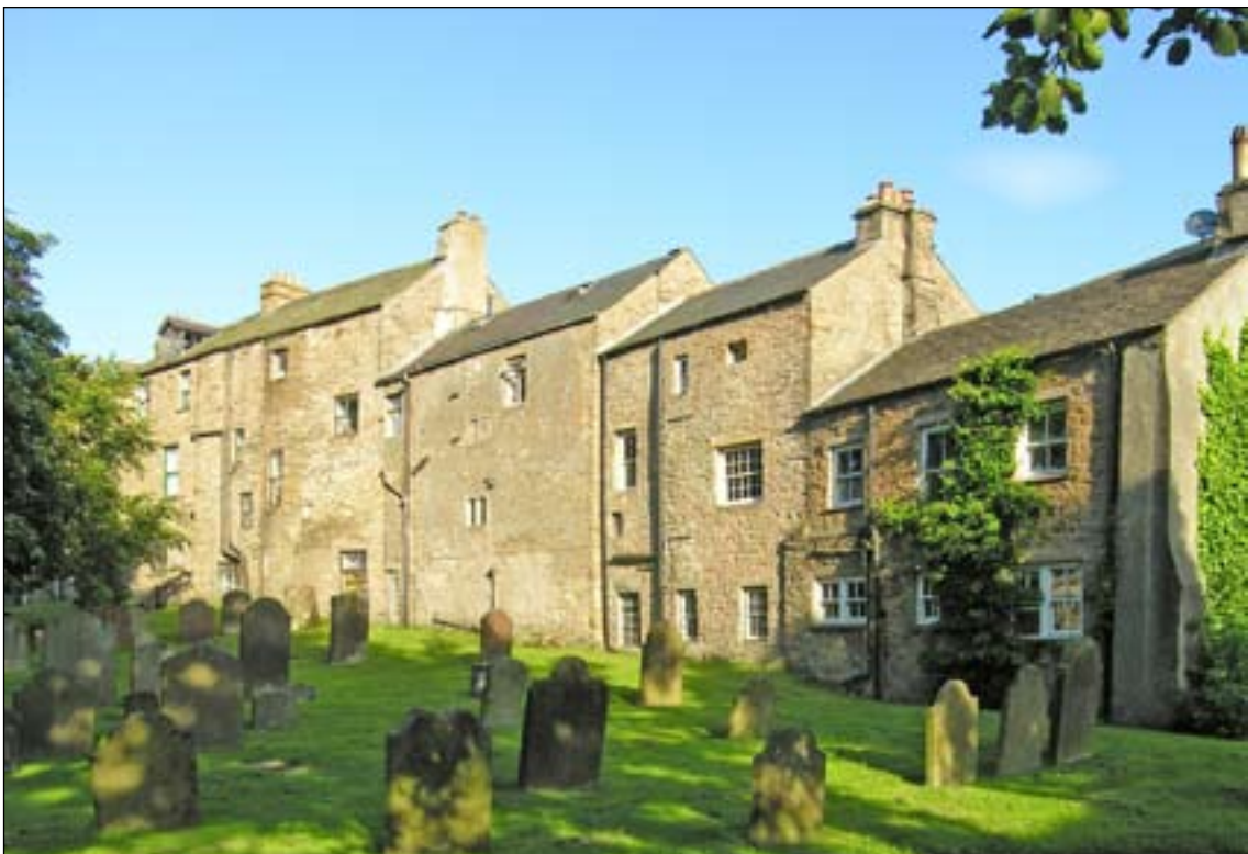
Fig. 26: Houses on Front St, Alston, seen from the rear. They are single-pile, built up against the boundary of the churchyard, and date from c. 1700. The former library, now unoccupied, is the 2nd from the left; Pennine Ways is 2nd from the right. [DPI35367].
