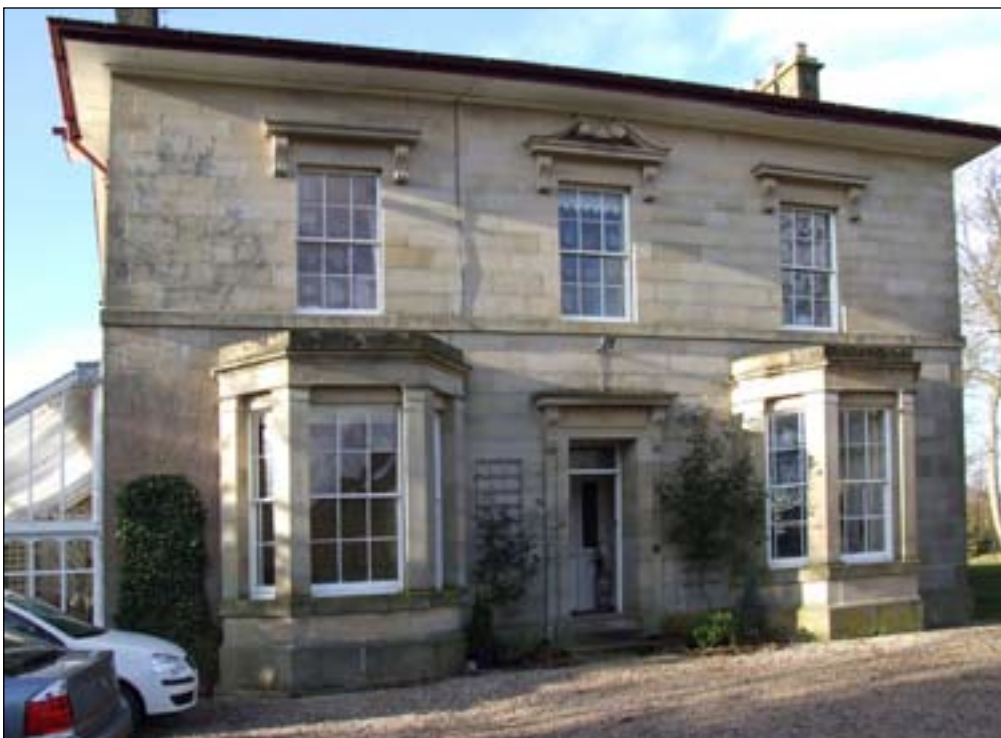
Fig. 64: Harbut Lodge, with the ashlar masonry so rare in the parish. [DPI35401].
