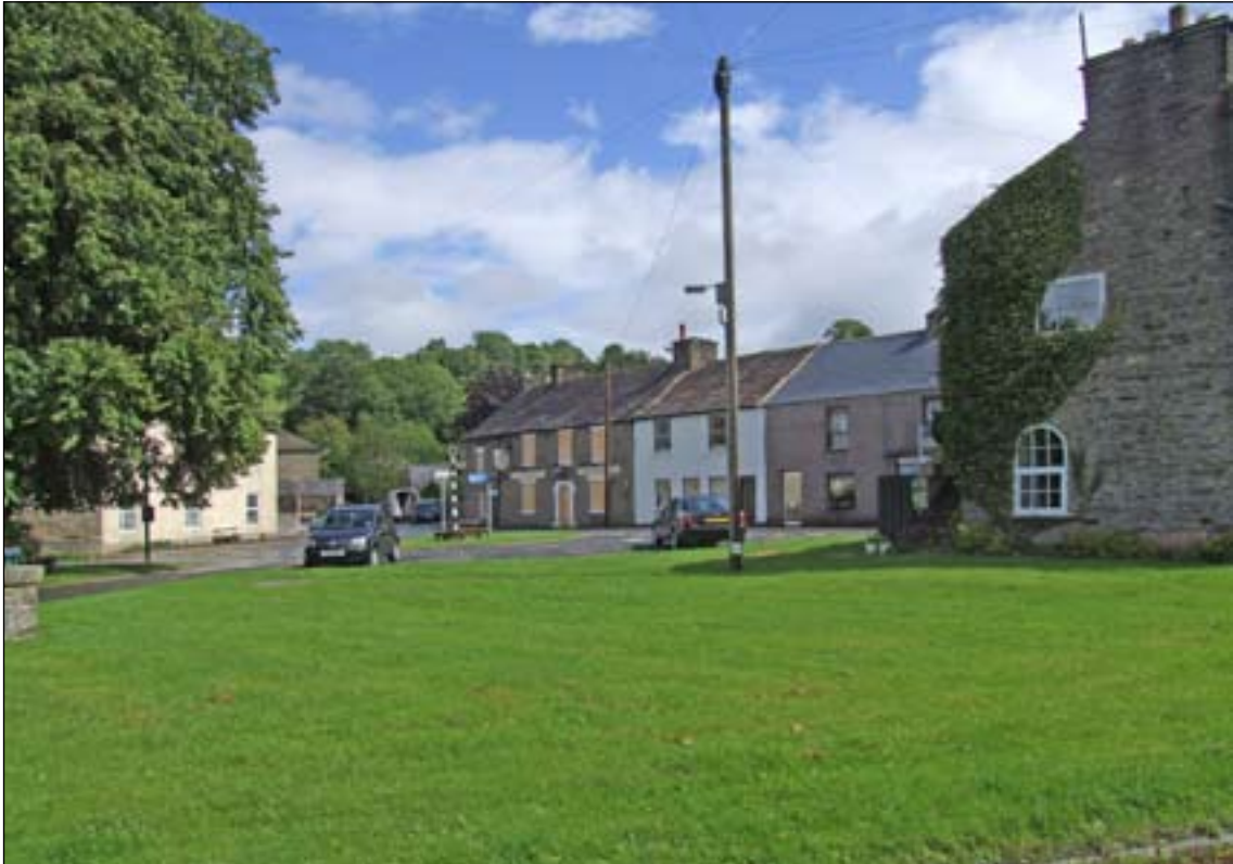
Fig. 102: The Green at Garrigill with the former smithy to the right and the George and Dragon shown with its windows boarded. [DPI35475].
