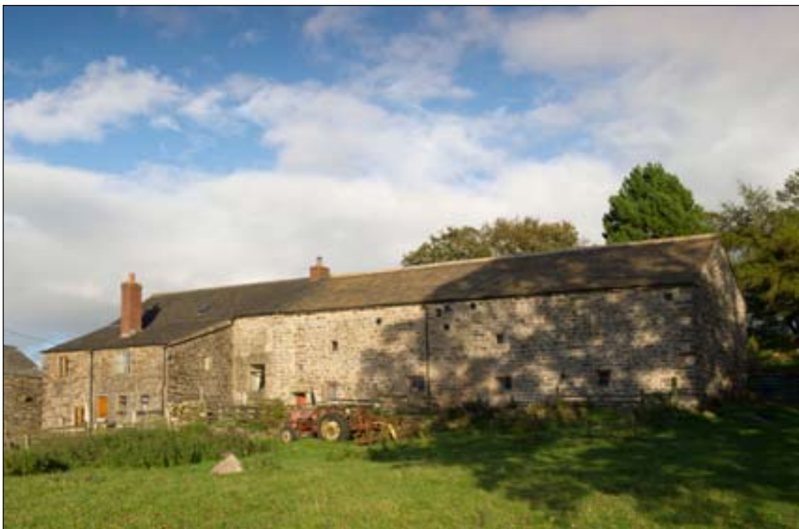
Fig. 116: Annat Walls [DPI09762]
