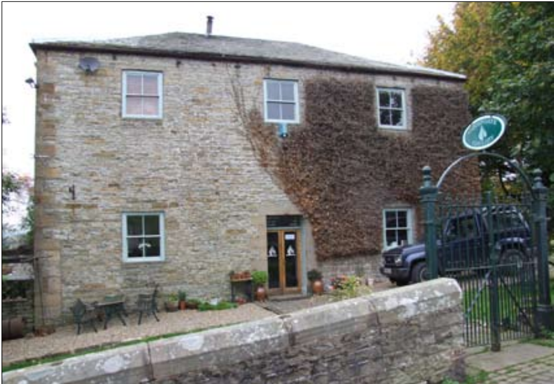
Fig. 52: The former Independent chapel, Gossipgate, Alston. It was converted to a house in the 1970s. [DPI35389].
