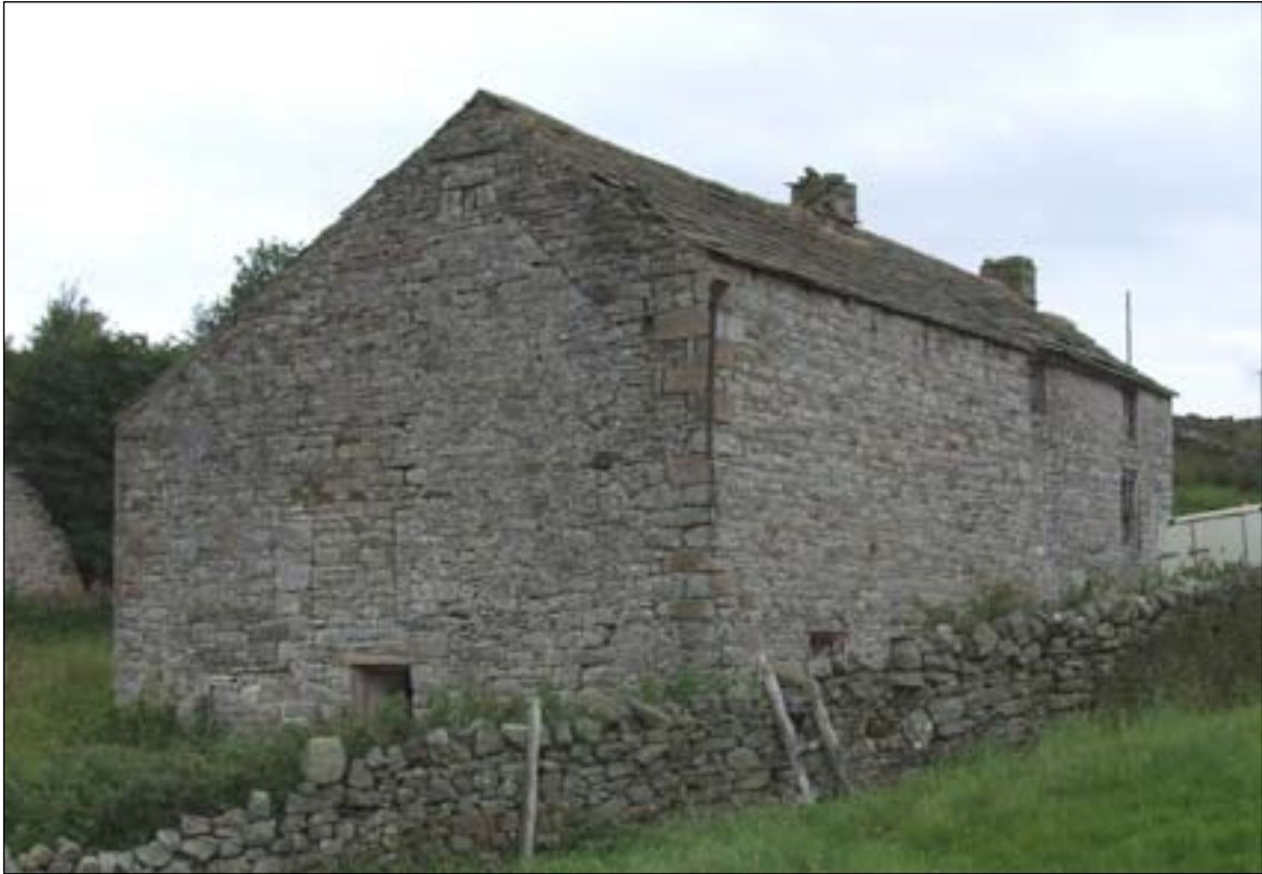
Fig. 23: the pair of bastles near Annat Walls, from the SW. That in the foreground is older than that beyond, which is dated 1707. Both were originally one and a half storeys high, with a steeper-pitched roof and each had a smoke hood. [DPI35363].
