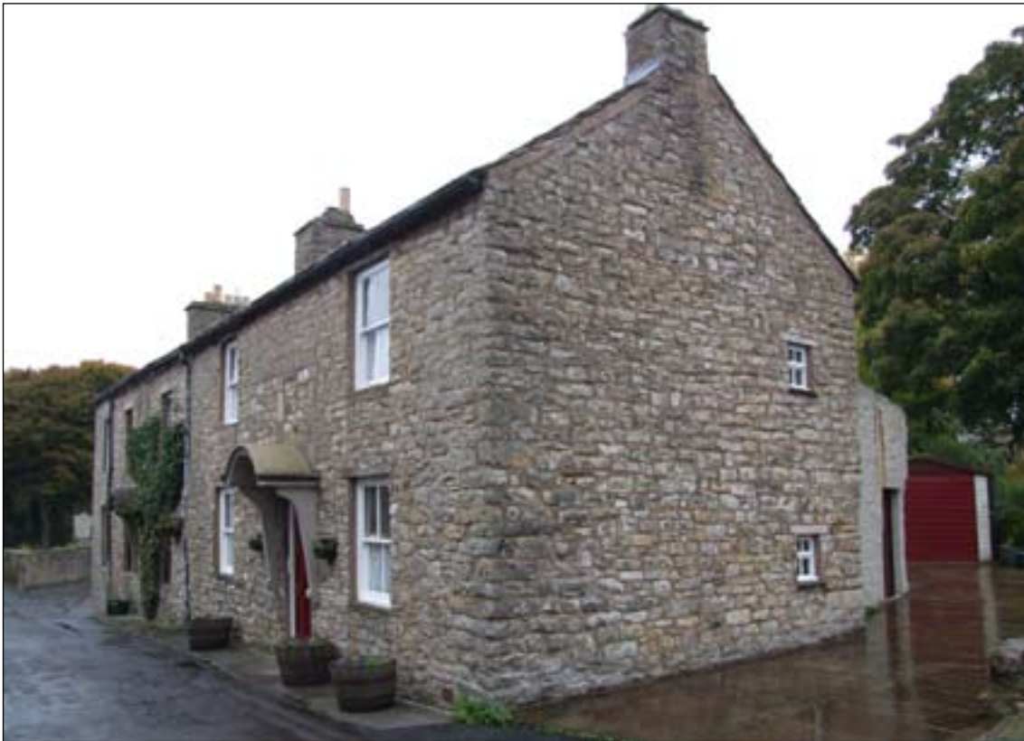
Fig. 93: Houses in King's Arms Lane, Alston, with concrete canopies added to a much-altered 18th century structure with former first-floor entry. [DPI35483]
