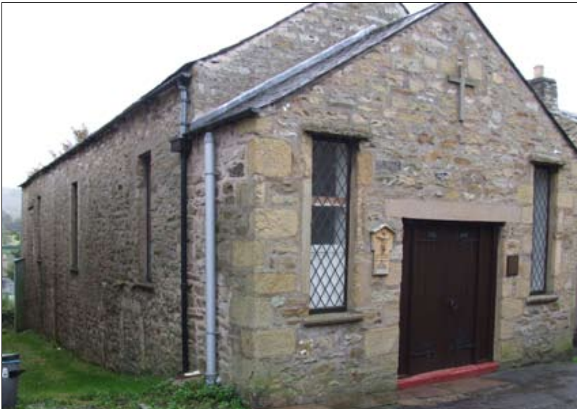
Fig. 94: St Wulstan's Catholic Church, King's Arms Lane, Alston. [DPI35485]
