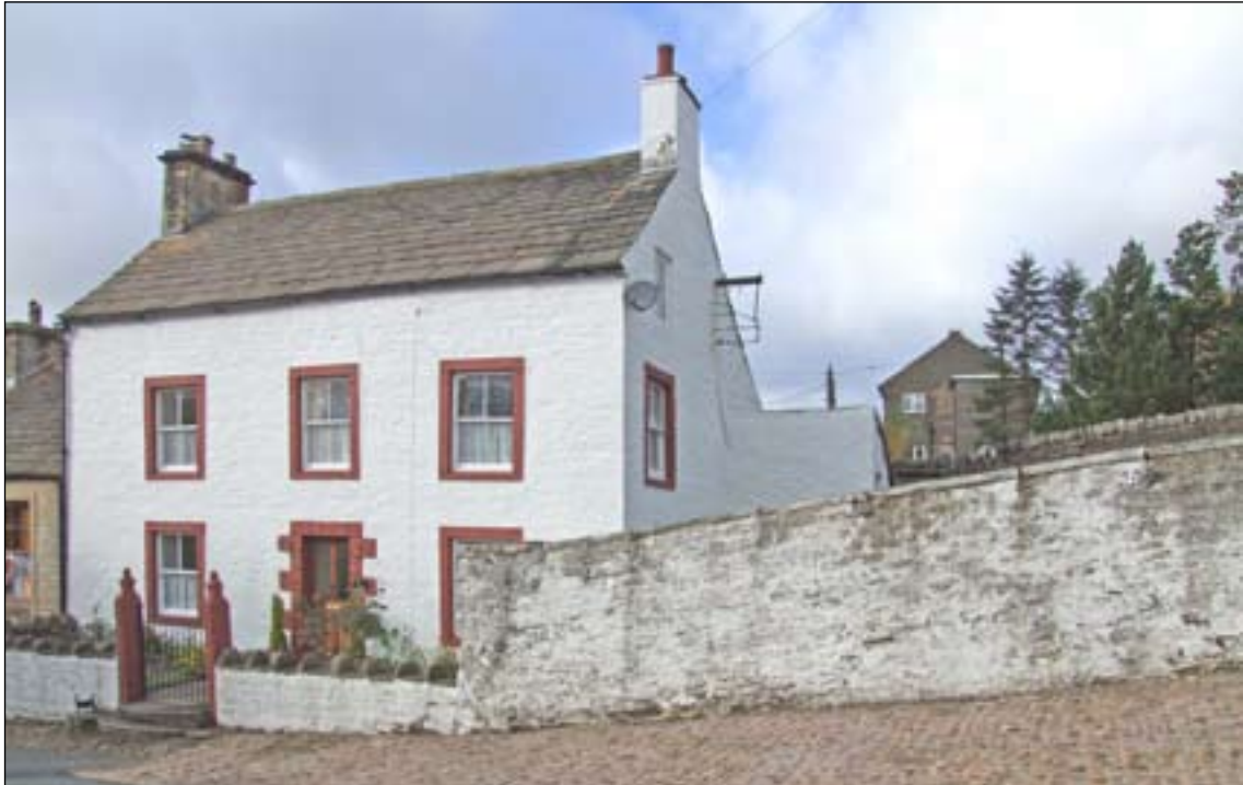
Fig. 13: Coursed rubble disguised by white paint on the mid-18th century Ivy House, Church Lane, Nenthead. [DPI35361]
